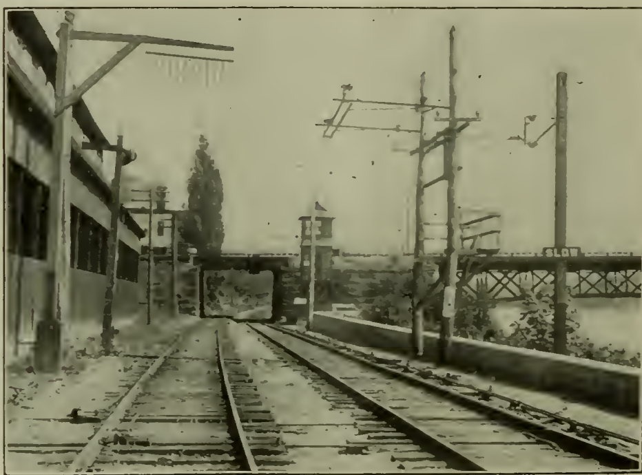
OVERHEAD CONSTRUCTION AT CLARISSA STREET BRIDGE, ROCHESTER—SHOWING TROLLEY SECTION INSULATOR AND BRIDGE WIRING.
