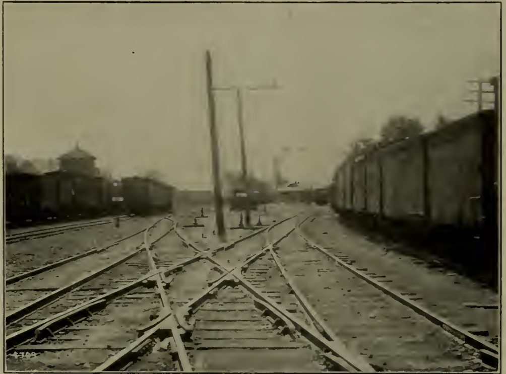
AVON YARD—LOOKING SOUTH TOWARD STATION.
