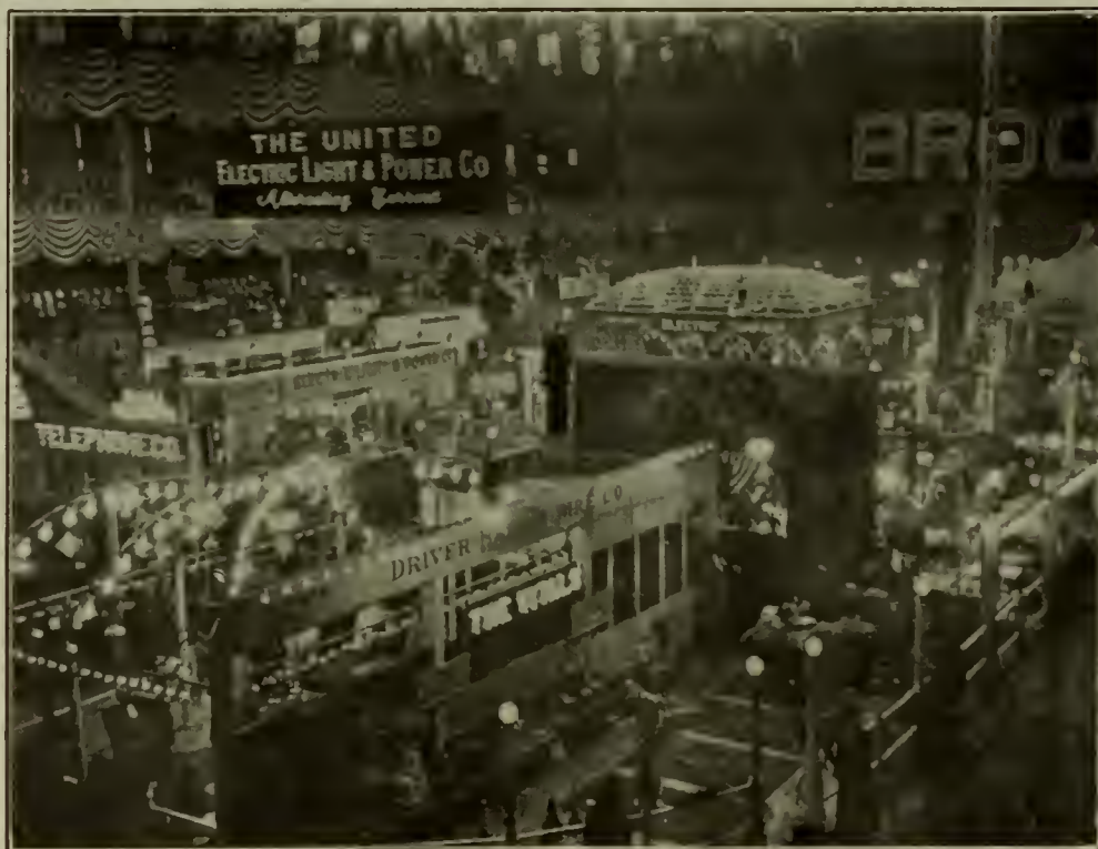
GENERAL VIEW OF SHOW FROM MADISON AVENUE END OF BUILDING.
