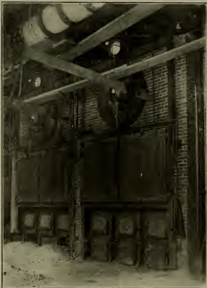
TWO OF THE BOILERS.
