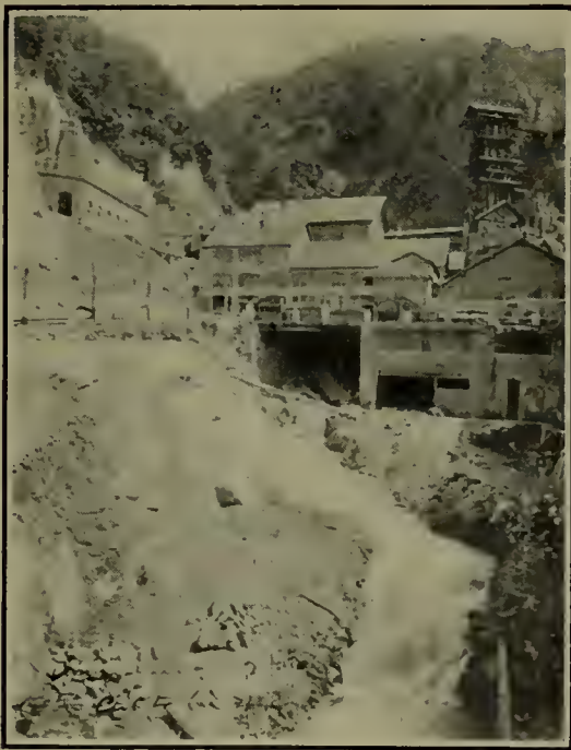
THE POWER PLANT.
