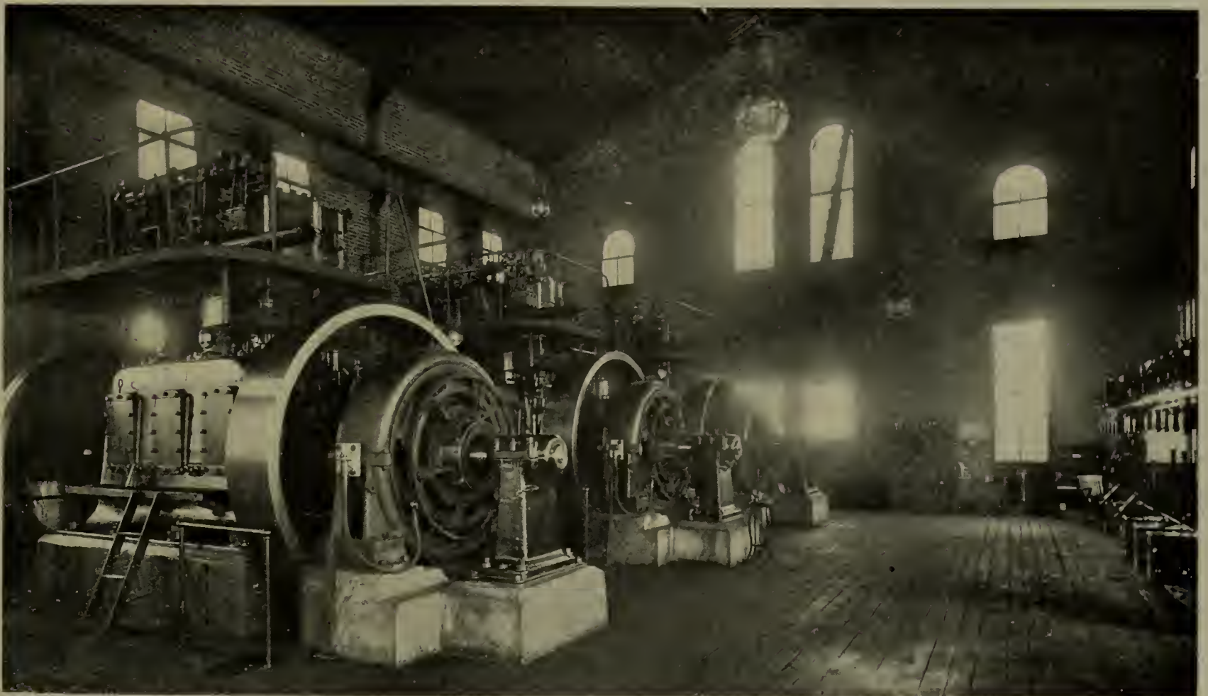
FIG. 1—INTERIOR OF THE GAS POWER STATION OF THE GOULD STORAGE BATTERY COMPANY AND THE GOULD COUPLER COMPANY, AT DEPEW, N. Y. DIRECT CURRENT AT 250 VOLTS IS GENERATED FOR DISTRIBUTION THROUGHOUT THE WORKS BY THREE 150-KW. GAS-ENGINE UNITS
