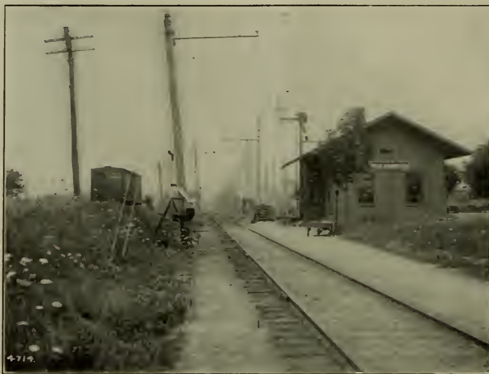
OVERHEAD BRACKET CONSTRUCTION—MAIN LINE AND SIDING AT WEST HENRIETTA STATION.
