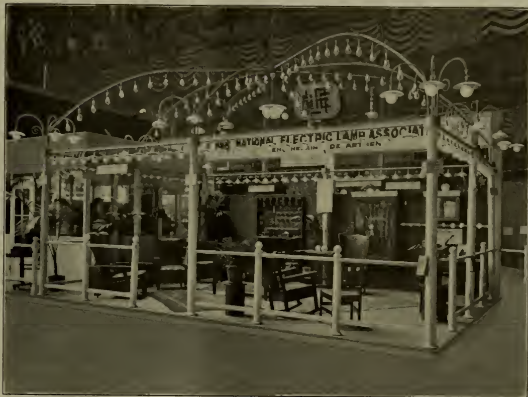
EXHIBIT OF THE NATIONAL ELECTRIC LAMP ASSOCIATION.
