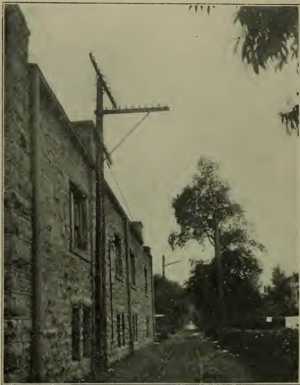
FIG. 1.—SHOWING TELEPHONE AND LIGHTING SERVICE CROSSING THE MAINS OF ANOTHER COMPANY.
