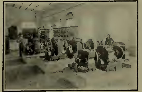
INTERIOR OF PLANT.
