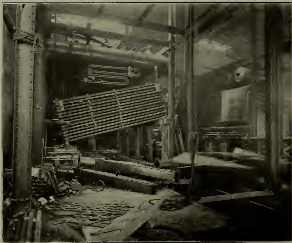
BOILER-ROOM—SIXTEEN BABCOCK-WILCOX BOILERS. 175 LBS. PRESSURE, 150° F. SUPERHEAT
