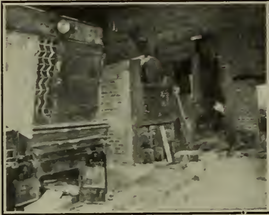
FIG. 2.—INTERIOR OF THE BOILER HOUSE.
