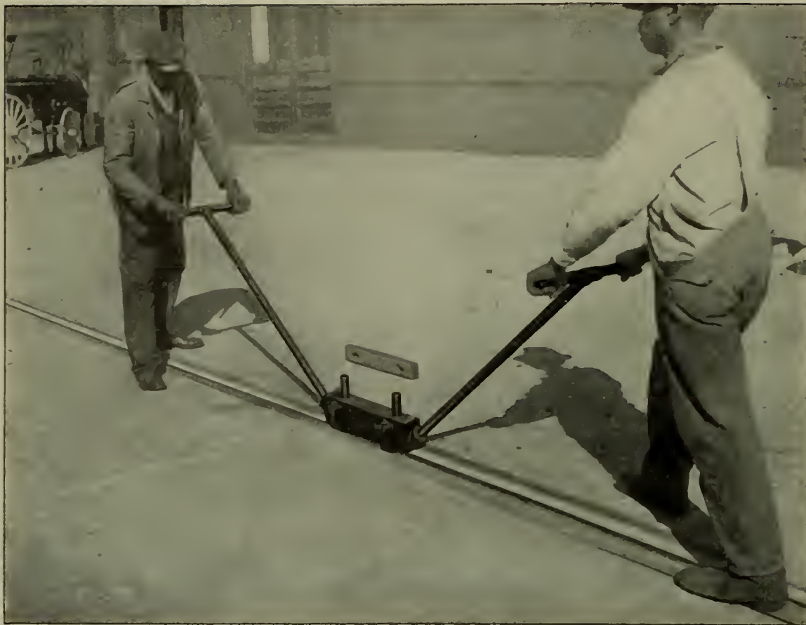
FILING OFF CORRUGATIONS IN A STREET-CAR RAIL
