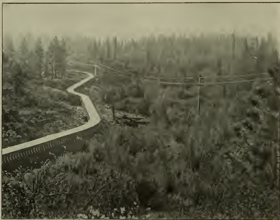
FIG. 8.—PART OF THE FLUME CONNECTING CASCADE RESERVOIR WITH THE FOREBAY. A PART OF THE TRANSMISSION LINE IS ALSO SHOWN
