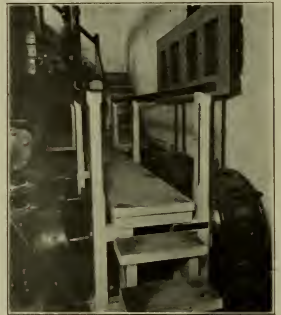
INDUCTION MOTOR DRIVING PUMP.
