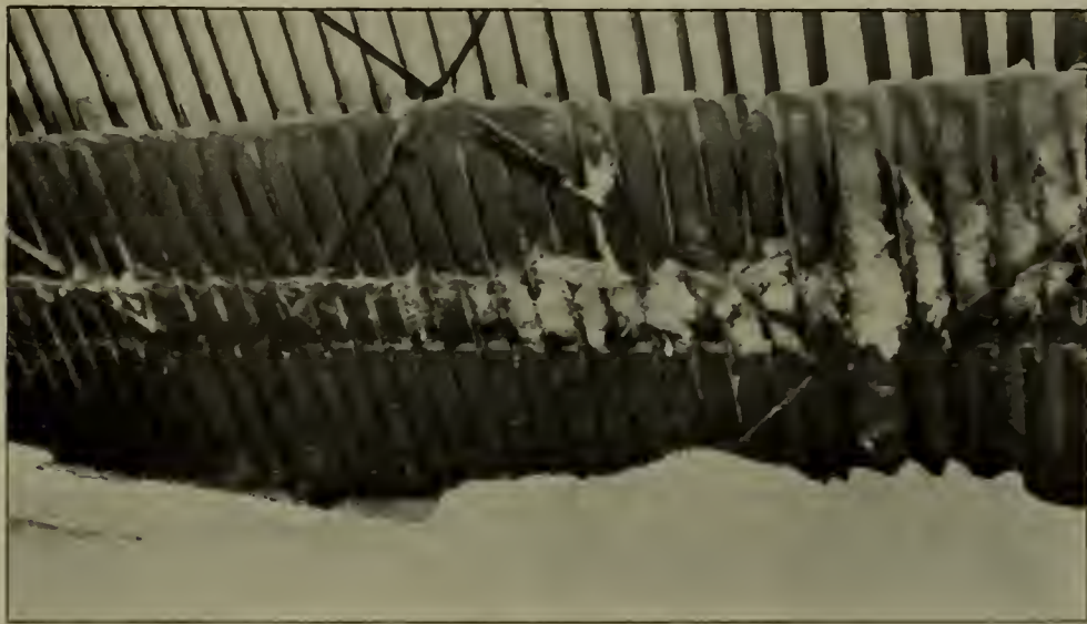
FIG. 7.—A VIEW OF THE UNDER SIDE OF RACKING AFTER THE WATER HAD LOWERED A FEW FEET IN THE FOREBAY. NOTE THAT THE OPENINGS ARE ENTIRELY CLOSED BY ICE SHUTTING OFF THE FLOW OF WATER
