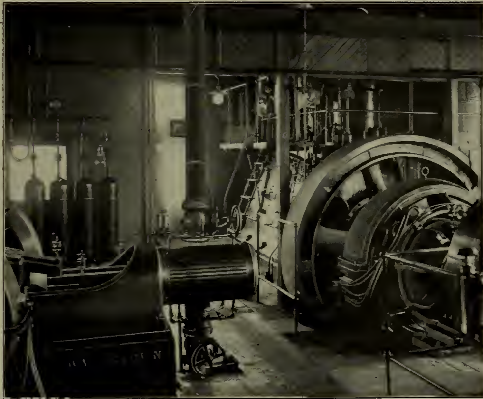
225-HORSE-POWER DIESEL OIL ENGINE DIRECT-CONNECTED TO 165-K. W. FORT WAYNE GENERATOR
