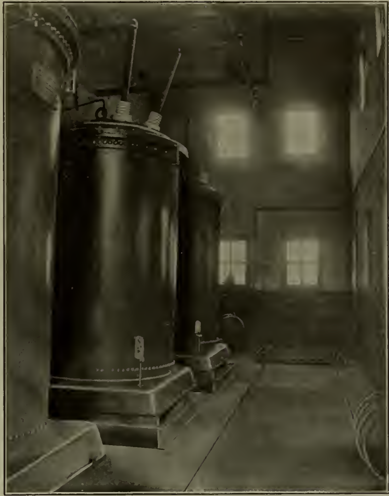
MAIN TRANSFORMER ROOM IN SUBSTATION.
