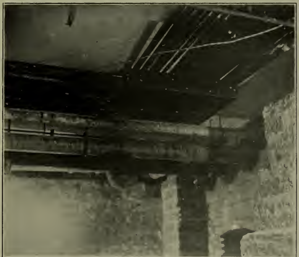
ONE OF SEVERAL LARGE PULL BOXES ON THE CEILING OF THE BASEMENT.
