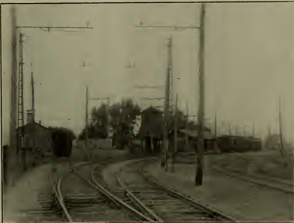
OVERHEAD CONSTRUCTION—MT. MORRIS TERMINAL.
