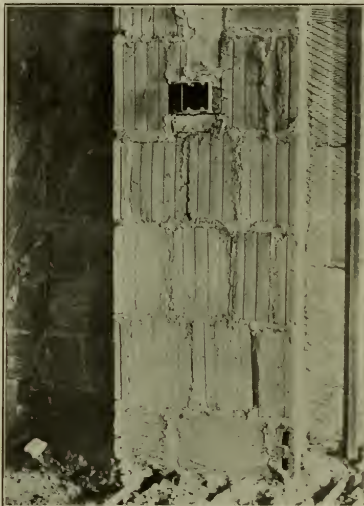
SWITCH BOX—WALL READY FOR PLASTERING.
