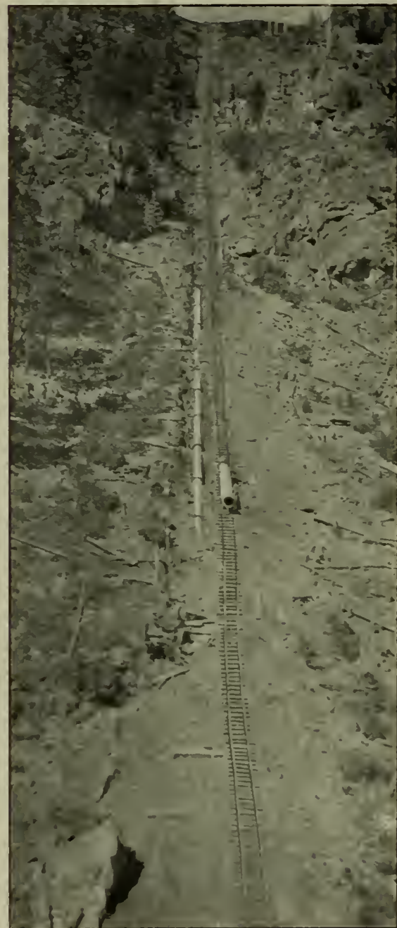
FIG. 6.—A PART OF THE PIPE LINE, SHOWING THE TEMPORARY TRACK FOR HAULING THE PIPE UP THE BLUFF FROM THE POWER HOUSE
