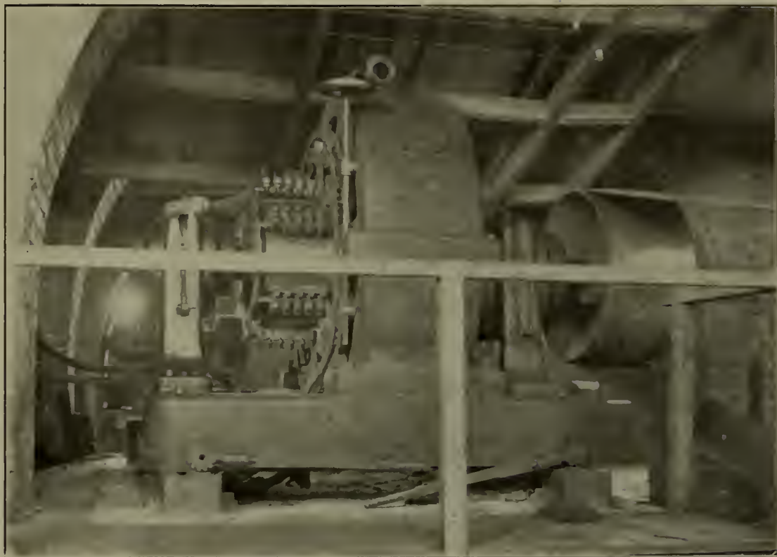
A 100 HORSE-POWER VARIABLE-SPEED MOTOR OPERATING VARIABLE-SPEED PART OF A PAPER MACHINE.
