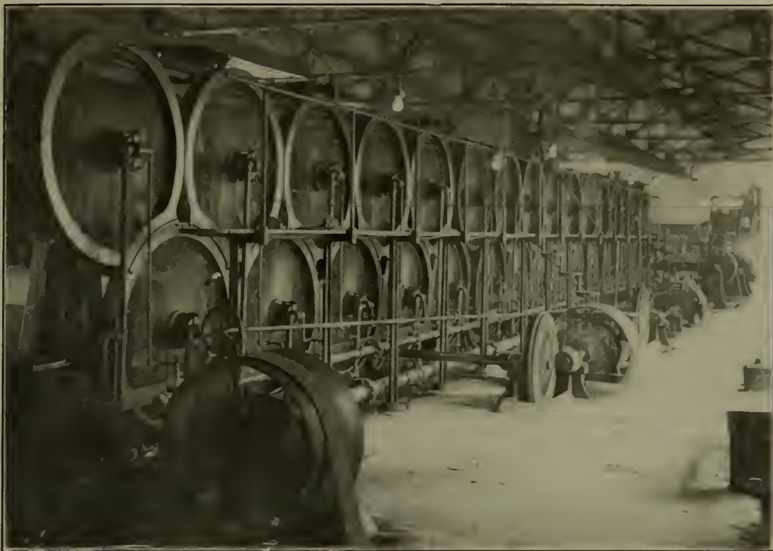
BACK VIEW OF PAPER MACHINE SHOWING METHOD OF DRIVING FROM BENEATH THE FLOOR.
