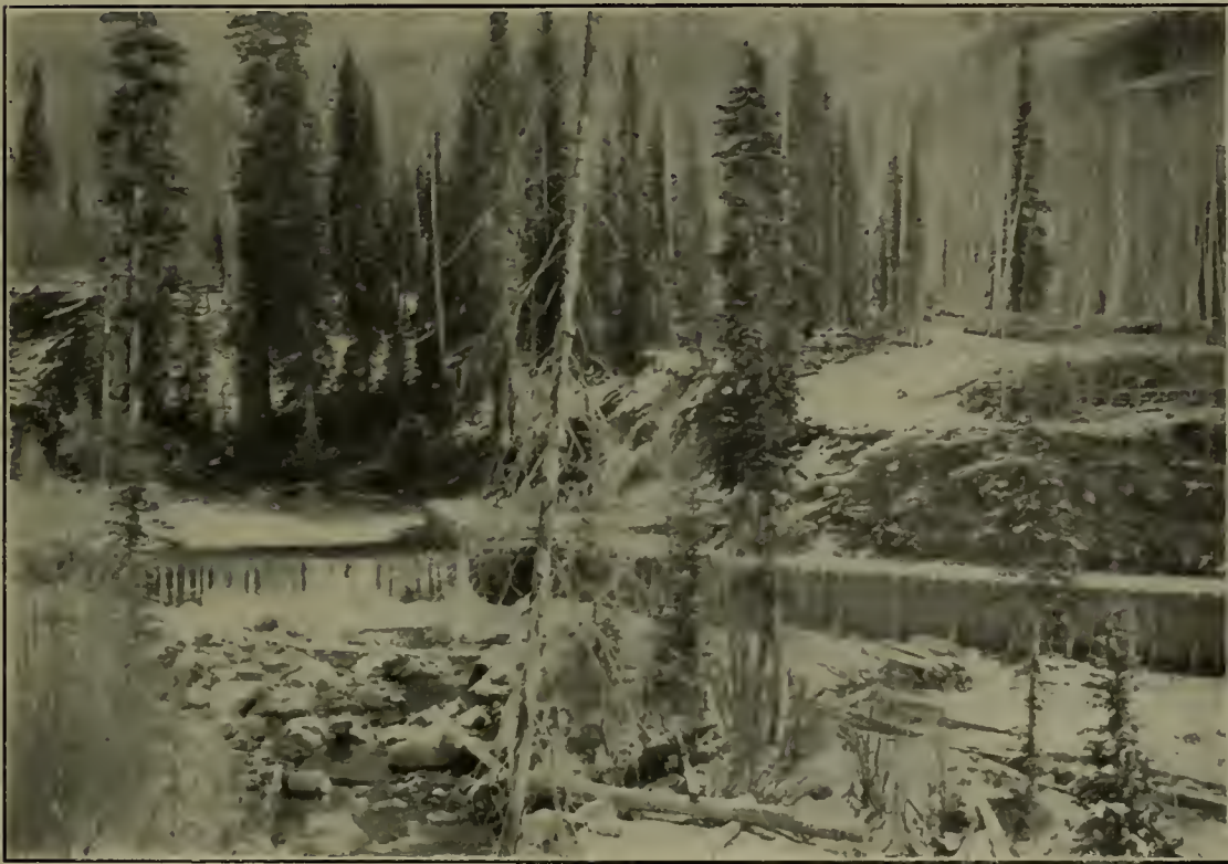
FIG. 1.—THE DIVERTING DAM AND HEADGATE AT CASCADE CREEK, A TRIBUTARY OF THE ANIMAS RIVER IN COLORADO. THE PRESENT 6000-H. P. DEVELOPMENT OF THE ANIMAS POWER & WATER COMPANY UTILIZES ONLY THE WATERS OF THIS CREEK
