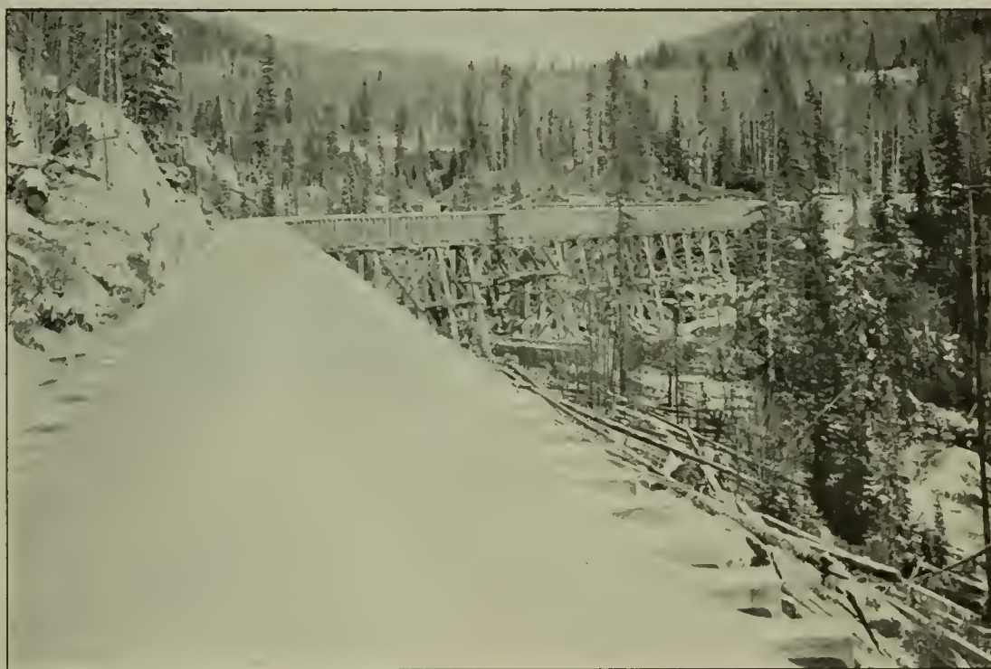
FIG. 9.—A PART OF CASCADE FLUME EXTENDING FROM THE DIVERTING DAM TO THE STORAGE RESERVOIR
