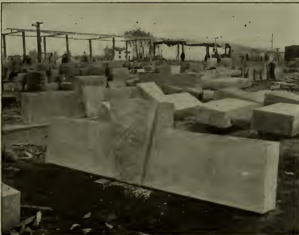
WINDOW LINTELS FOR POWER STATION
