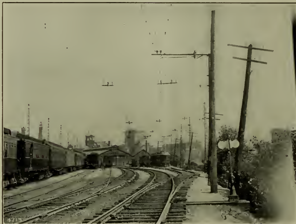
ROCHESTER TERMINAL YARD—OVERHEAD CONSTRUCTION—FOUR ELECTRIFIED TRACKS.
