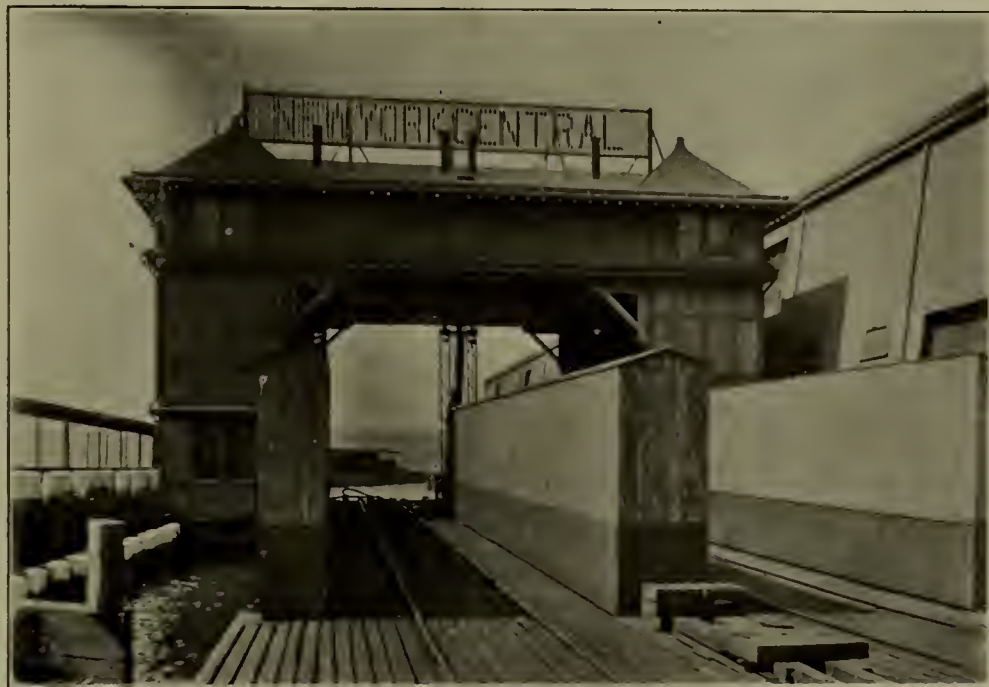
TRANSFER BRIDGE—LAND END.
