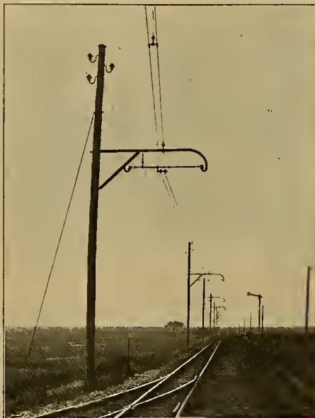
FIG. 1. SINGLE-TRACK LINE CONSTRUCTION
