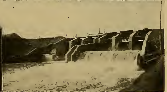
Fig. 2. Croton Dam Power Plant, Head of the 110,000-volt Transmission Line
