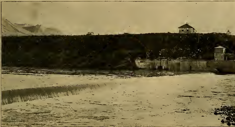
DIVERSION DAM AND POWER-CANAL INTAKE ON SALT RIVER ABOVE ROOSEVELT RESERVOIR
