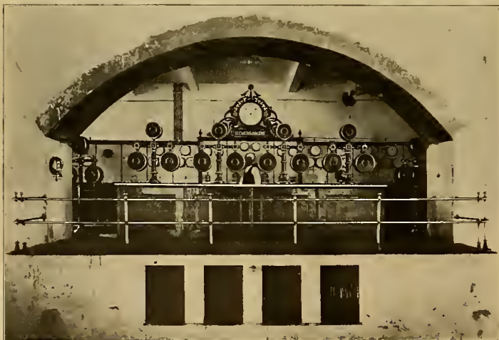
Fig. 6. Main Switchboard at Leizaran Generating Station
