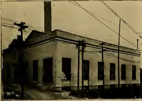
FIG. 5. EXTERIOR VIEW OF CENTRAL STATION AT GRAND FORKS, N. D.
