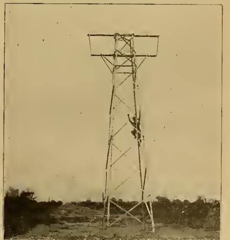
STEEL TOWERS FOR TRANSMISSION LINE FROM ROOSEVELT POWER HOUSE
