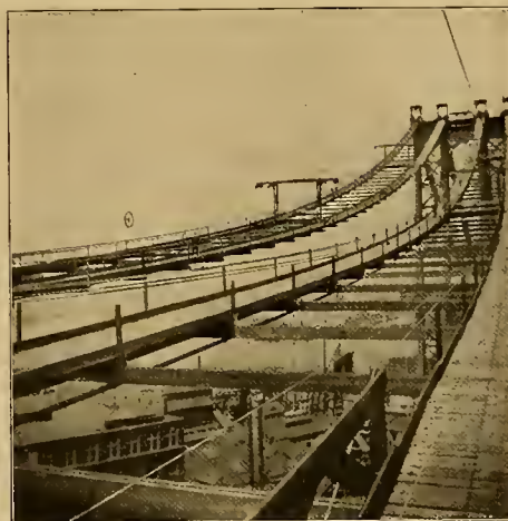
View from Top of Anchorage
