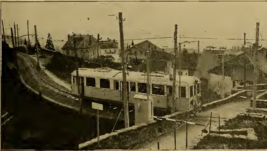
FIG. 1. AUTOMATIC ELECTRIC CROSSING GATE IN SWITZERLAND
