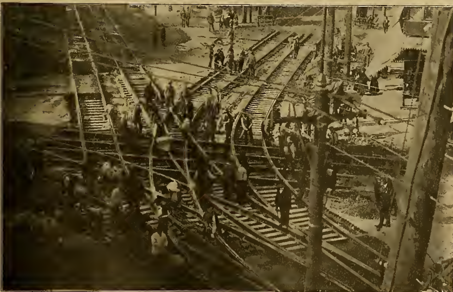
A DIFFICULT PIECE OF SPECIAL TRACK WORK IN CHICAGO
