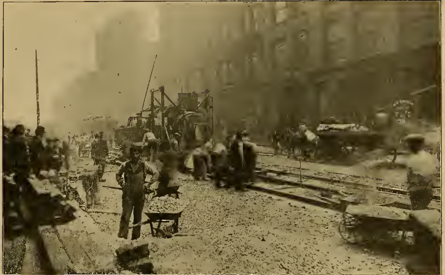
ELECTRICALLY DRIVEN CONCRETE-MIXING MACHINE IN USE ON TRACK WORK IN DOWNTOWN STREET, CHICAGO
