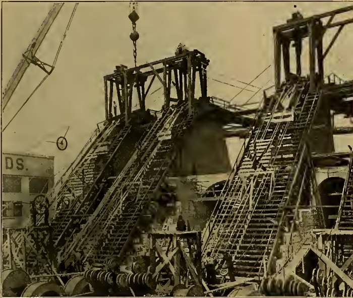
View of Brooklyn Anchorage, Showing Hauling Sheave Starting Across
