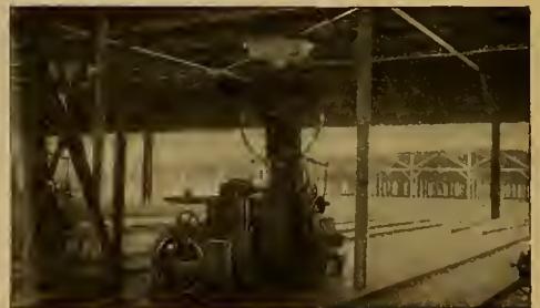
FIG. 6. MOTOR-DRIVEN BAND RESAW, SHOWING MOTOR STARTER
