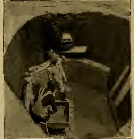
FIG. 5. BUILDING A BRICK MANHOLE
