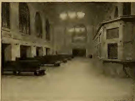
Fig. 2. Night Illumination with Arc-light Diffusers
