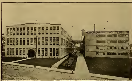
MAIN AND STORAGE BUILDINGS OF A MODERN LAMP FACTORY
