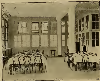
Employees' Dining Room
