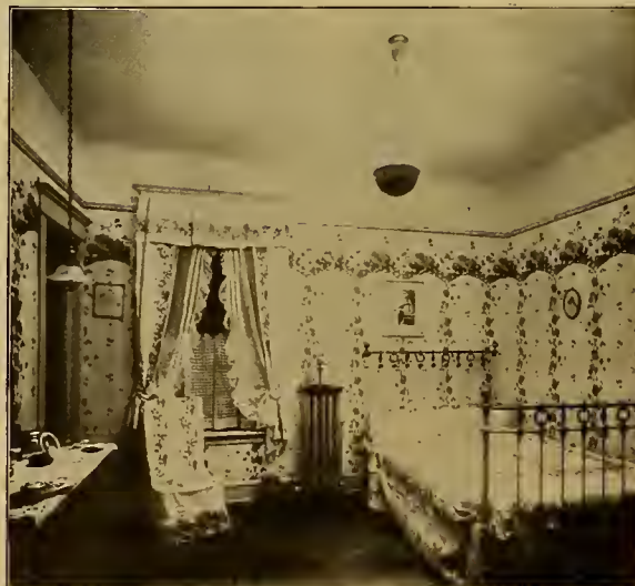
Bedroom Illuminated by Single-unit Fixture Containing One 60-watt Tungsten Lamp. Photographed by Light of the Unit
