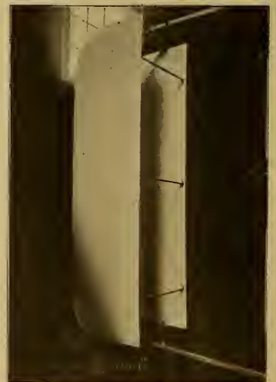
Copyright, 1908, by Waldon Fawcett, Washington, D. C. FIG. 14. BACK VERTICAL-PLANE RUDDER
