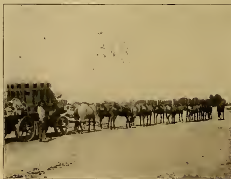
HAULING MACHINERY TO THE POWER HOUSE AT ROOSEVELT DAM
