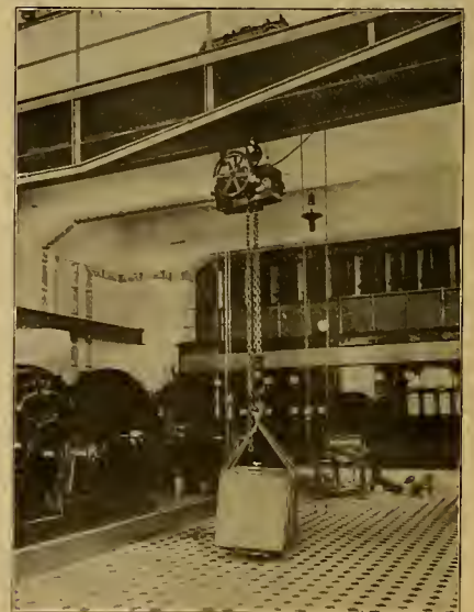
FIG. 2. DIRECT-CURRENT HOISTING BLOCK IN USE IN CENTRAL STATION.
