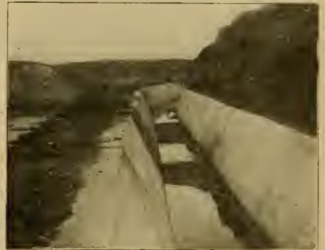
PORTION OF CONCRETE-LINED POWER CANAL TO ROOSEVELT POWER HOUSE
