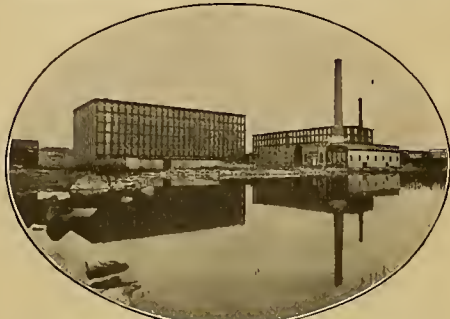
Power Plant at Water's Edge MILLS OF THE AMERICAN THREAD COMPANY, FALL RIVER
