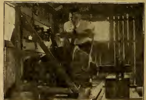
OPERATOR USING GROOVE CUTTER ON EXTENDED SHAFT OF CONTRACTOR'S MOTOR
