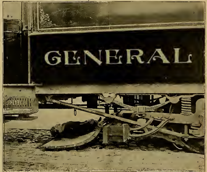
Boy Dummy Picked Up by Wright-Clark Wheel Guard on Cobble-paved Track
