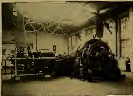
Direct-connected Generating Unit
