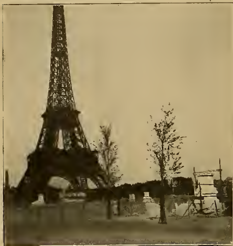
FIG. 1. NEW "WIRELESS" PLANT FOR EIFFEL TOWER, SHOWING STONE ANCHOR PILLARS FOR AERIAL WIRES
