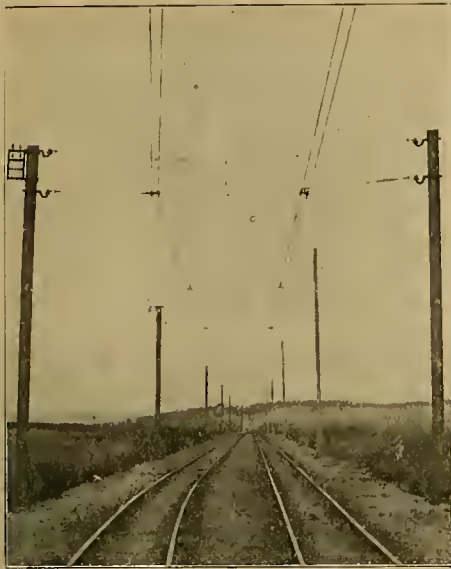
Fig. 7. Double-track Line Construction A 2,000-VOLT DIRECT-CURRENT FREIGHT RAILWAY
