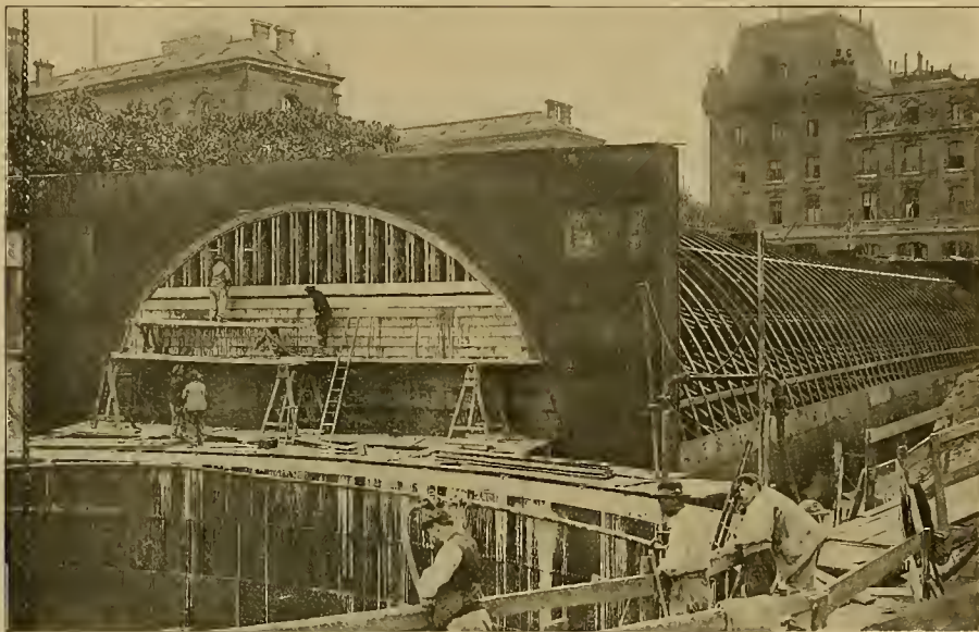
MIDDLE CAISSON OF PARIS UNDERGROUND RAILWAY STATION.
