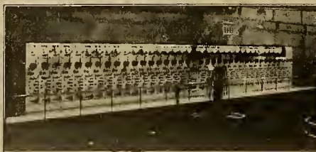
Fig. 3. Switchboard with Mercury-arc Rectifiers—Night View
