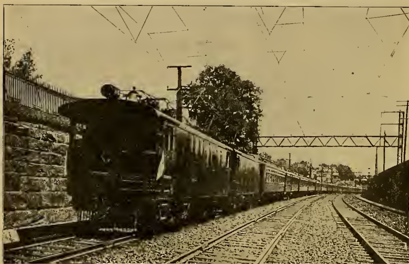
New York, New Haven & Hartford Passenger Train—Double-Catenary Suspension of 11,000-volt, 25-cycle Power Wire
