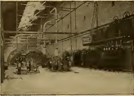
FIG. 2. POWER PLANT AT BOGALUSA LUMBER MILL
