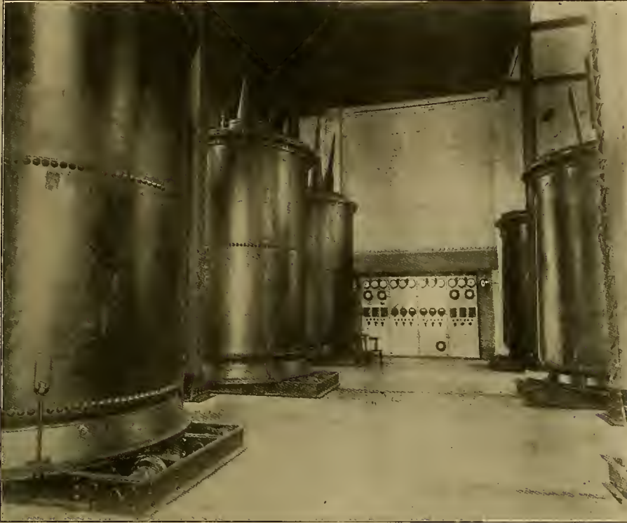
On the Left are the 110,000-volt Transformers, Stepping Down to 20,000 Volts and 7,200 Volts. The 72,000-volt Transformers are Seen at the Right
