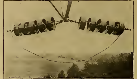
FIG. 5. 110,000-VOLT STRAIN INSULATOR
