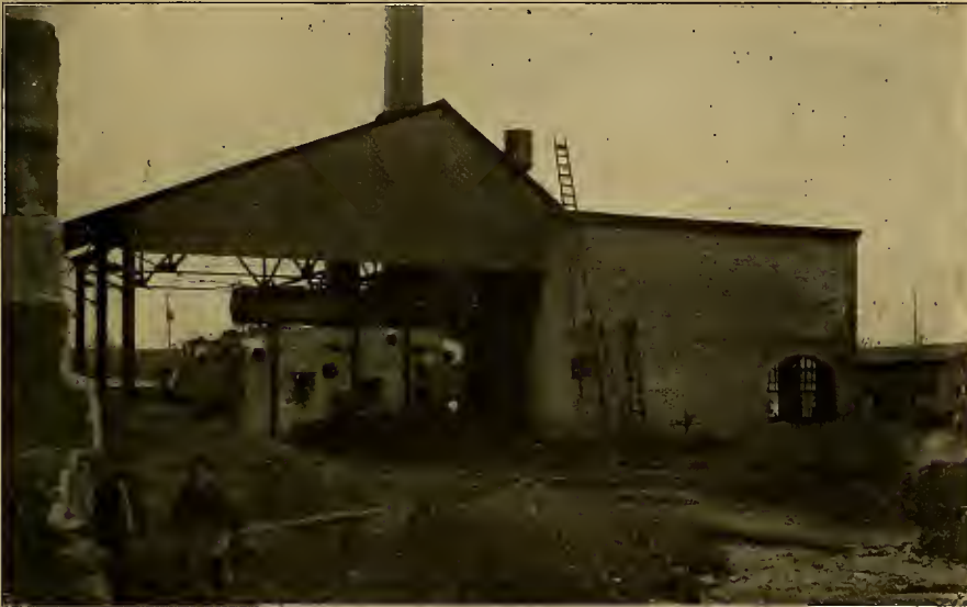
The Excavation in Foreground Is for a Cooling Tower. It Will Be Noted that Boiler Room Is Not Enclosed. POWER HOUSE FOR MONTEREY ELECTRIC RAILWAYS
