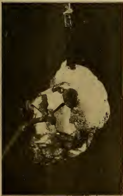
COLLECTION OF SALTS ON WIRE IN DAMP BASEMENT.
