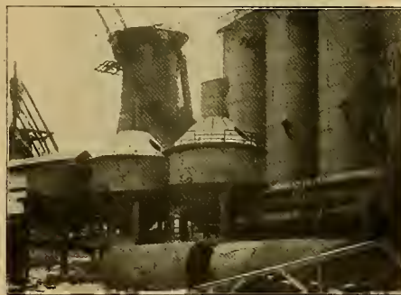
BLAST FURNACE GROUP, SHOWING PRIMARY WASHERS OF GAS-CLEANING SYSTEM
