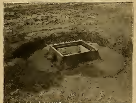
FIG. 9. CONCRETE ROOF OF MANHOLE WITH IRON FRAME FOR COVER
