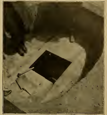
FIG. 8. FORM FOR CONCRETE TOP OF MANHOLE IN PLACE
