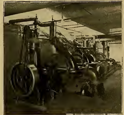
CENTRIFUGAL PUMPS FOR BAROMETRIC CONDENSERS IN FALK COMPANY'S PLANT
