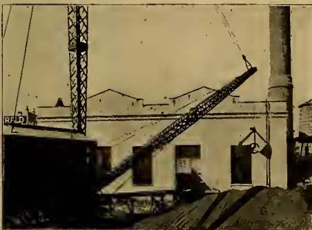
FIG. 6. COAL-HANDLING APPARATUS AT GRAND FORKS STATION
