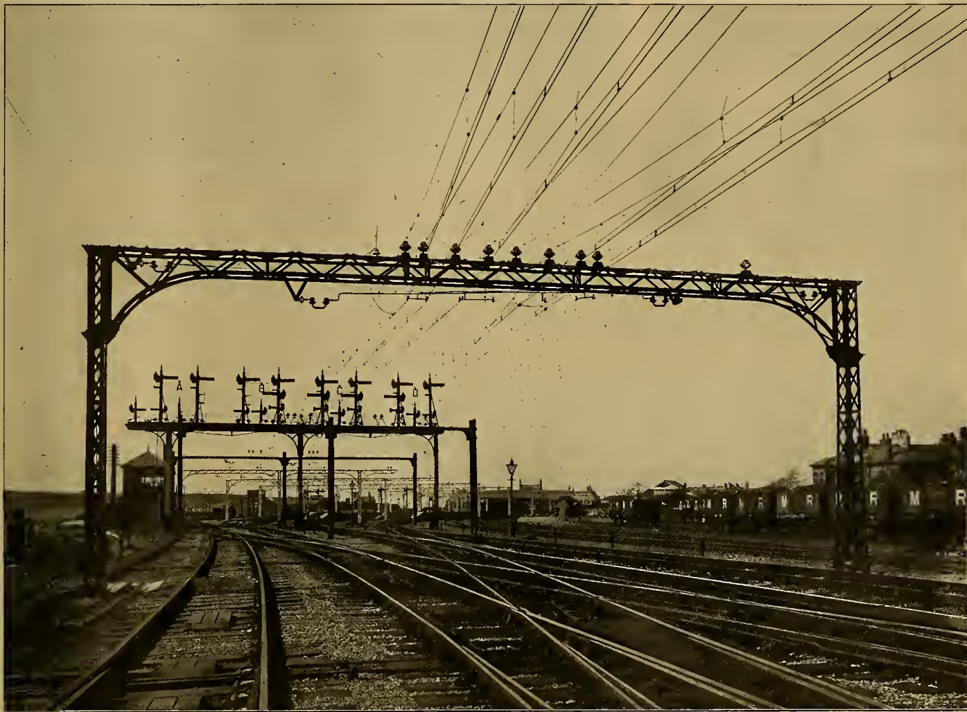
WIDE-SPAN SUPPORTING BRIDGE FOR OVERHEAD CONSTRUCTION FOR FIRST SINGLE-PHASE RAILWAY IN ENGLAND.
