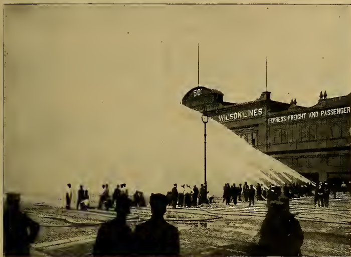
TEST OF HIGH-PRESSURE FIRE SERVICE IN NEW YORK CITY
