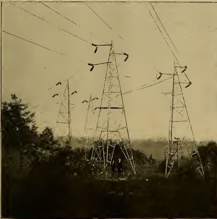
Fig. 1. A Right-angle Turn on the 110,000-volt and 72,000-volt Tower-lines Near Grand Rapids. The 110,000-volt Lines Are on the Right or Outer Side of the Turn
