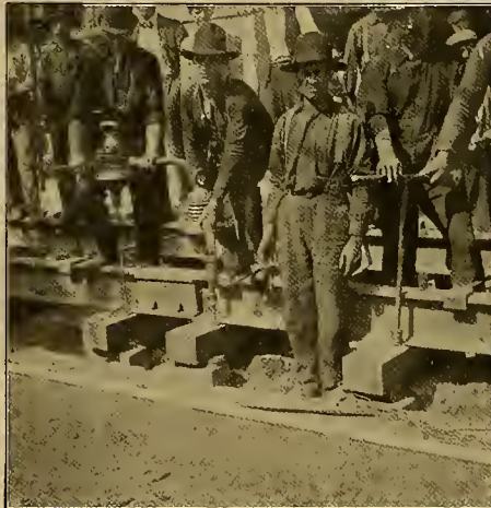
ELECTRIC SPIKING MACHINES USED ON TRACK CONSTRUCTION IN CHICAGO
