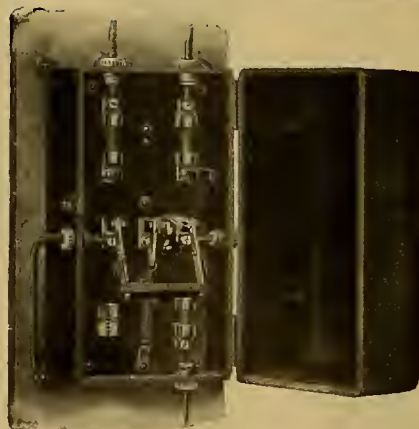
Showing M. & R. Cut-out after operating.
