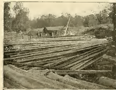
POLE YARD AT CLAY ROOT, MO.
