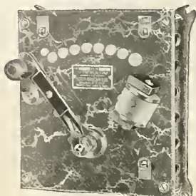
Motor Starting Rheostat with no voltage release. (Bulletin 10.)
