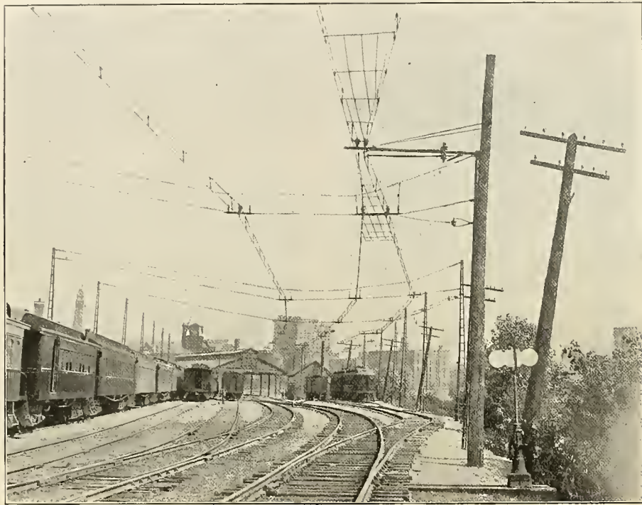
Overhead Construction at Rochester Terminal. SINGLE-PHASE OPERATION ON ROCHESTER DIVISION OF ERIE RAILROAD.
