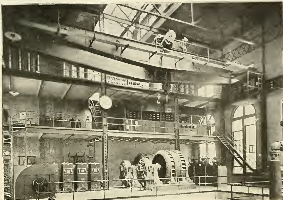
Fig. 1. North End of Generator Room, showing Transformers, Frequency Changers, Switchboard Gallery, Lightning Arresters and Traveling Crane.
