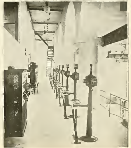
FIG. 8. CENTRALIZED SWITCHING COLUMNS IN OBERMATT POWER STATION.
