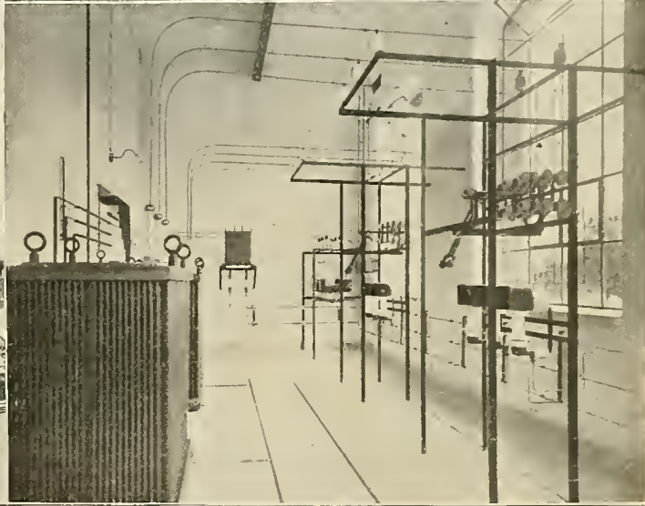
Car Barn and Repair Shop. Transformer Room in Sub-station.
