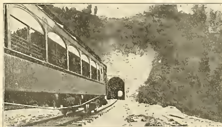
COLFAX TUNNEL ON THE INLAND EMPIRE SYSTEM.
