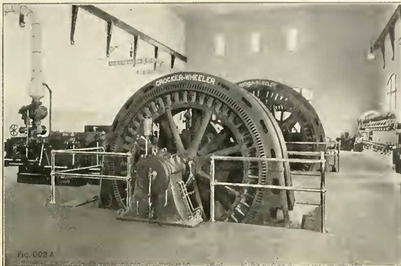
Two 500 K. V. A. and One 200 K. V. A. Generators, Elgin National Watch Co., Elgin, Ill.
