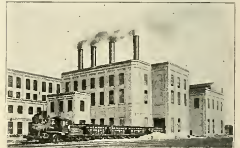
STEEL COAL CARS AT WEST ALLIS TOWER HOUSE.
