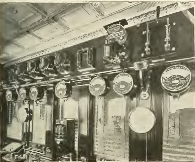
INTERIOR OF CONTROLLING HOUSE, PYRMONT BRIDGE.
