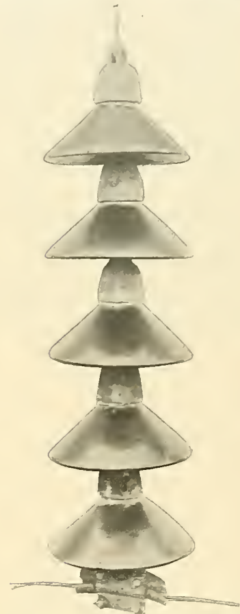
NEW SUSPENSION-TYPE INSULATOR FOR HIGH-VOLTAGE TRANSMISSION.
