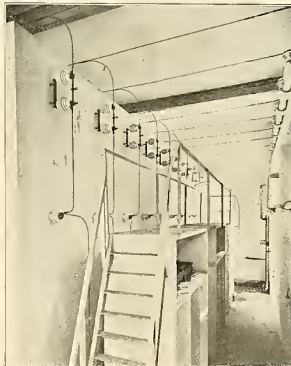
FIG. 7. CONNECTIONS BETWEEN THE LIGHTNING ARRESTERS AND OUTGOING LINES.
