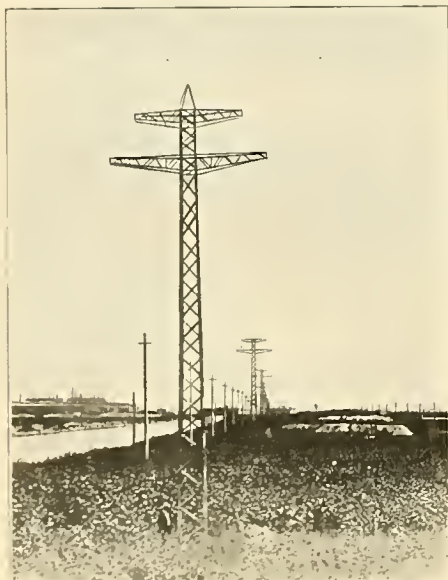
FIG. 5. VIEW OF LOCKPORT-CHICAGO TRANSMISSION LINE, WITH SUB-STATION IN THE DISTANCE.
