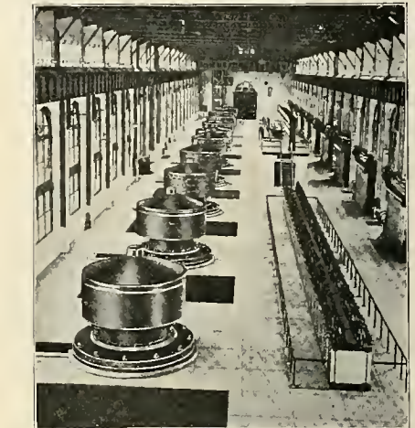
INTERIOR OF A NIAGARA FALLS POWER HOUSE, SHOWING 10 VERTICAL 5,000-HORSEPOWER GENERATORS.
