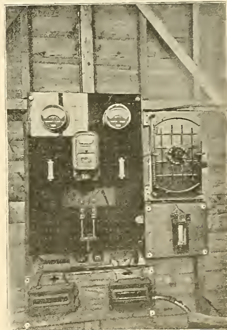
FIG. 2. SWITCHBOARD AND CURRENT REGULATOR IN POPLAR DISINFECTANT PLANT.
