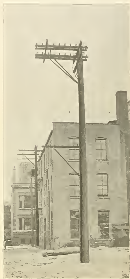
FIG. 3. POLE WITH IRON PIPE CONTAINING ELECTRIC-LIGHT WIRES CONNECTING OVERHEAD AND UNDERGROUND WORK AND PASSING TELEPHONE CROSS-ARM.
