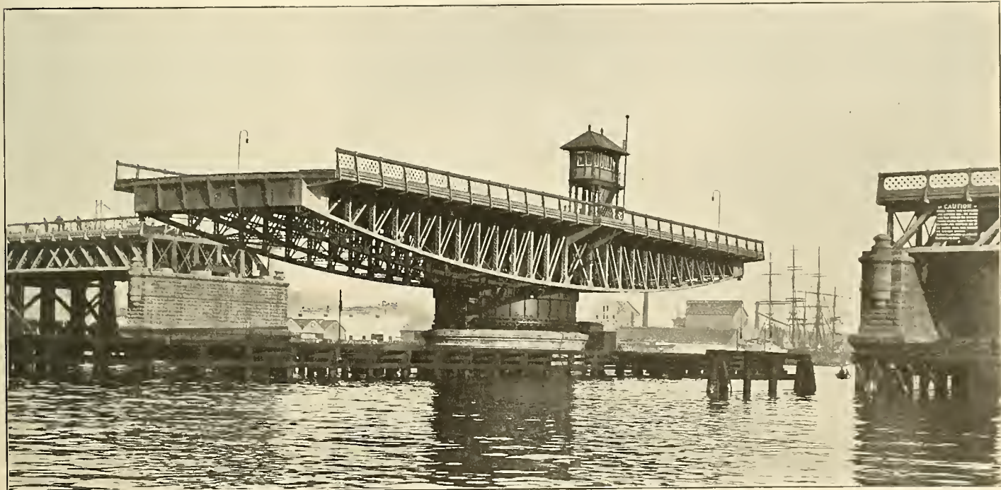
ELECTRIC SWING SPAN OF PYRMONT BRIDGE, SYDNEY, AUSTRALIA.
