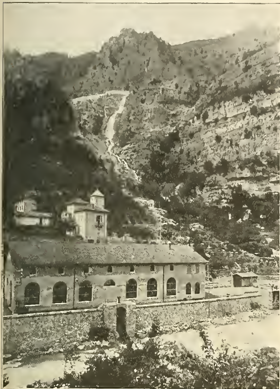
PATARAS HYDRO-ELECTRIC STATION ON THE LOUP RIVER, FRANCE.
