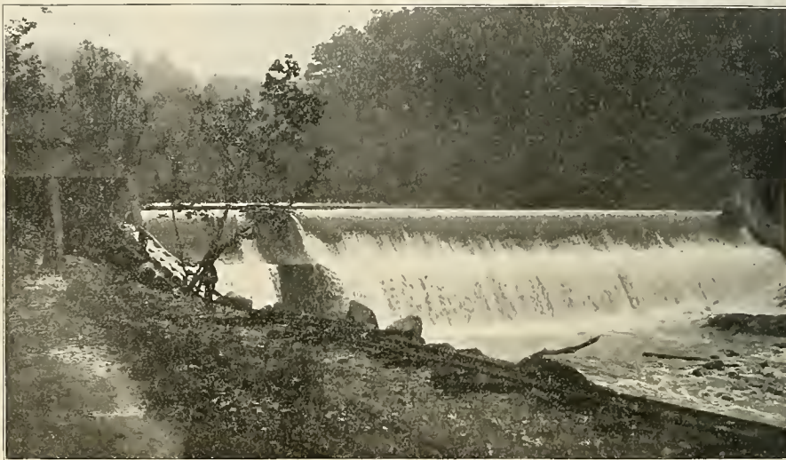
PATAPSCO RIVER DAM WITH POWER PLANT INSIDE.
