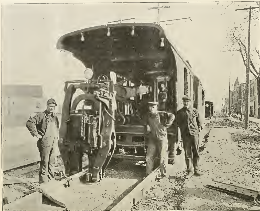
FIG. 2. FRONT VIEW OF ELECTRIC TRACK-WELDING OUTFIT.
