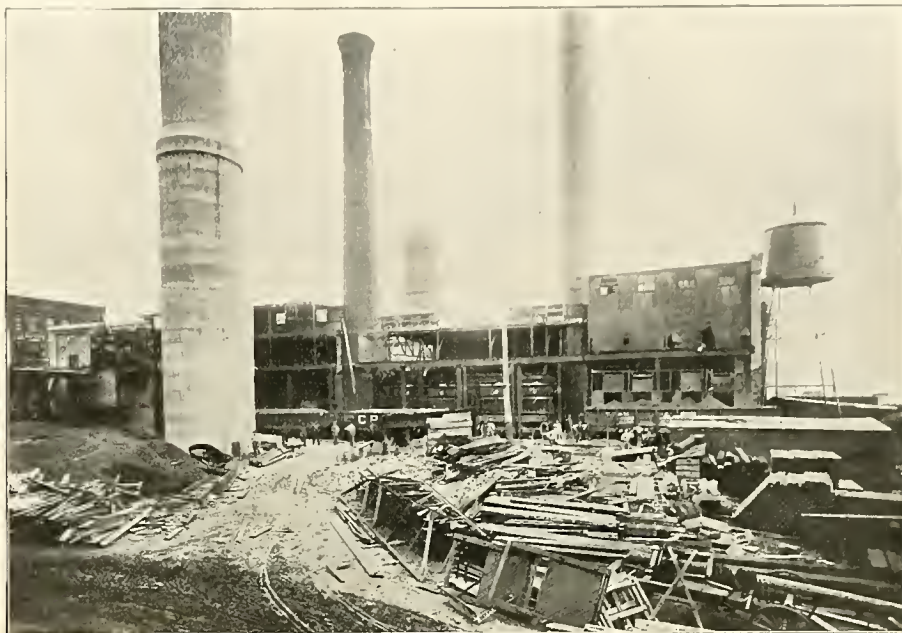
REBUILDING CENTRAL-STATION BOILER ROOM IN PEORIA DURING OPERATION.
