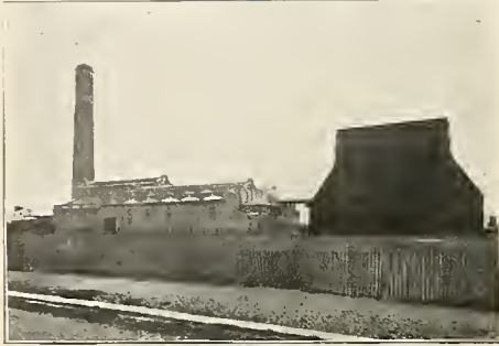
EXTERIOR OF THE PARK ROYAL POWER HOUSE OF THE GREAT WESTERN RAILWAY.
