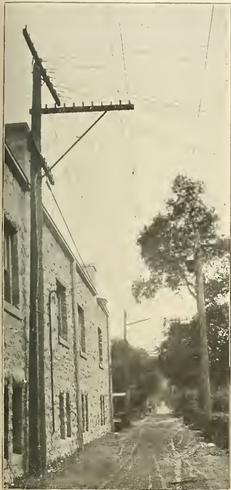
FIG. 1. TELEPHONE WIRES CROSSING ABOVE ELECTRIC-LIGHT PRIMARY CIRCUIT IN ALLEY.
