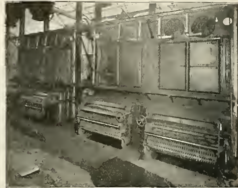
FIG. 6. BOILER ROOM IN BLUE ISLAND STATION OF THE NORTH SHORE COMPANY.
