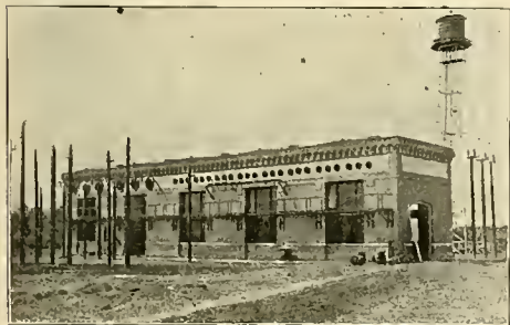
LOCKPORT SUB-STATION, SHOWING 11,000-VOLT OUTDOOR LIGHTNING ARRESTER.
