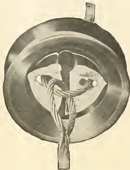
FIG. 2. LOOP OF TIE WIRES INTERMESSED IN A BROKEN INSULATOR.
