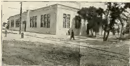
FIG. 1. POWER AND ALCOHOL BUILDING, JAMESTOWN EXPOSITION, CONTAINING FUEL-TESTING PLANT.
