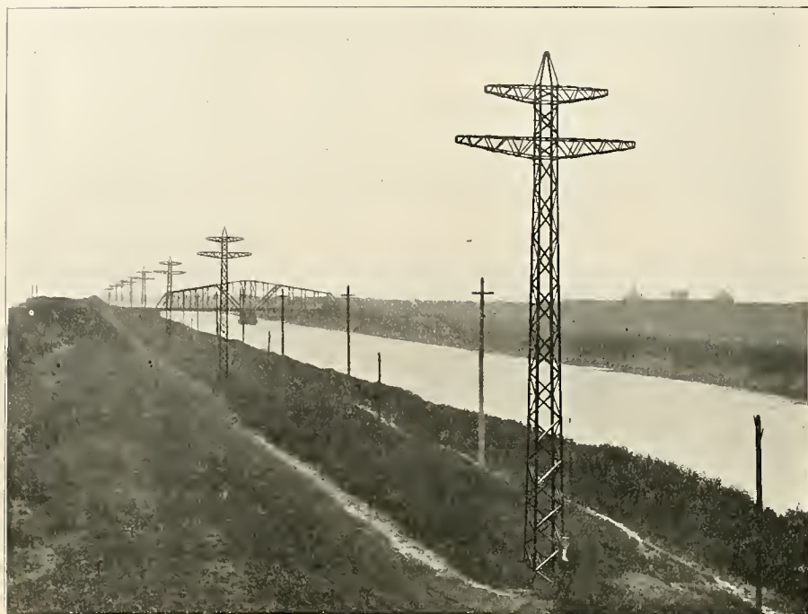
FIG. 4. VIEW ON CHICAGO DRAINAGE CANAL, SHOWING LOCKPORT-CHICAGO TRANSMISSION LINE.
