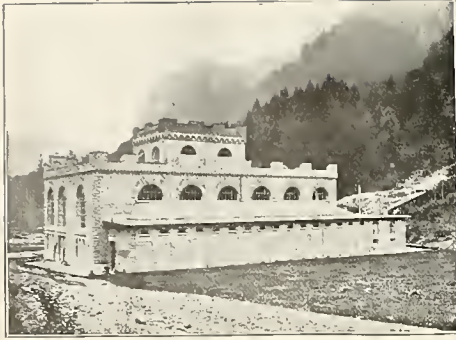
FIG. 2. REAR VIEW OF POWER STATION WITH TRANSFORMER HOUSE ADDITION.
