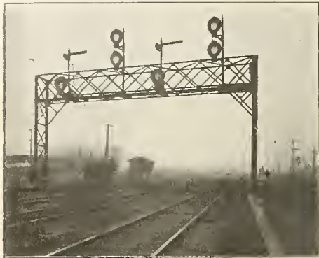
Interlocking Tower in the Distance.
