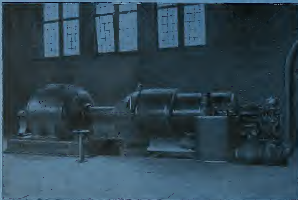
1,000 K. W., Allis-Chalmers Steam Turbine and Generator
