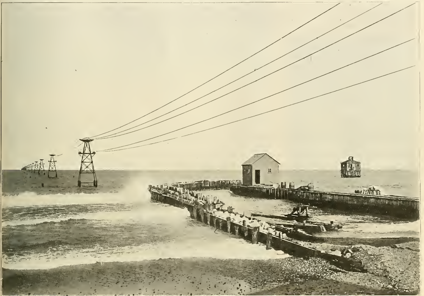
FIG. 1. AERIAL TRAMWAY OVER LAKE MICHIGAN, USED IN CONSTRUCTING SOUTHWEST LAND AND LAKE TUNNEL.
