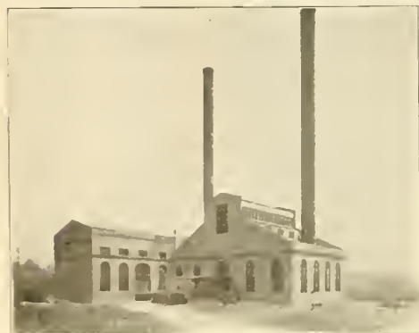
FIG. 4. PRESENT EXTERIOR VIEW OF NORTH SHORE POWER STATION AT BLUE ISLAND.
