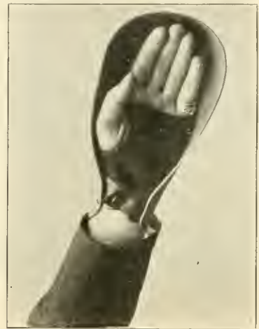
FIG. 4. PROTECTIVE GLOVE FOR X-RAY OPERATORS.
