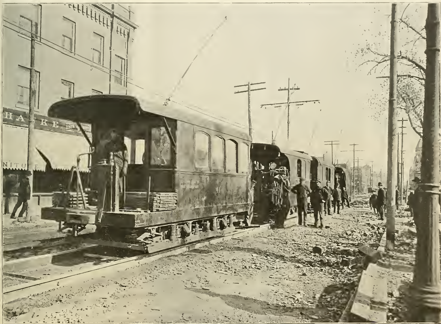
FIG. 1. ELECTRIC TRACK-WELDING OUTFIT ON A CHICAGO STREET.
