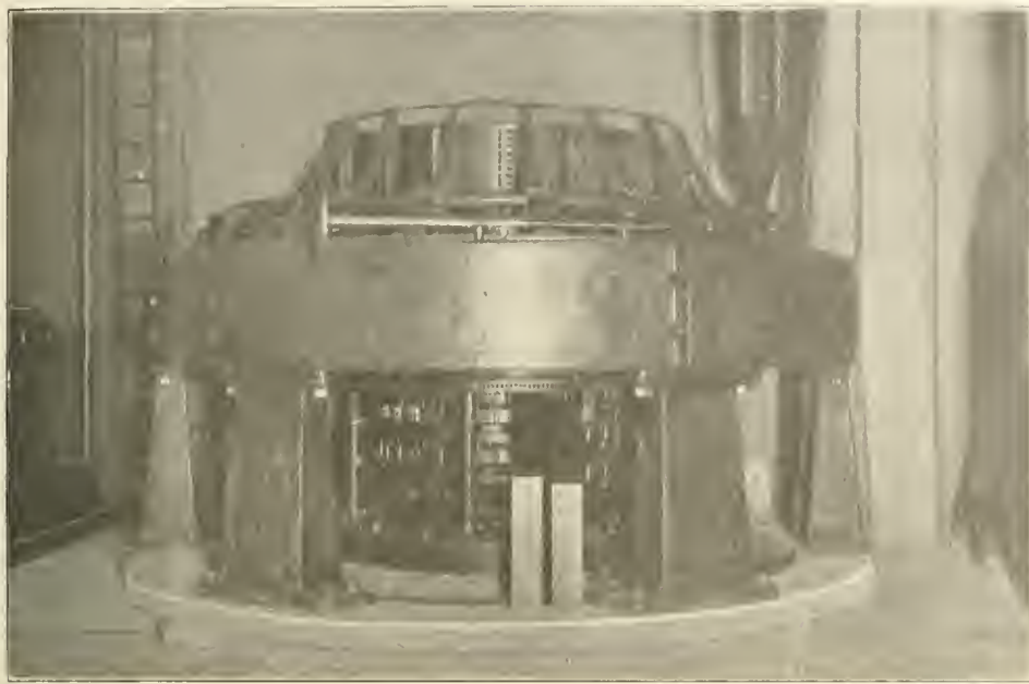
FIRST 2,000-KILOWATT VERTICAL-SHAFT ROTARY CONVERTER IN SERVICE.
