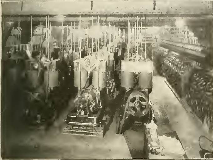
Bipolar Edison Dynamos on Upper Level.
