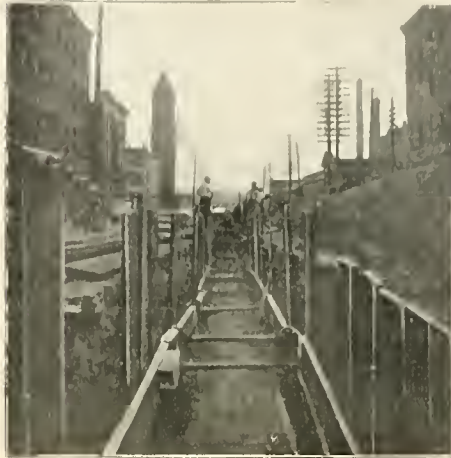
UNDERGROUND WORK IN LIBERTY STREET, PEORIA.
