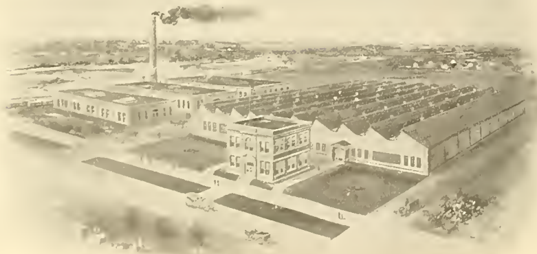
WARNER INSTRUMENT PLANT IN BELOIT
