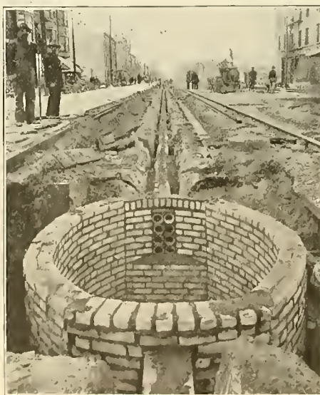
FIG. 3. FEEDER DUCTS IN OLD STREET-RAILWAY CABLE TRENCH, CHICAGO.
