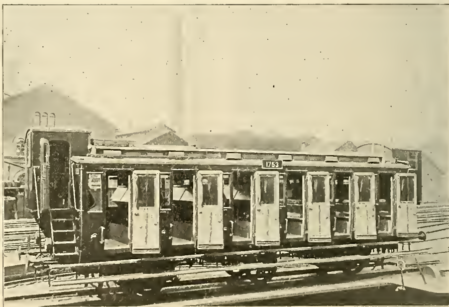
BATTERY-PROPELLED CAR WITH DOORS OPEN SHOWING BATTERY COMPARTMENTS UNDER THE SEATS.
