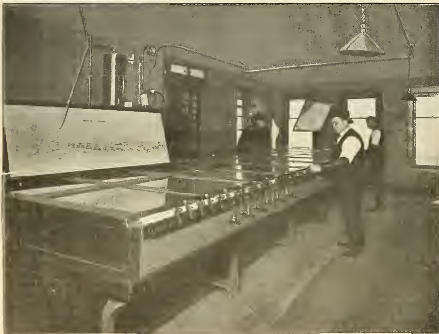
FIG. 3. NEW ELECTRO-PNEUMATIC INTERLOCKING MACHINE IN THE WESTERN AVENUE TOWER, CHICAGO.
