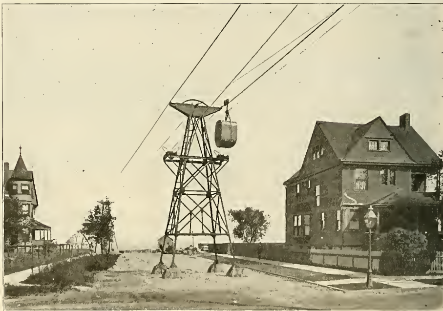
FIG. 5. TOWER AND CABLE CONSTRUCTION OF AERIAL TRAMWAY.—FIRST CAR RETURNING FROM THE LAKE.
