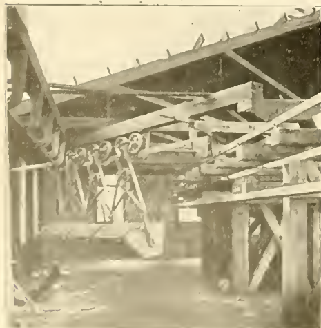
FIG. 4. VIEW IN TERMINAL STATION OF AERIAL TRAMWAY, SHOWING TRAVELING BUCKETS.
