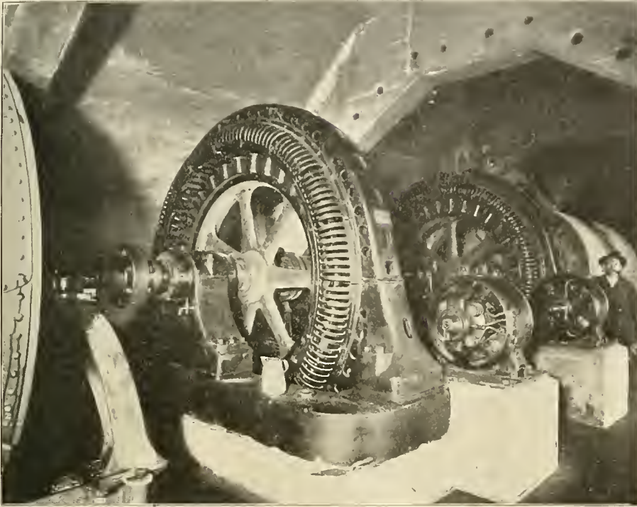
HYDRO-ELECTRIC POWER PLANT INSIDE PATAPSCO RIVER DAM.
