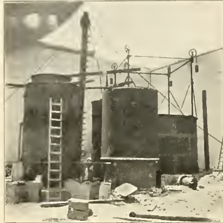
FIG. 4. GAS-PRODUCER PLANT AT JAMESTOWN FUEL-TESTING STATION.
