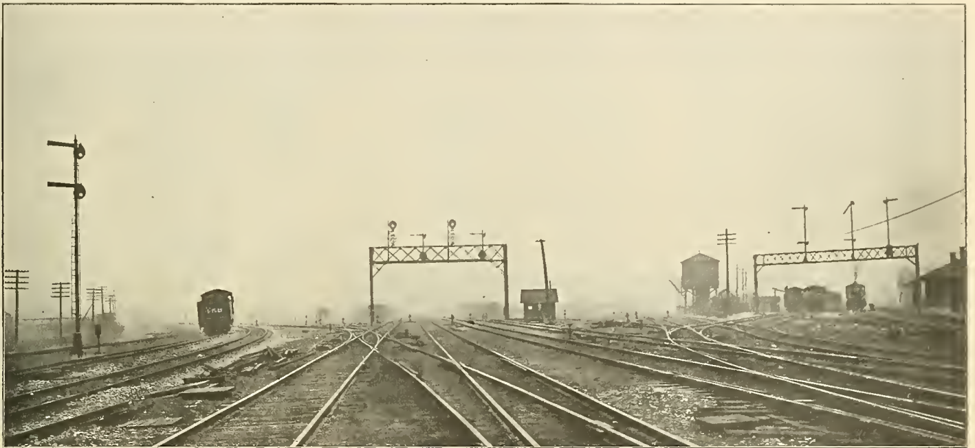
FIG. 1. ELECTRO-PNEUMATIC INTERLOCKING SYSTEM AT THE JUNCTION OF PENNSYLVANIA, NORTHWESTERN AND ST. PAUL RAILROADS IN CHICAGO.
