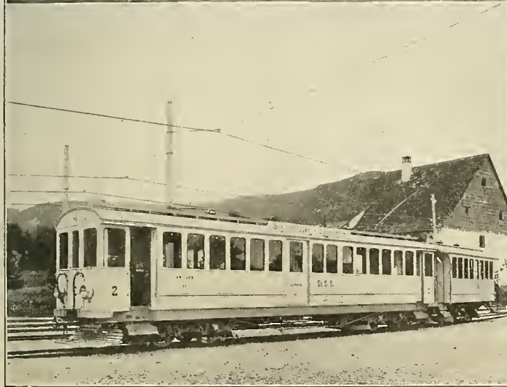
View of Track and Trolley Construction. A Motor Car and Trailer.
