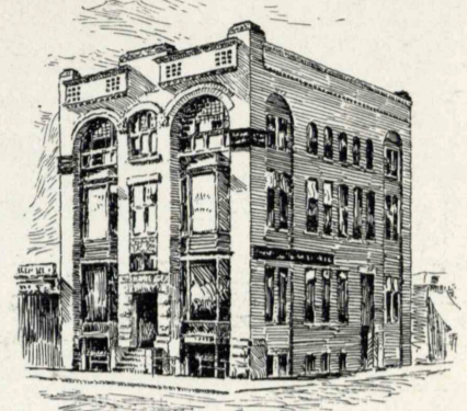
FIRST NATIONAL BANK, KANSAS CITY, KAN. HEATED BY BOLTON HEATER
