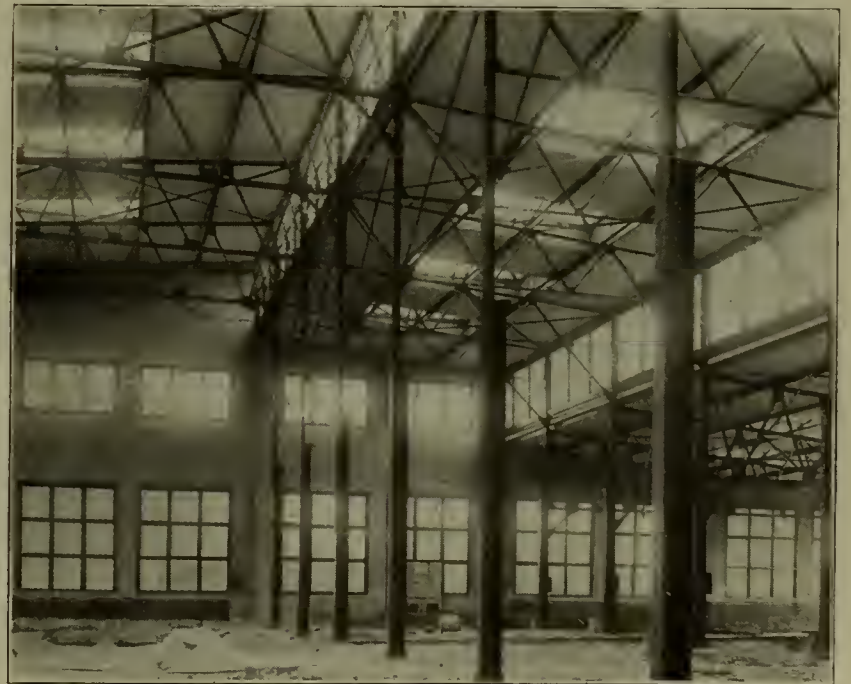
Interior of Coach and Boiler Shop.
