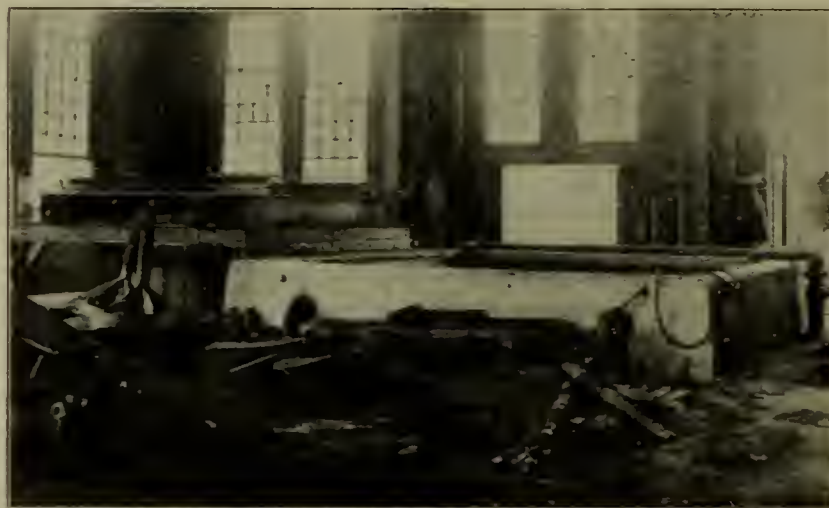
Fig. 4—Heat Treating Plant at Juniata Shops, P. R. R.
