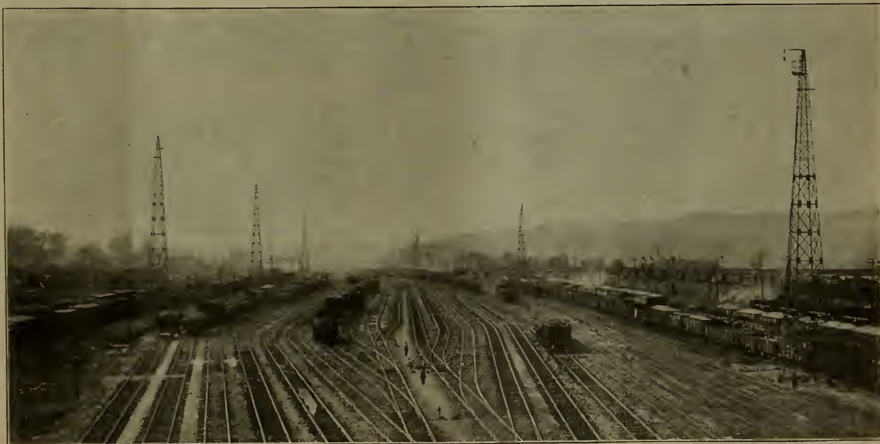
Classification Yard of P. & L. E. at McKees Rocks, Showing Lighting Towers.
