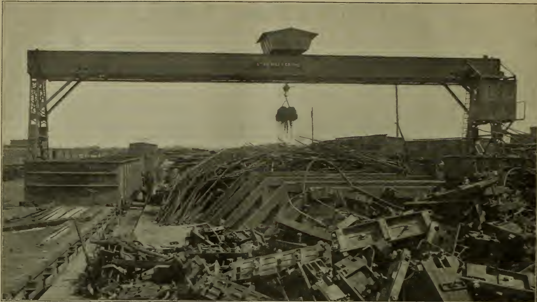
Scrap Platform, Bins and Crane, with Lifting Magnet, B. & A. R. R.
