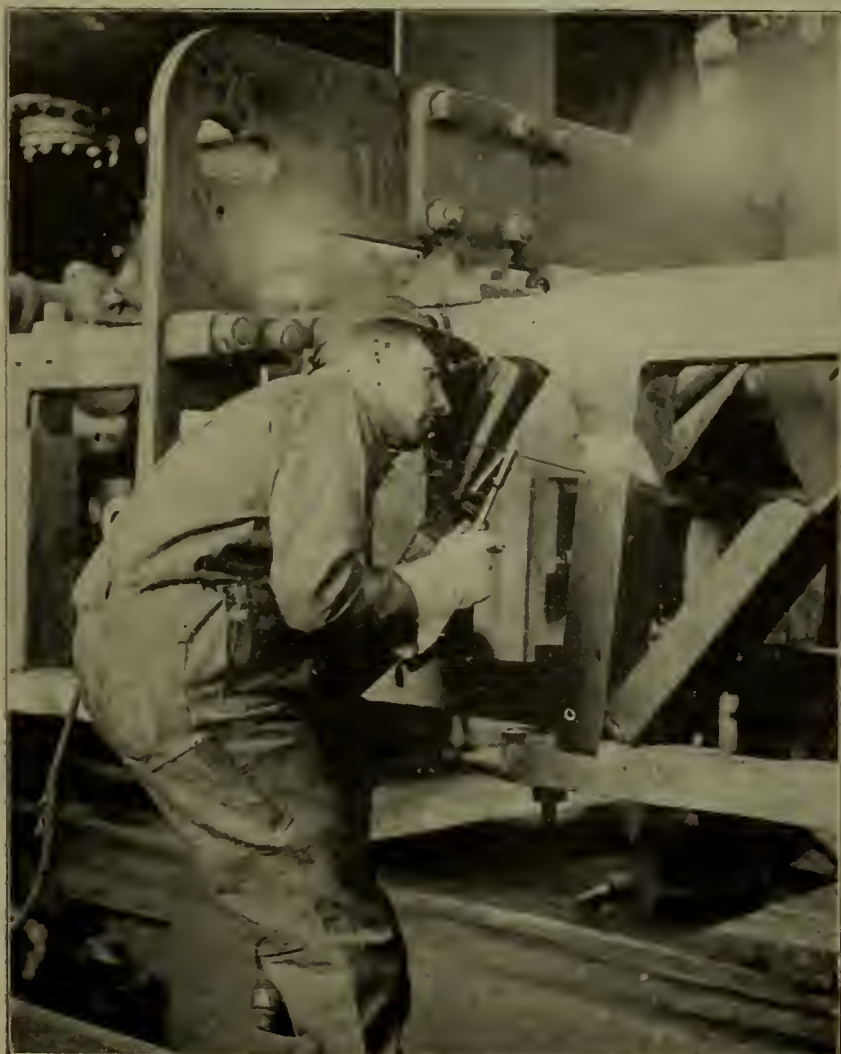
Repairing Broken Locomotive Frame.
