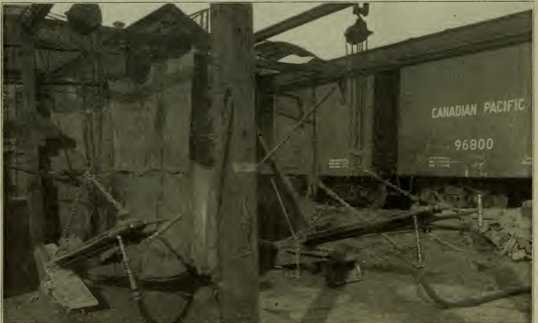
Air Hammers for Stripping Bolsters, C. P. R.
