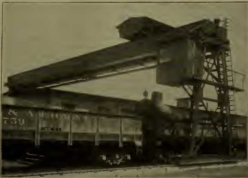
Crane Operator's Cage and Method of Collecting Current. Storehouse in Background.
