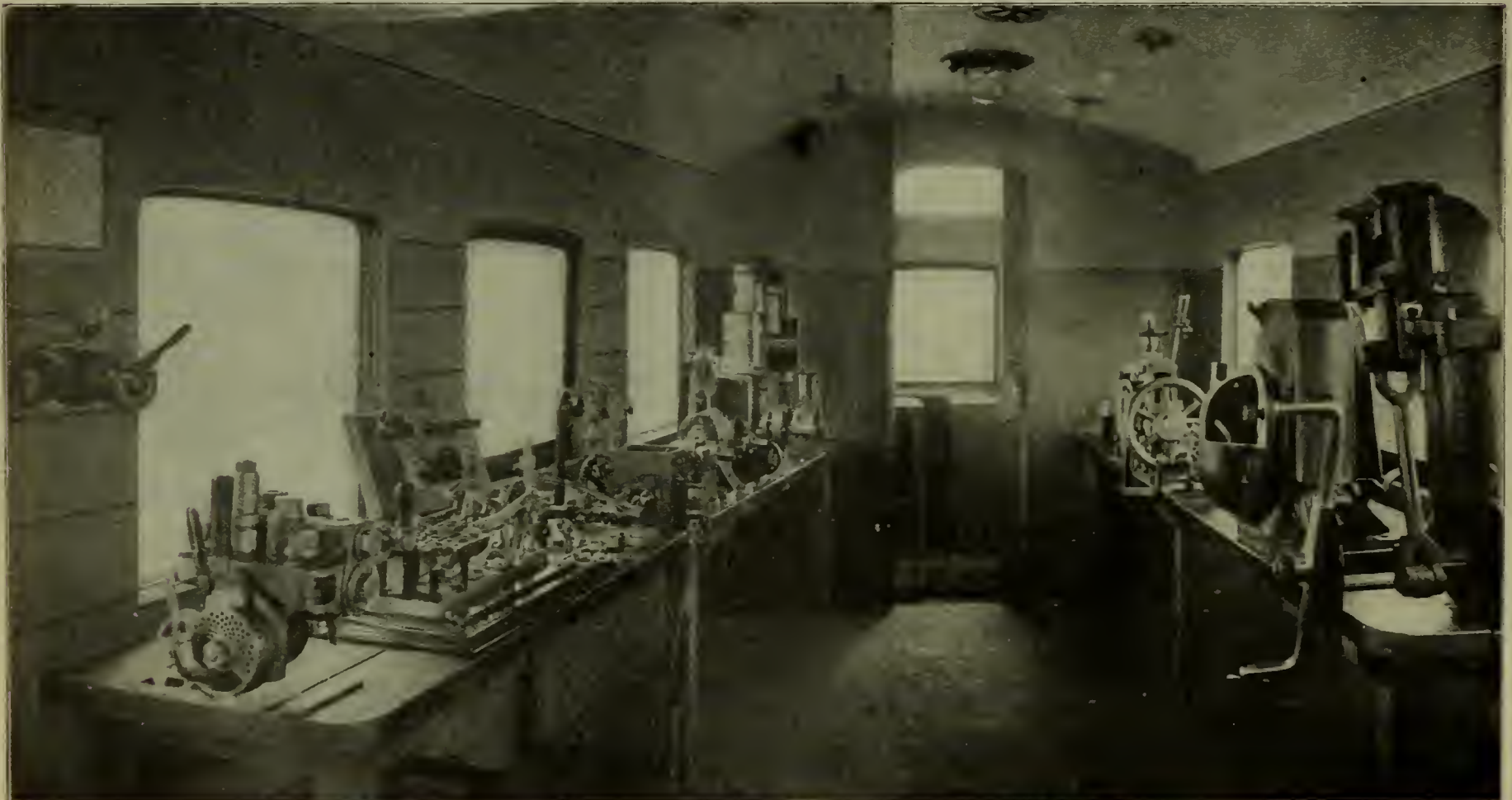
Interior of Enginemen's Instruction Car, Great Eastern R. R. of England.
