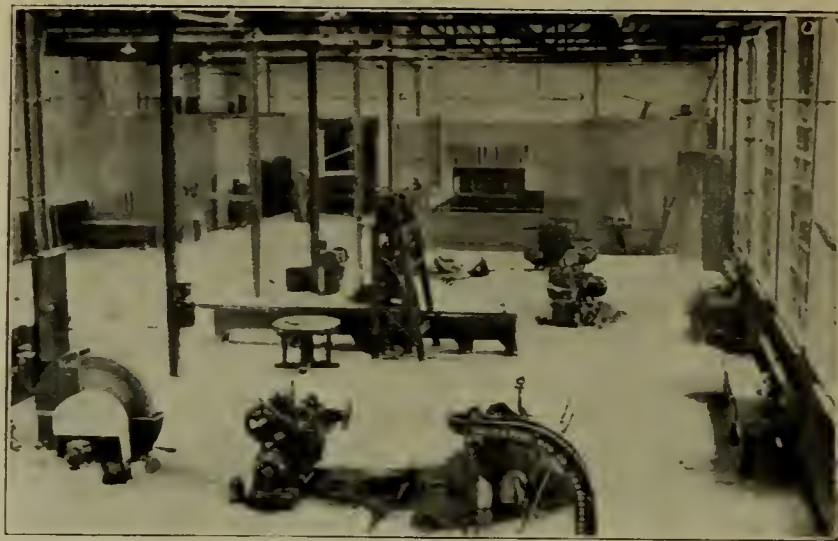
Machine Shop Looking East.
