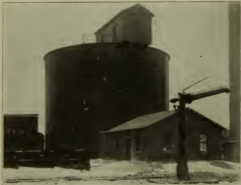
Fig. 4. Burr Oak Combination Softener and Storage Plant.
