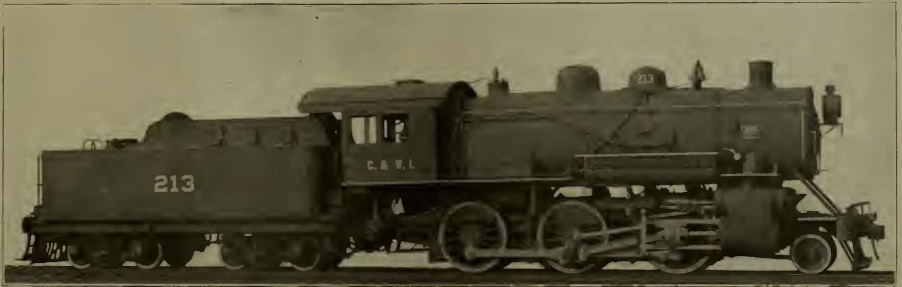
2-6-0 Switching Locomotive, C. & W. I. R. R.
