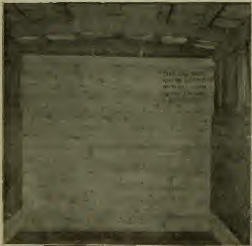
C. P. Wooden Box Car Showing Reinforcing Lining. Note Bolts Which Extend Through Lining and Outside Z Bars.
