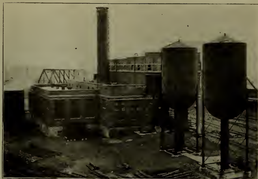
Power House and Water Tanks.
