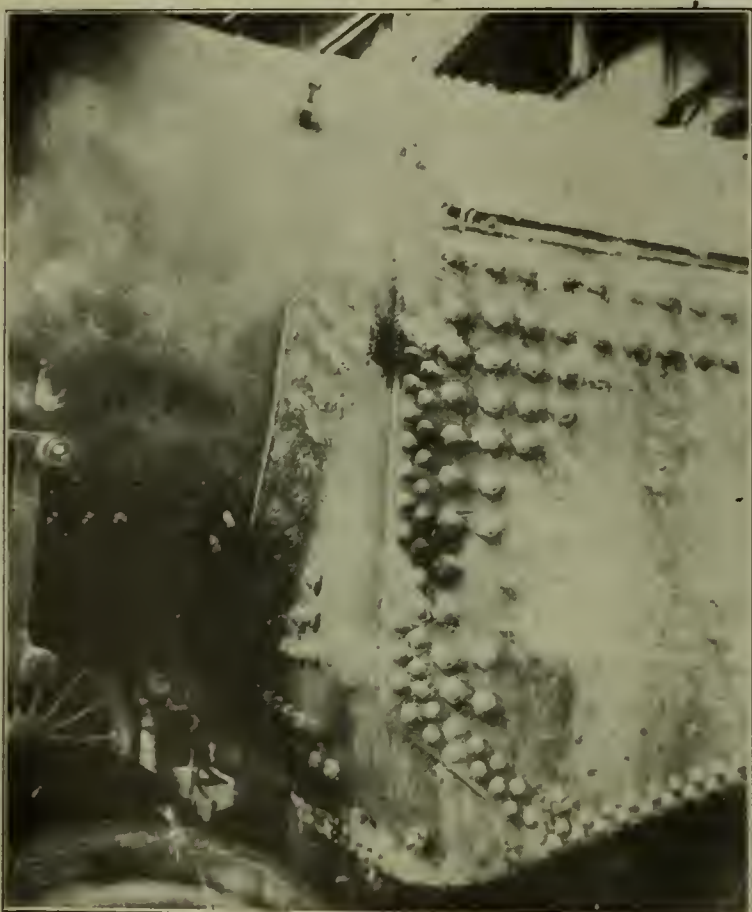
Connection Rivet Cut Off with Oxy-Acetylene Cutting Burner.
