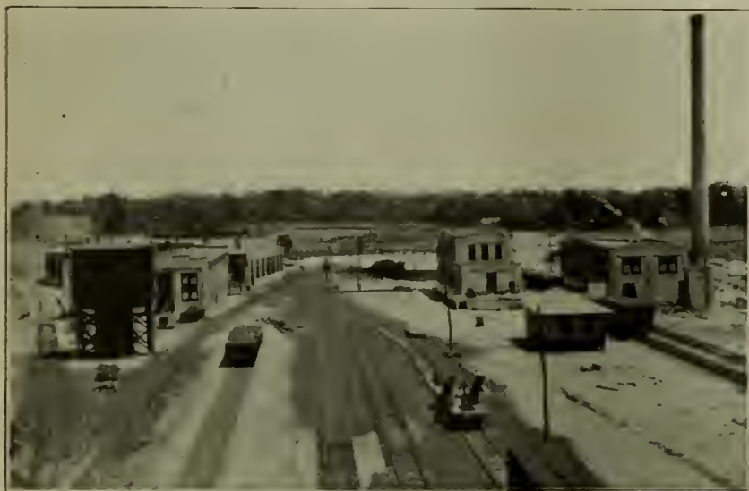
Roundhouse and Machine Shop at Left, Offices and Storeroom in Center and Powerhouse at Right.
