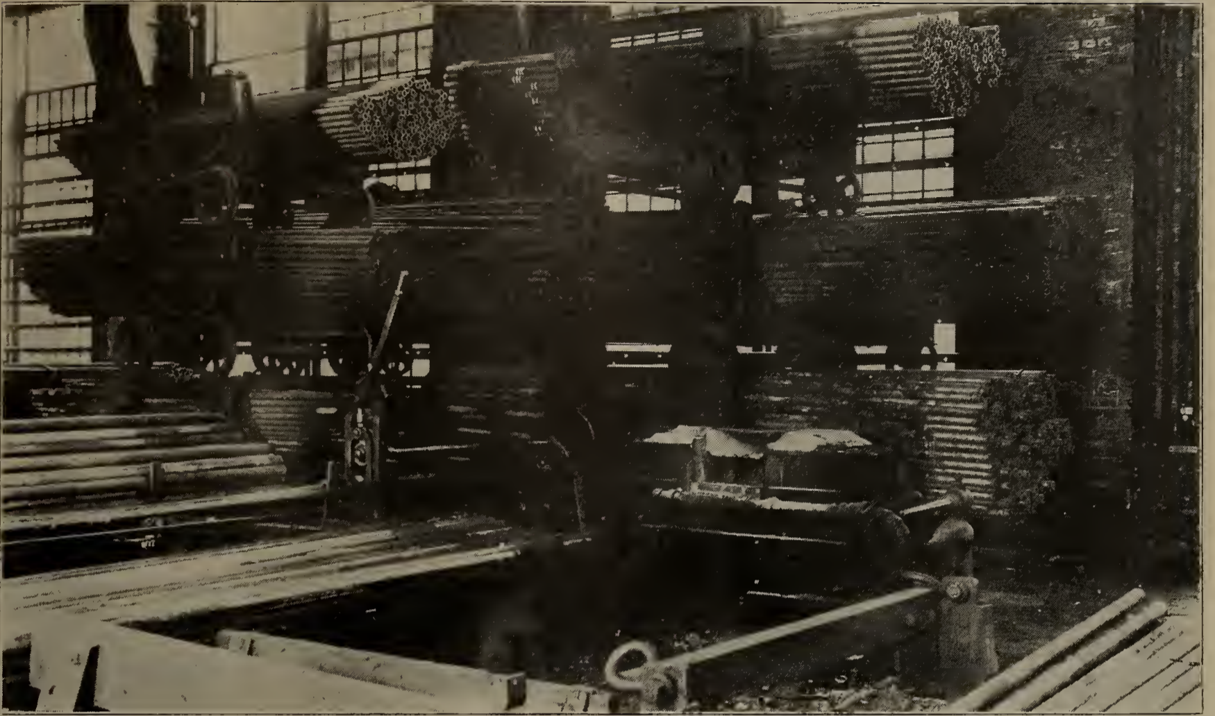
Handling Boiler Tubes, Angus Shops, Fig. 2.
