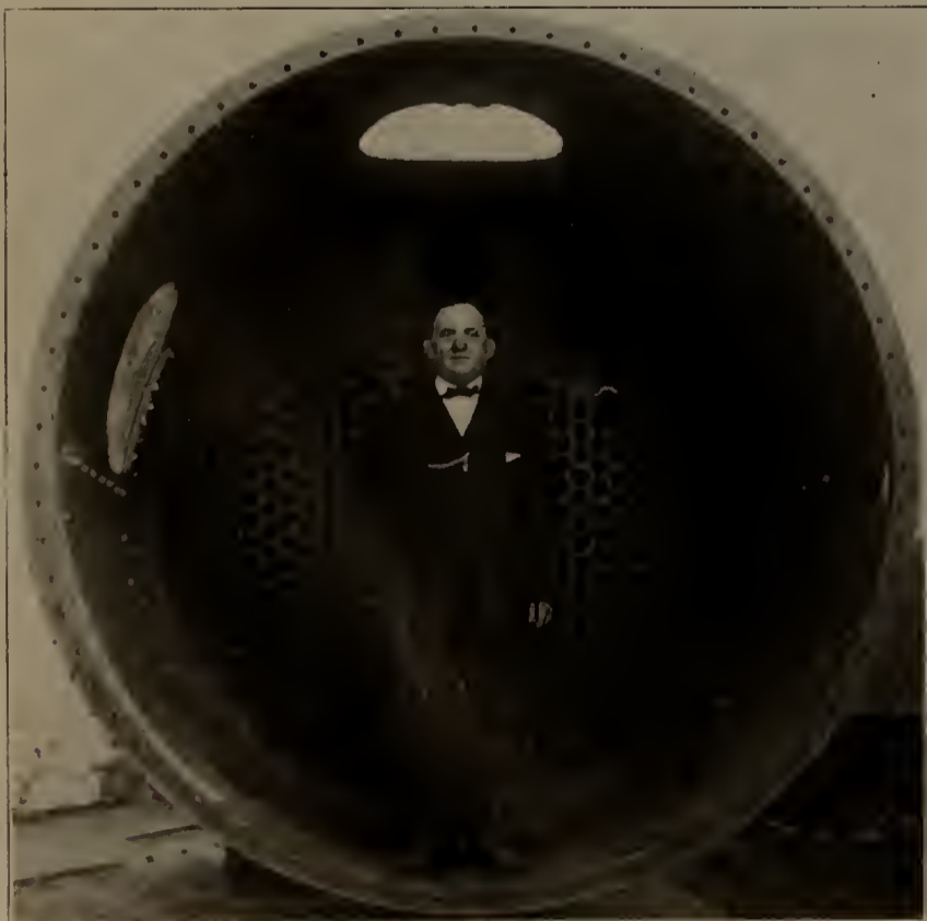
Front End of Boiler, D. & H. Mallet.
