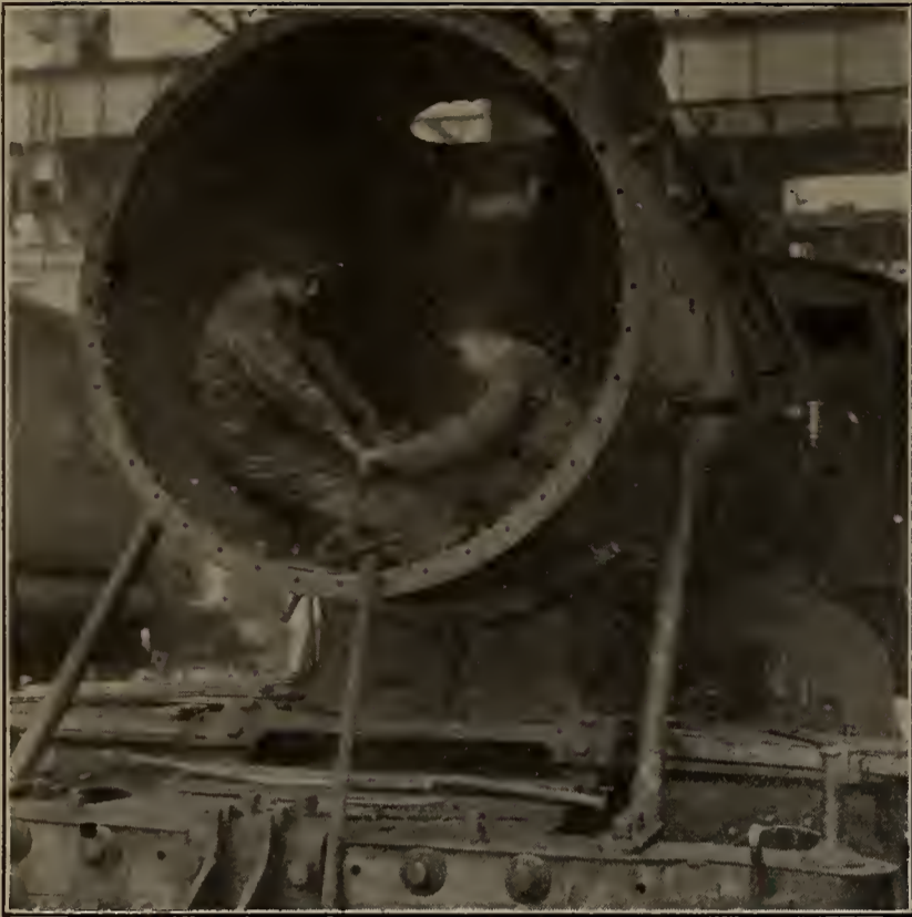
Cutting Flues, Grand Trunk Apprentices at Montreal.
