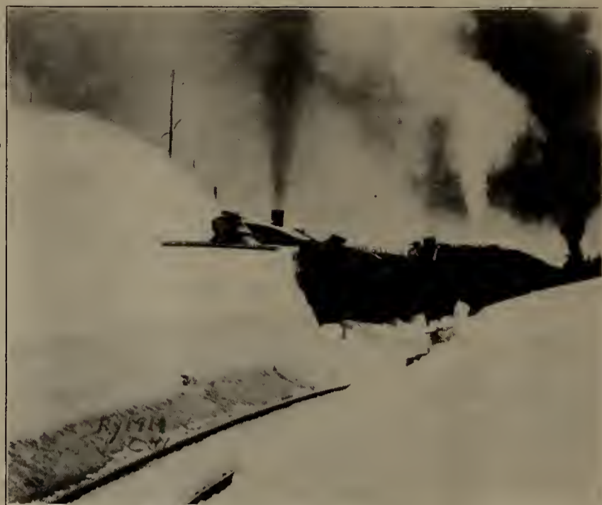
Clearing a Siding, Moffat Road.
