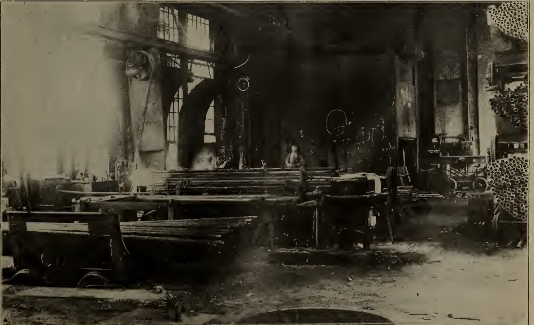
Handling Boiler Tubes, Angus Shops, Fig. 4.
