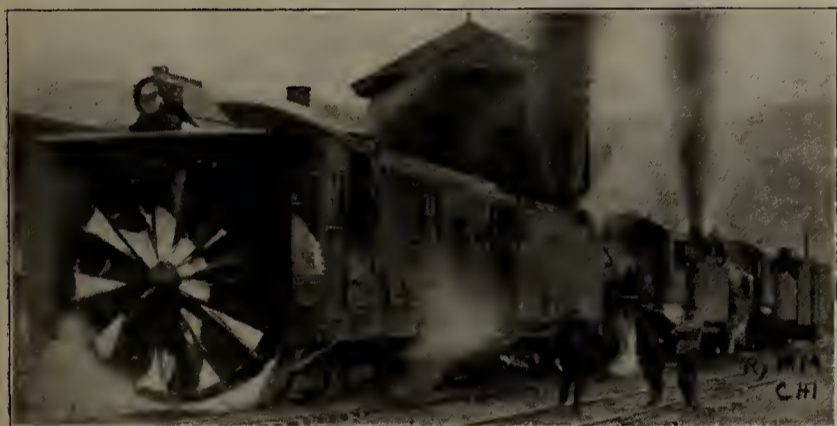
Plow and Equipment, Moffat Road.
