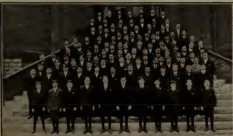
Apprentices at Stratford Shops.
