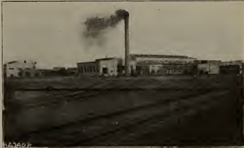
General View of Empalme Shops, Southern Pacific Co.
