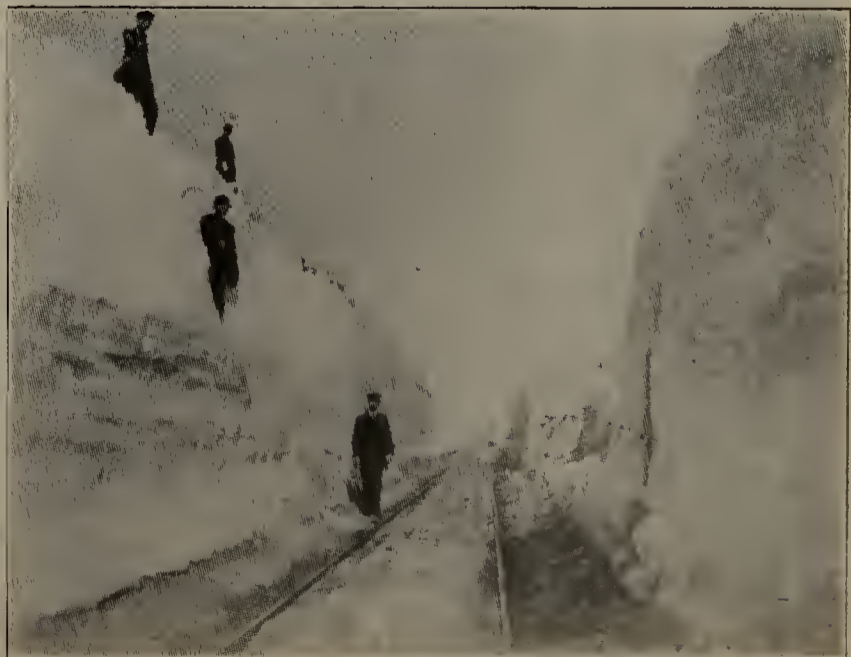
Cut 24 Feet Deep, after Passage of Rotary, C., St. P., M. &amp; O. Ry.
