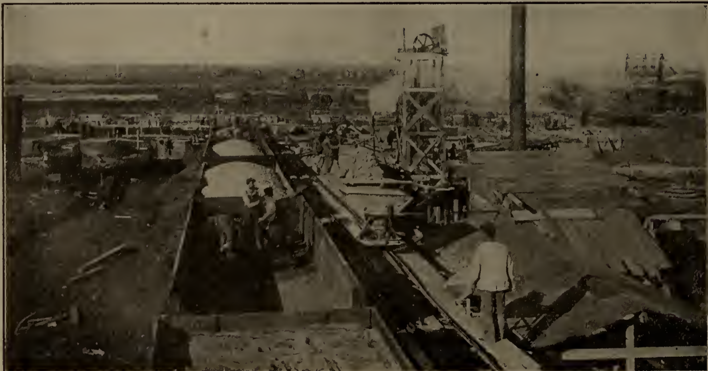
View of Concrete Mixing for B. &amp; M. Shops.
