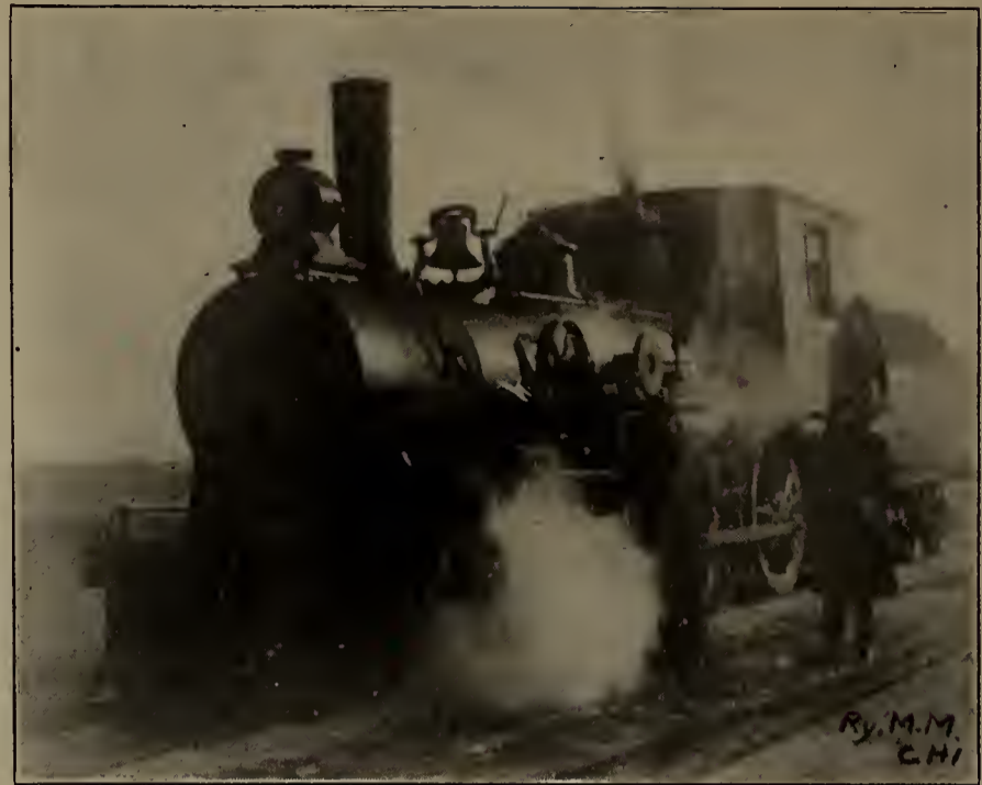
Locomotive Equipped with Doyle's Combustion Apparatus.
