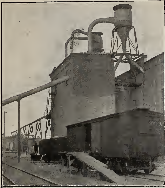
FIG. 22—VIEW OF SHAVING COLLECTOR ON POWER HOUSE C. P. R. SHOPS.
