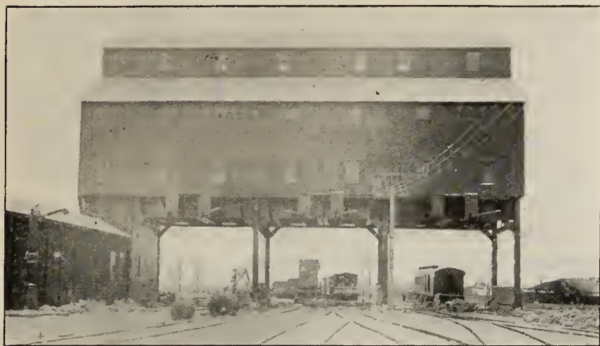
FIG. 6—COALING STATION AND SAND HOUSE, ELKHART ROUNDHOUSE.
