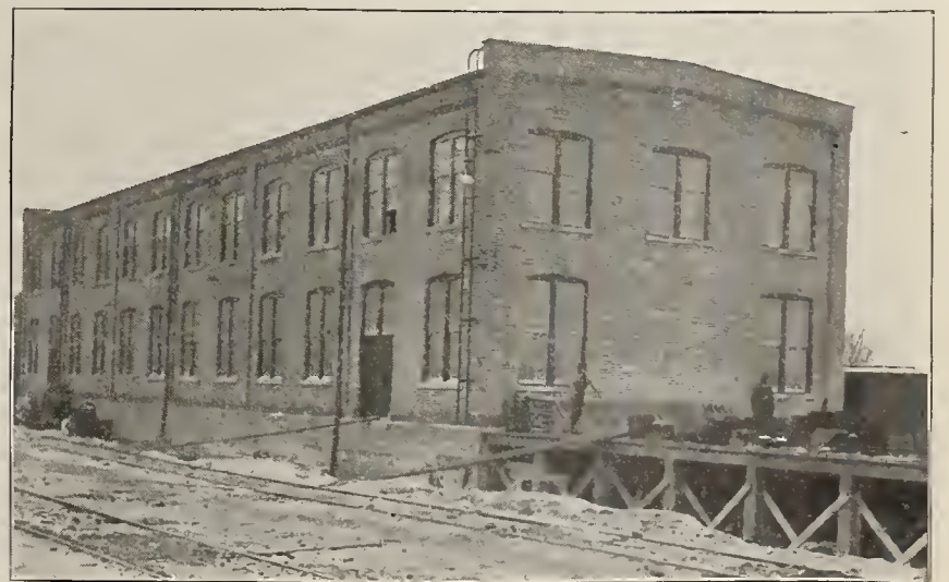
FIG. 3—VIEW OF STOREHOUSE, PERE MARQUETTE SHOPS AT GRAND RAPIDS.
