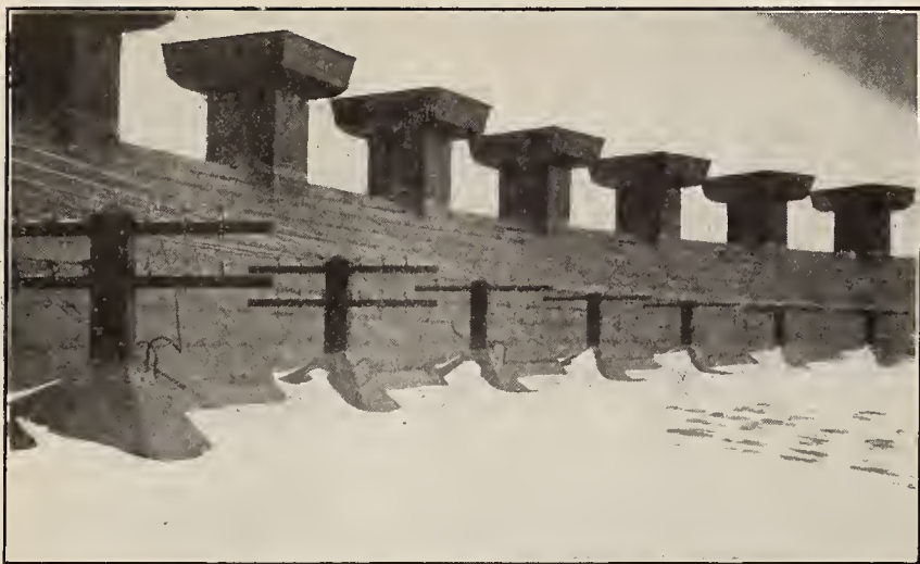
FIG. 11—VIEW OF WIRING AND SMOKE JACKS ON ROOF ELKHART ROUNDHOUSE.
