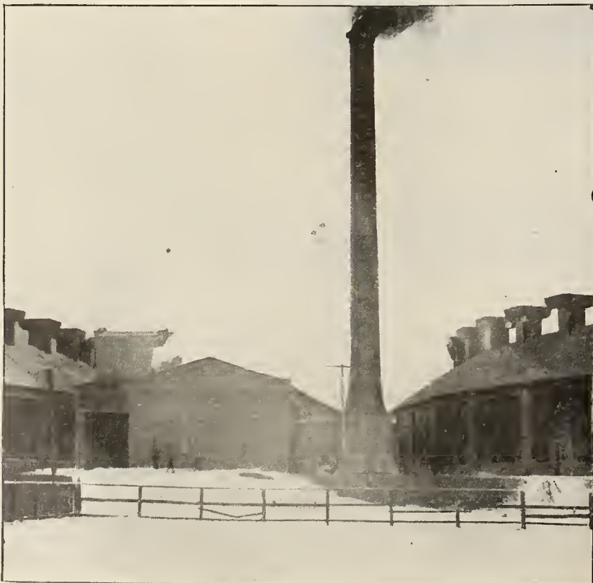
FIG. 4—VIEW OF POWER HOUSE AT ELKHART ROUNDHOUSE.
