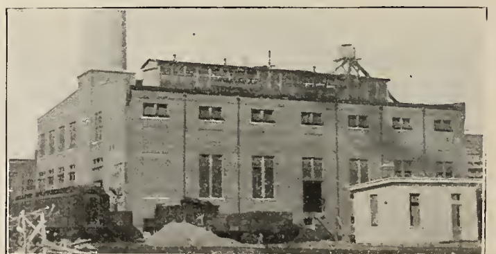
POWERHOUSE—L. & N. SHOPS AT SOUTH LOUISVILLE
