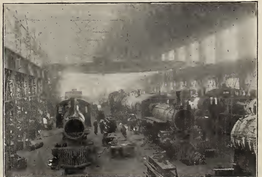
FIG. 2—VIEW IN THE ERECTING SHOP, CANADIAN PACIFIC SHOPS.
