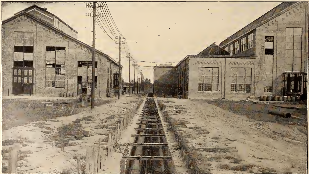
FIG. 18—VIEW BETWEEN BLACKSMITH AND MACHINE SHOPS, SHOWING PORTION OF EACH BUILDING, LINE OF POSTS CARRYING WIRES FOR ELECTRICAL DISTRIBUTION AND TUNNEL FOR STEAM AND AIR MAINS—C & E I. R. R.
