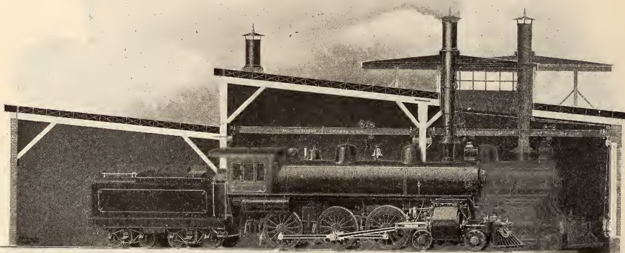
SHOWING CRANE IN ROUNDHOUSE WITH ADJUSTABLE SMOKE JACK.
