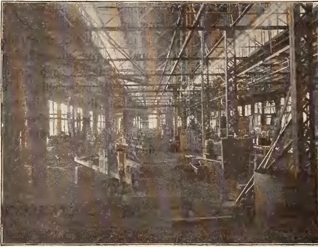
FIG. 4—INTERIOR OF NEW BLACKSMITH SHOP—SCHENECTADY WORKS OF THE AMERICAN LOCOMOTIVE COMPANY.
