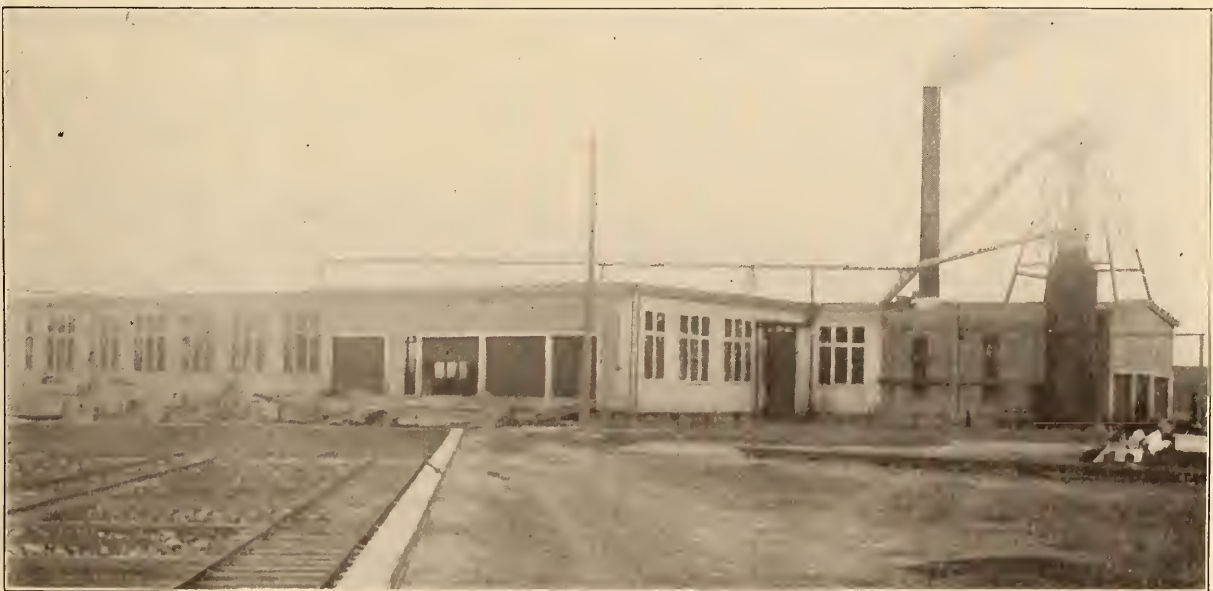
FIG. 3—MILL BUILDING, POWER HOUSE ANNEX BEING SHOWN AT RIGHT.
