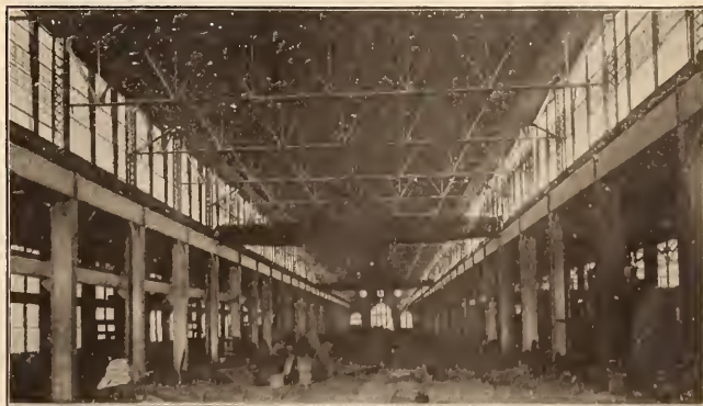
FIG. 3—SHOWING STRUCTURAL WORK OF NEW FOUNDRY—SCHENECTADY WORKS OF THE AMERICAN LOCOMOTIVE COMPANY.
