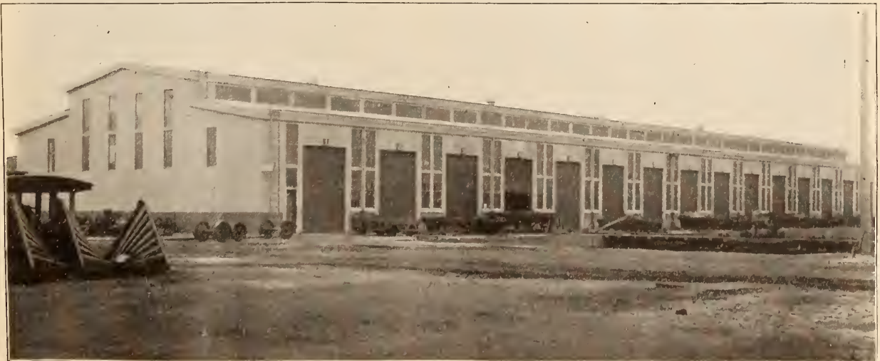
FIG. 6—COACH REPAIR AND PAINT SHOP—TRANSFER TABLE IS SHOWN IN FOREGROUND.
