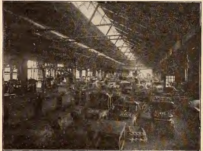
FIG. 6—INTERIOR OF NEW CYLINDER SHOP—SCHENECTADY WORKS OF THE AMERICAN LOCOMOTIVE CO.
