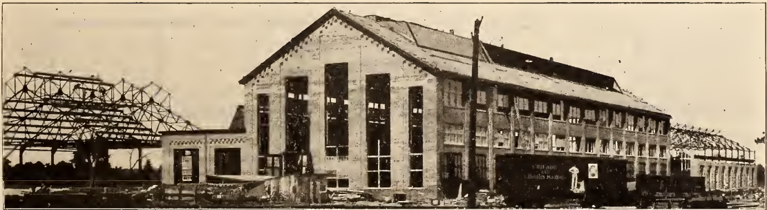
FIG. 11—GENERAL VIEW OF BLACKSMITH, MACHINE AND BOILER SHOPS DURING ERECTION—C. & E. I. R. R.
