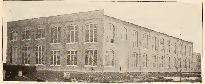
FIG. 2—EXTERIOR VIEW OF LOCOMOTIVE AND MACHINE SHOP—TERMINAL R. R. OF ST. L.
