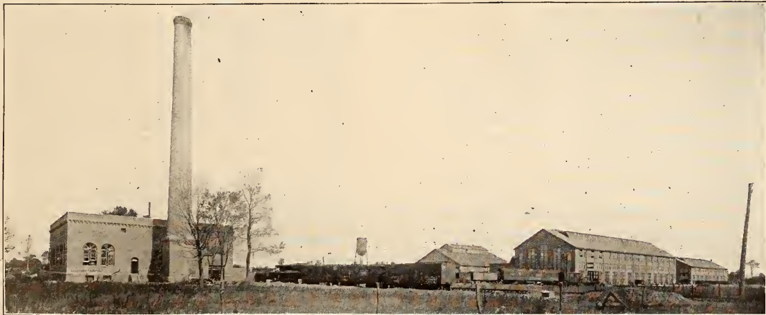
FIG. 1—VIEW SHOWING LOCATION OF POWER HOUSE WITH RELATION TO OTHER BUILDINGS OF PLANT. LARGE BUILDING AT RIGHT IS MACHINE AND ERECTING SHOP—C. & E. I. R. R.
