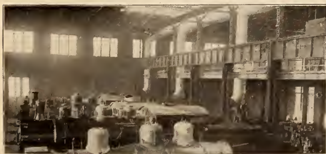
FIG. 7—SHOWING DISTRIBUTION OF HOT AIR DISCHARGE PIPES IN LOCOMOTIVE AND MACHINE SHOP—TERMINAL R. R. OF ST. L.
