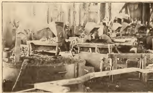
FORGES EQUIPPED WITH DOWN DRAFT HOODS, BRAINERD, MINN., BLACKSMITH SHOP, N. P. RY.
