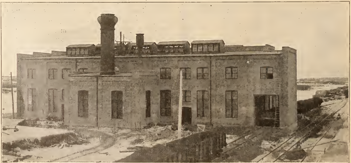
FIG. 1.—POWER HOUSE OF THE NEW SHOPS OF THE ROCK ISLAND SYSTEM AT EAST MOLINE, ILL.
