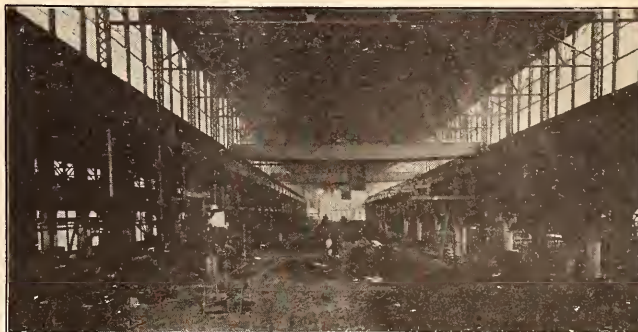
FIG. 2—CENTRE BAY OF NEW BOILER SHOP—SCHENECTADY WORKS OF THE AMERICAN LOCOMOTIVE CO.
