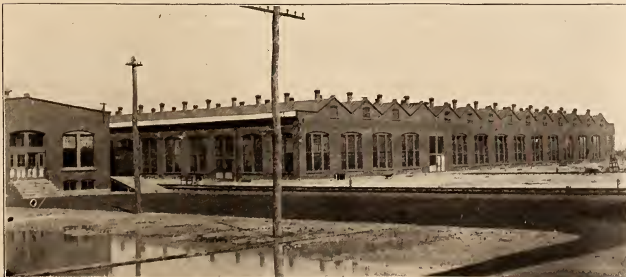
PAINT SHOP AND FRONT OF PAINT STORAGE, P., B. & W. RAILROAD.
