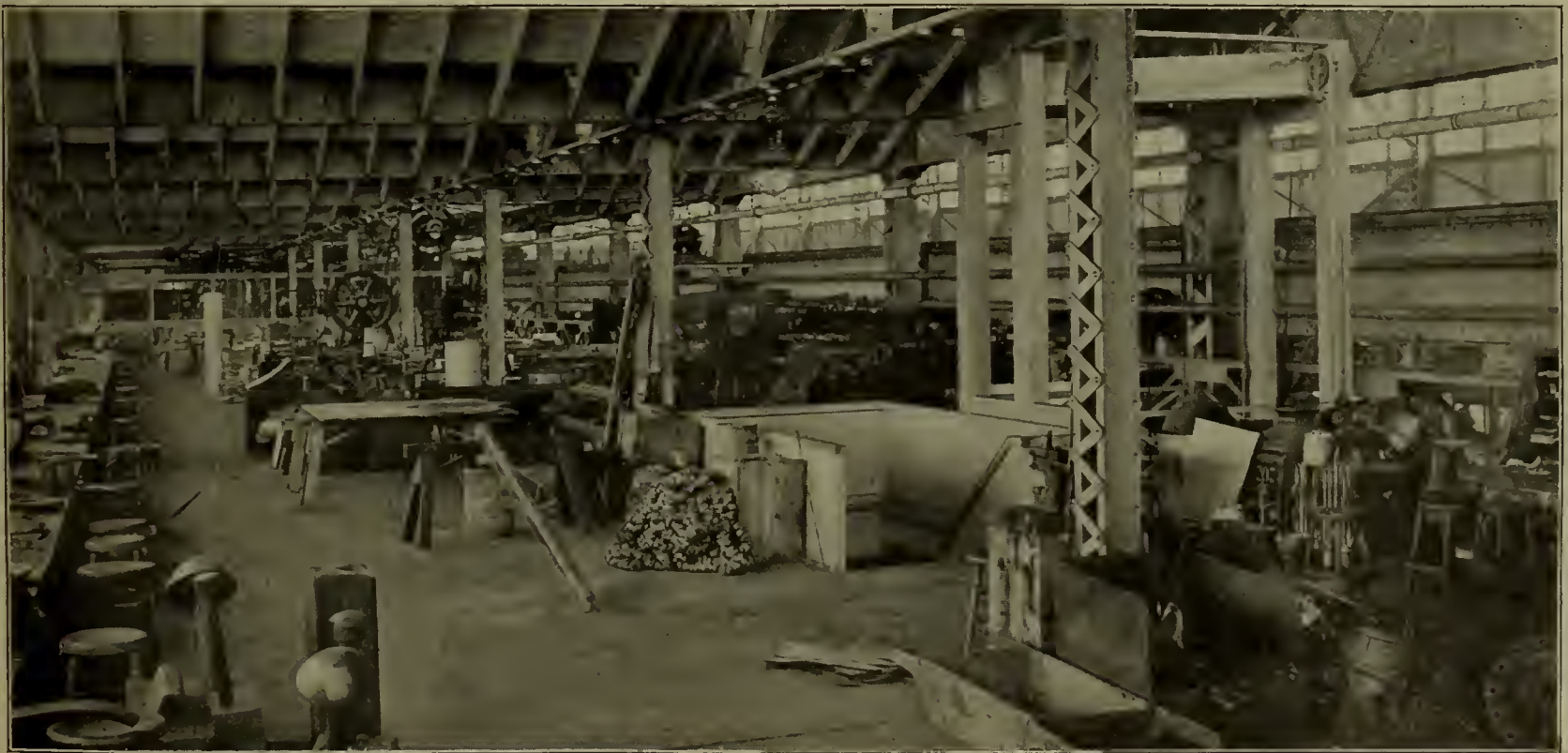
FIG. 10—TOPEKA SHOPS OF THE ATCHISON, TOPEKA & SANTA FE RAILWAY—TIN SHOP LOCATED IN BALCONY OF LOCOMOTIVE SHOP.
