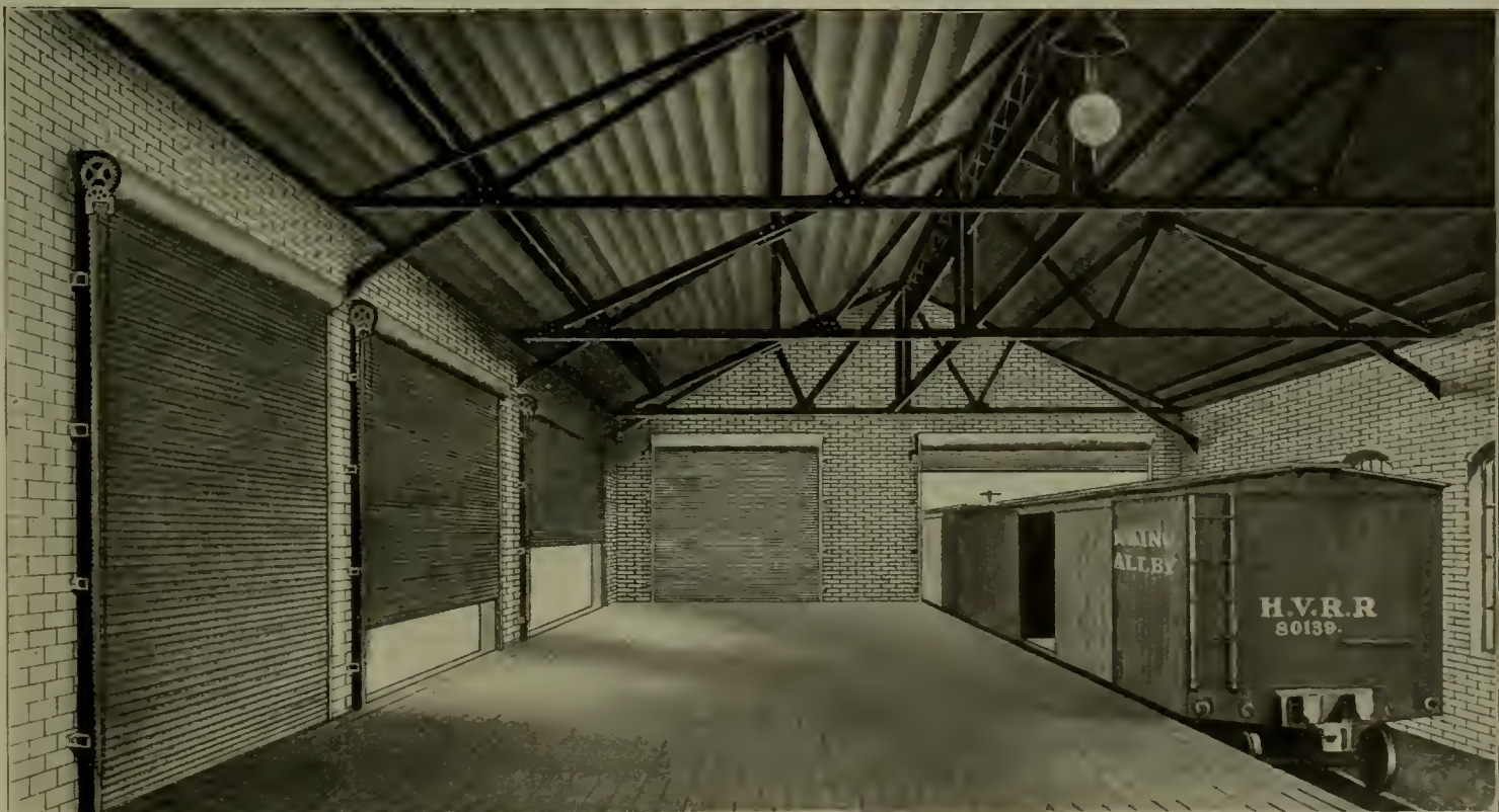
FIG. 5—APPLICATION OF ROLLING SHUTTERS TO HOCKING VALLEY FREIGHT HOUSE.
