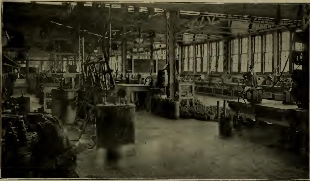
FIG. 5—TOPEKA SHOPS OF THE ATCHISON, TOPEKA & SANTA FE RAILWAY—AIR BRAKE REPAIR ROOM LOCATED IN BALCONY.
