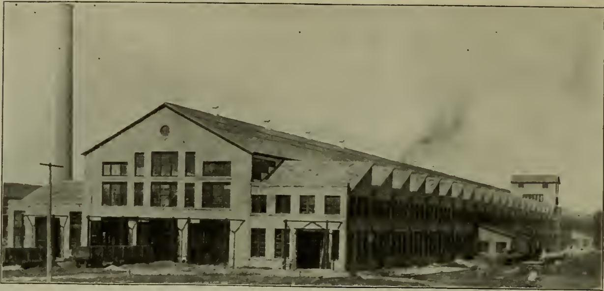
FIG. 4—TOPEKA SHOPS OF THE ATCHISON, TOPEKA & SANTA FE RAILWAY. LOCOMOTIVE AND BOILER SHOP. SHOWING SAW TOOTH ARRANGEMENT OF ROOF, RIVETING TOWER AND FAN HOUSES.
