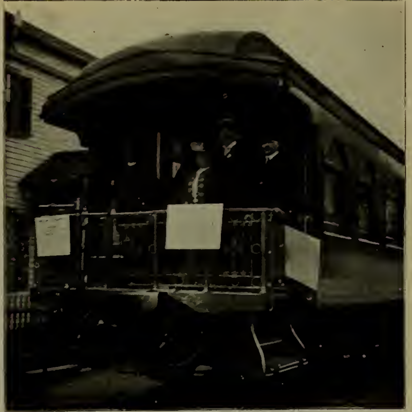
COL. DICKINSON AND HIS PARTY ON THE CAR ON WHICH PRESIDENT ROOSEVELT RODE 15,000 MILES. THIS CAR IS EQUIPPED WITH THE AXLE LIGHTING SYSTEM OF THE CONSOLIDATED RY. ELECTRIC LIGHTING AND EQUIPMENT CO.
