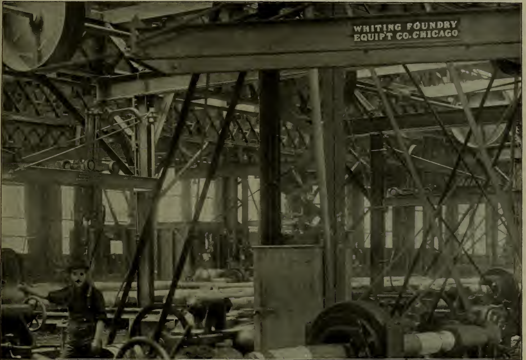
FIG. 3—TWENTY-SIX AIR HOIST BRACKET JIB CRANES, FOR HOWARD AXLE WORKS, CARNEGIE STEEL CO., HOMESTEAD, PA.
