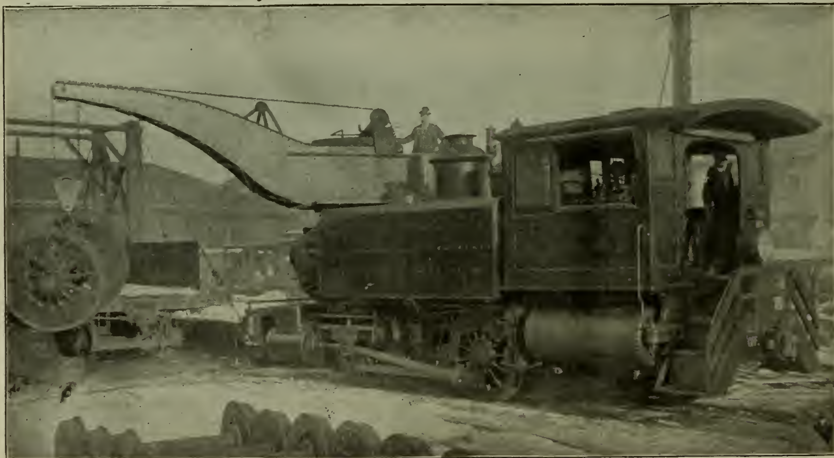
VIEW OF ATCHISON, TOPEKA & SANTA FE RY. LOCOMOTIVE CRANE IN OPERATION.
