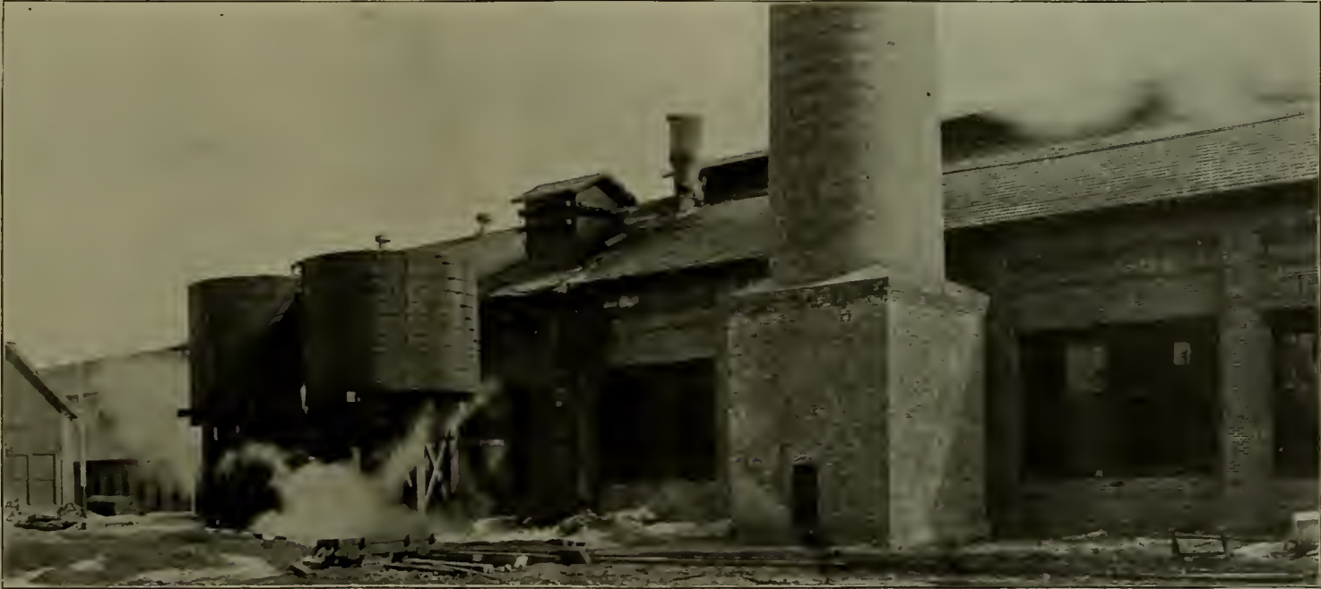
FIG. 6. TOPEKA SHOPS OF THE ATCHISON, TOPEKA & SANTA FE RAILWAY. POWER HOUSE—SHOWING BASE OF STACK, PURIFYING TANKS AND WIRE DISTRIBUTING TOWER.
