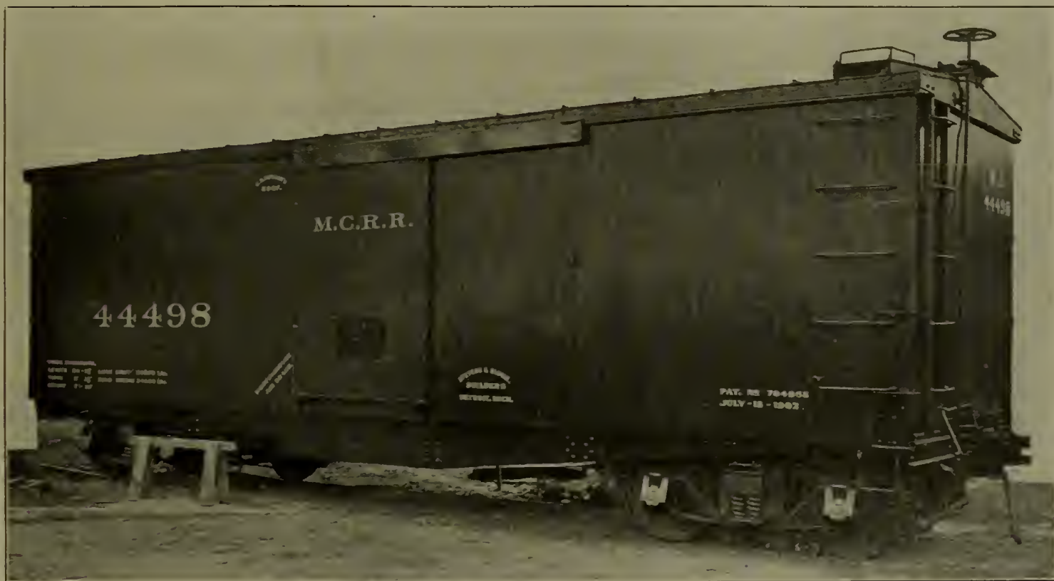
STEEL FRAME BOX CAR—FINISHED.
