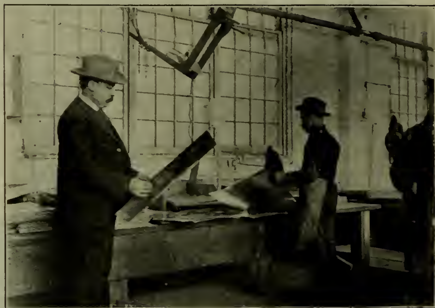
INSPECTING TERNE PLATES AT LAUGHLIN WORKS, AMERICAN TIN PLATE CO.
