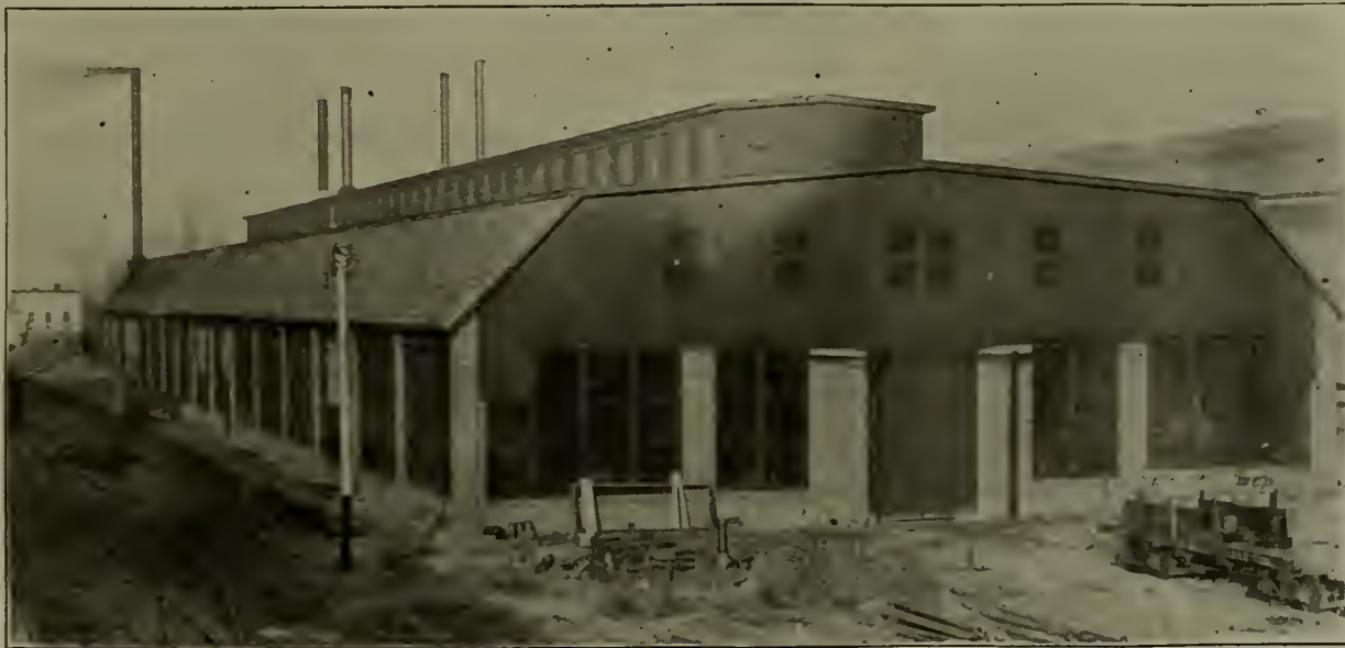
FIG. 3—TOPEKA SHOPS OF THE ATCHISON, TOPEKA & SANTA FE RAILWAY. BLACKSMITH SHOP.
