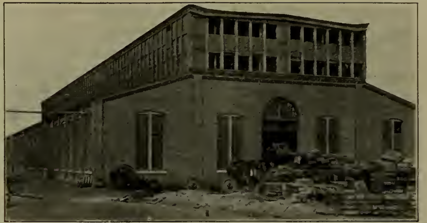
FIG. 5—EXTERIOR OF NEW CYLINDER SHOP, BROOKS WORKS OF THE AMERICAN LOCOMOTIVE CO.
