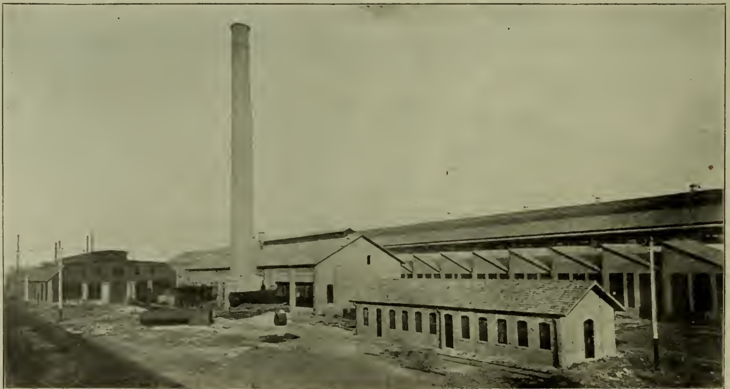
FIG. 5. TOPEKA SHOPS OF THE ATCHISON, TOPEKA & SANTA FE RAILWAY. SHOWING GENERAL ARRANGEMENT OF NEW BUILDINGS. BLACKSMITH SHOP AT EXTREME LEFT, POWER HOUSE NEAR CENTER, LAVATORY IN FOREGROUND AND LOCOMOTIVE AND BOILER SHOP IN BACKGROUND.
