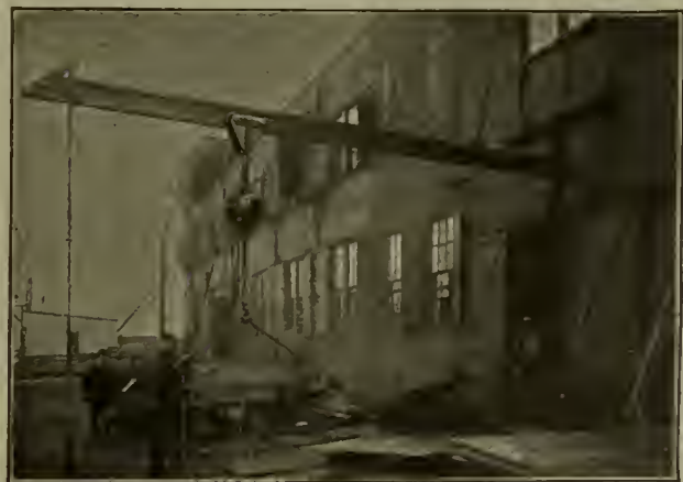
DELIVERING FINISHED MATERIAL ON OVERHEAD TROLLEY IN BRIDGE WORKS.
