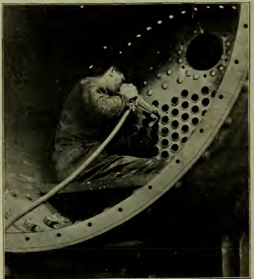
FIG. 7—Q. & C. PNEUMATIC HAMMER IN SERVICE BEADING FLUES.
