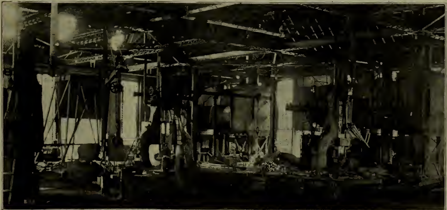
FIG. 6—TOPEKA SHOPS OF THE ATCHISON, TOPEKA & SANTA FE RAILWAY—INTERIOR OF BLACKSMITH SHOP, SHOWING LOCATION OF STEAM HAMMERS AND STEAM GENERATING FURNACES.
