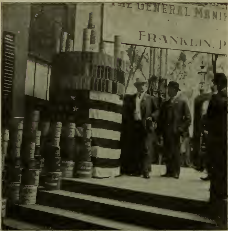
G. B. COFFIN AND HEATH & MILLIGAN EXHIBIT, AND IN THE BACKGROUND THE EXHIBIT OF THE GENERAL MANIFOLD CO., WHOSE SIGN SHOWS UP IN THE UPPER RIGHT HAND CORNER OF THE PICTURE.
