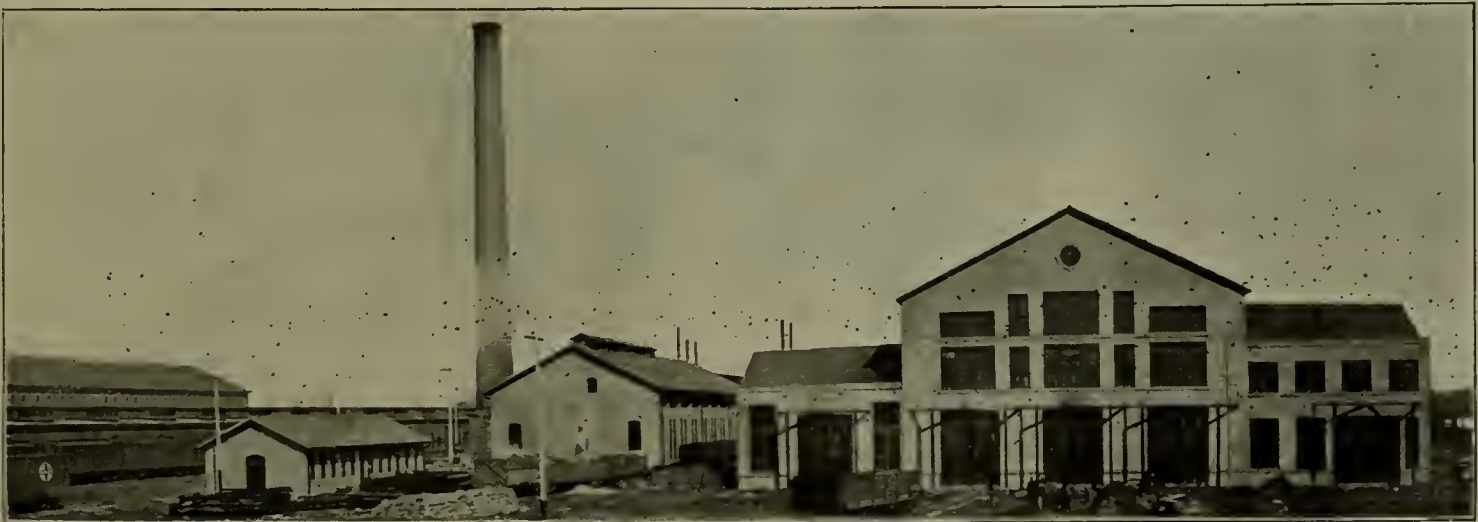
FIG. 2—TOPEKA SHOPS OF THE ATCHISON, TOPEKA & SANTA FE RAILWAY. VIEW LOOKING NORTH. LOCOMOTIVE AND BOILER SHOP TO RIGHT, PORTION OF CAR SHOP AT EXTREME LEFT, POWER HOUSE AND LAVATORY BETWEEN.
