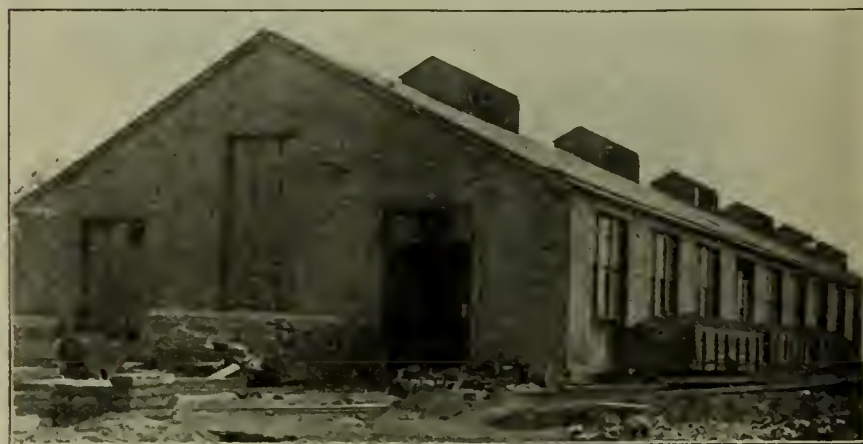
FIG. 2—EXTERIOR OF NEW HAMMER SHOP, BROOKS WORKS OF THE AMERICAN LOCOMOTIVE CO.
