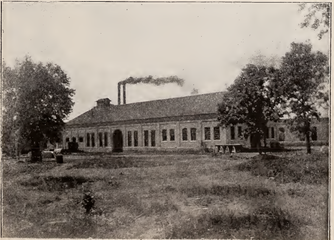
MACHINE SHOP, STOREHOUSE AND BOILER ROOM.
