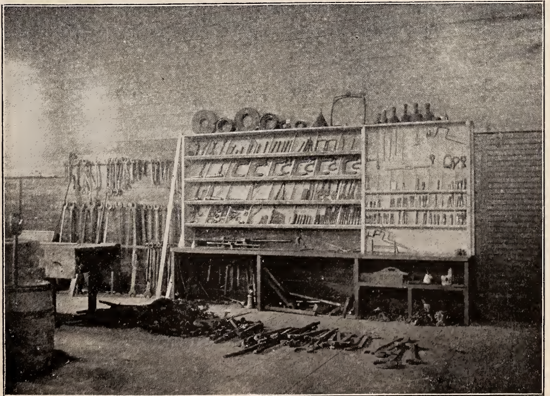
TOOL ROOM IN STOREHOUSE.
