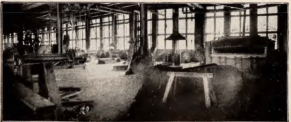
IN THE BOILER SHOP—THE ANNEALING FURNACE CORNER.
