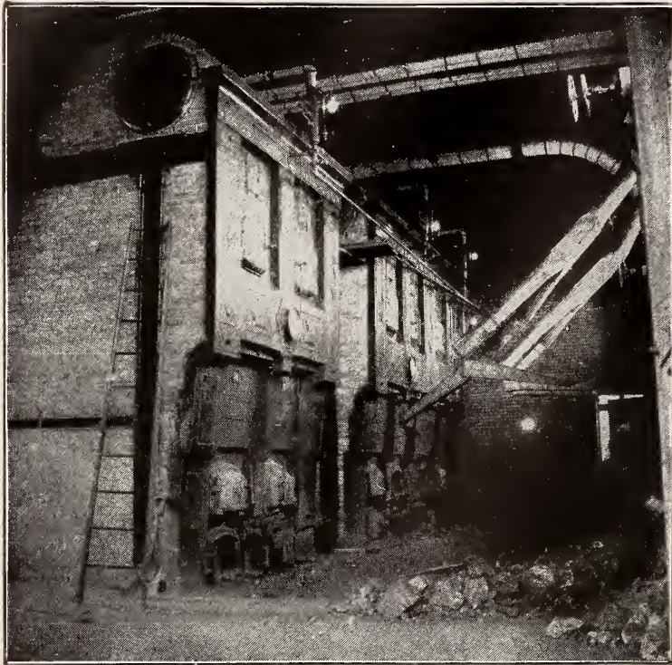
THE BOILER ROOM.
