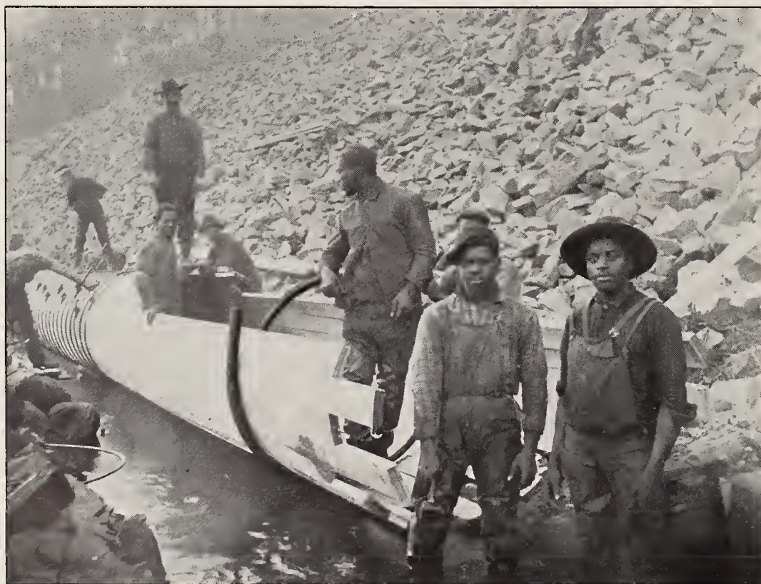
THE U-FORMED CRADLE AND INNER SUPPORTING RING FOR SETTING UP THE PIPE ARE HERE MORE CLEARLY SHOWN. FOR DESCRIPTION, SEE OPPOSITE PAGE
