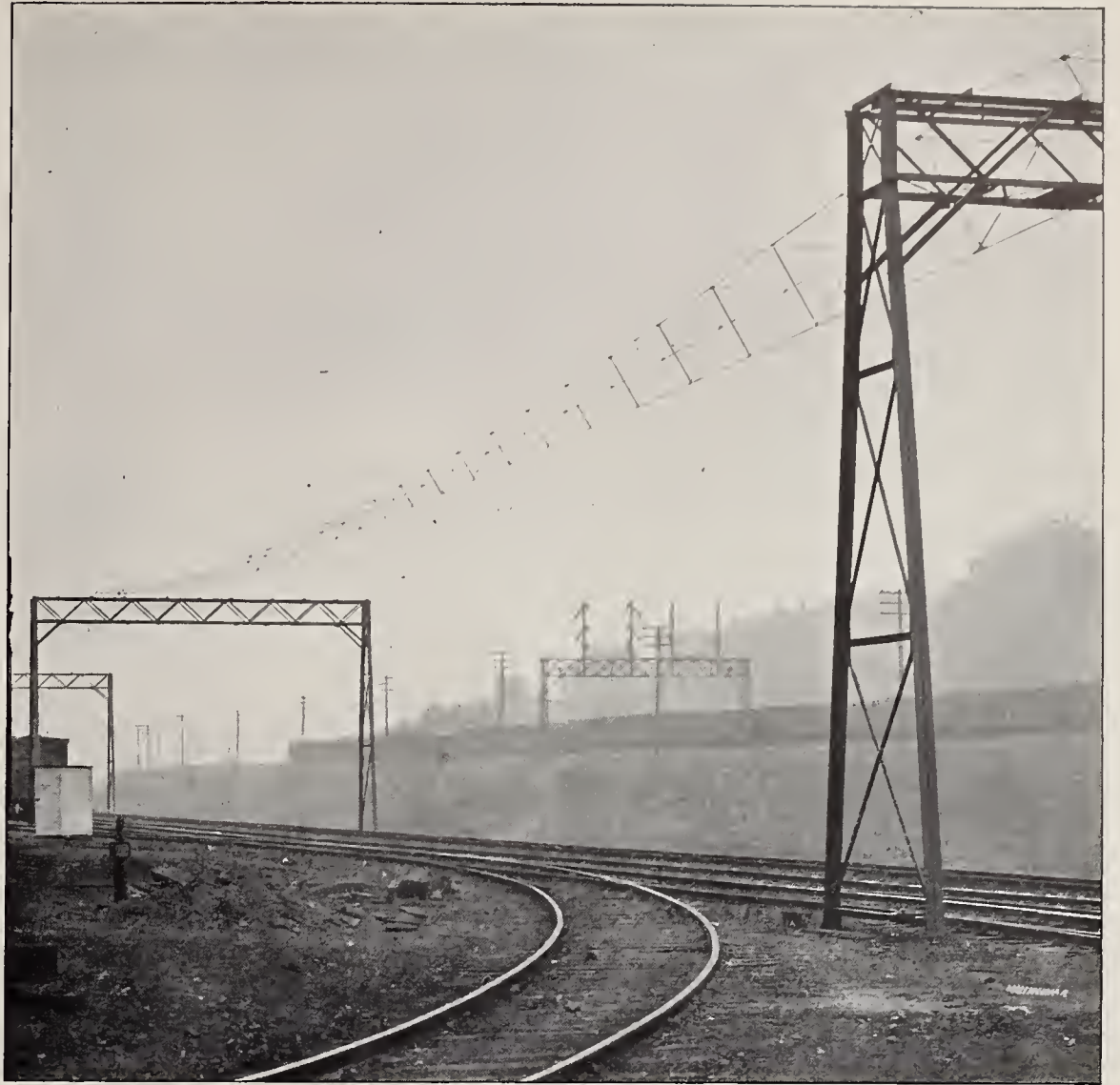
FIG. 9.—DOUBLE-CATENARY LINE CONSTRUCTION, WITH BRIDGE SUPPORTS
