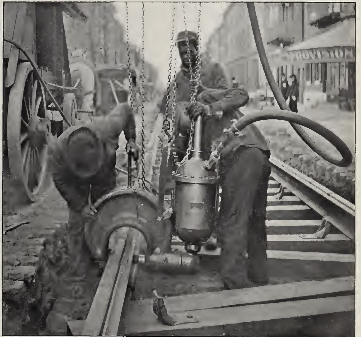
A HYDRO-PNEUMATIC RIVETING MACHINE ON TRACK WORK
