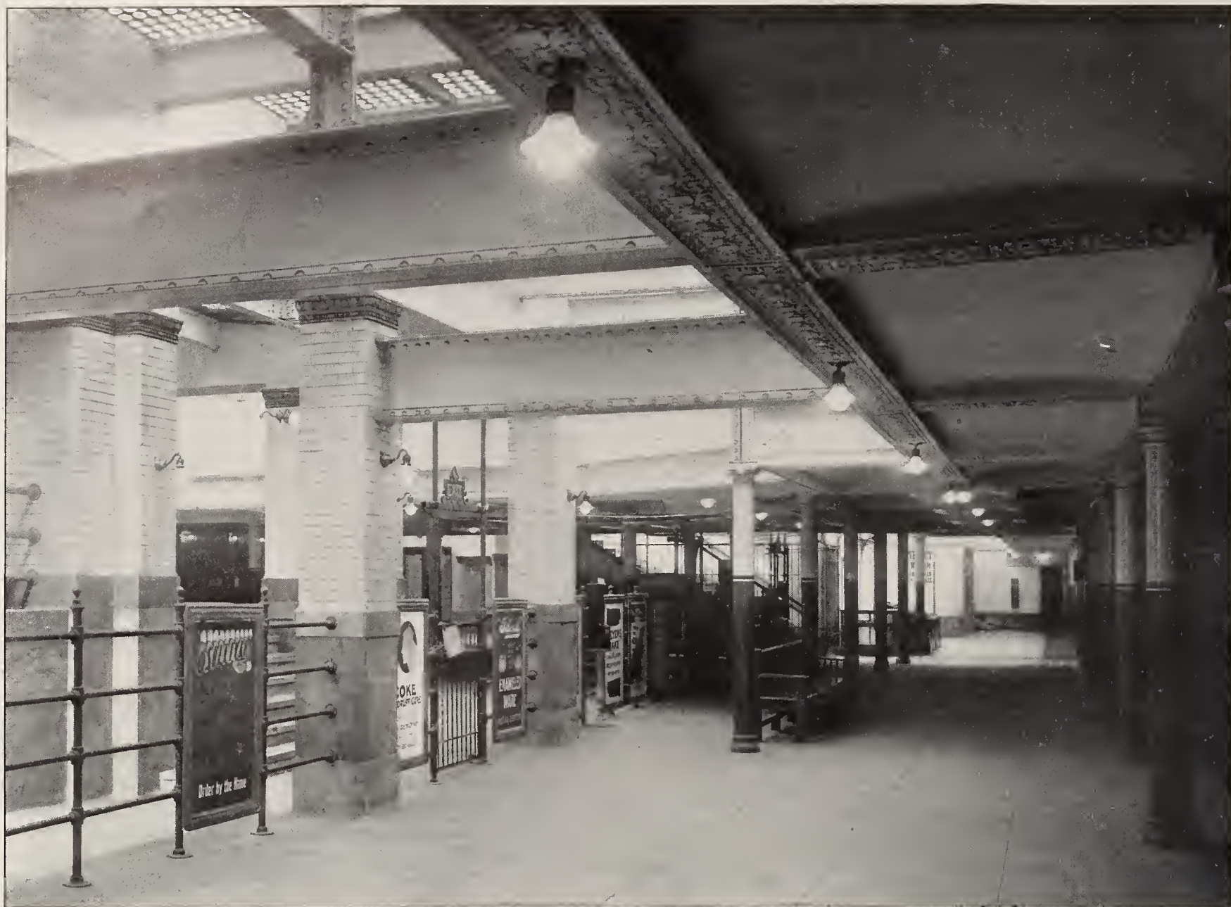
FIG. 2.—A SUBWAY STATION SHOWING ARRANGEMENT OF LAMPS FITTED WITH BELL-SHAPED PRISMATIC GLASS REFLECTORS AND ENCLOSED IN FROSTED GLASS BALLS
