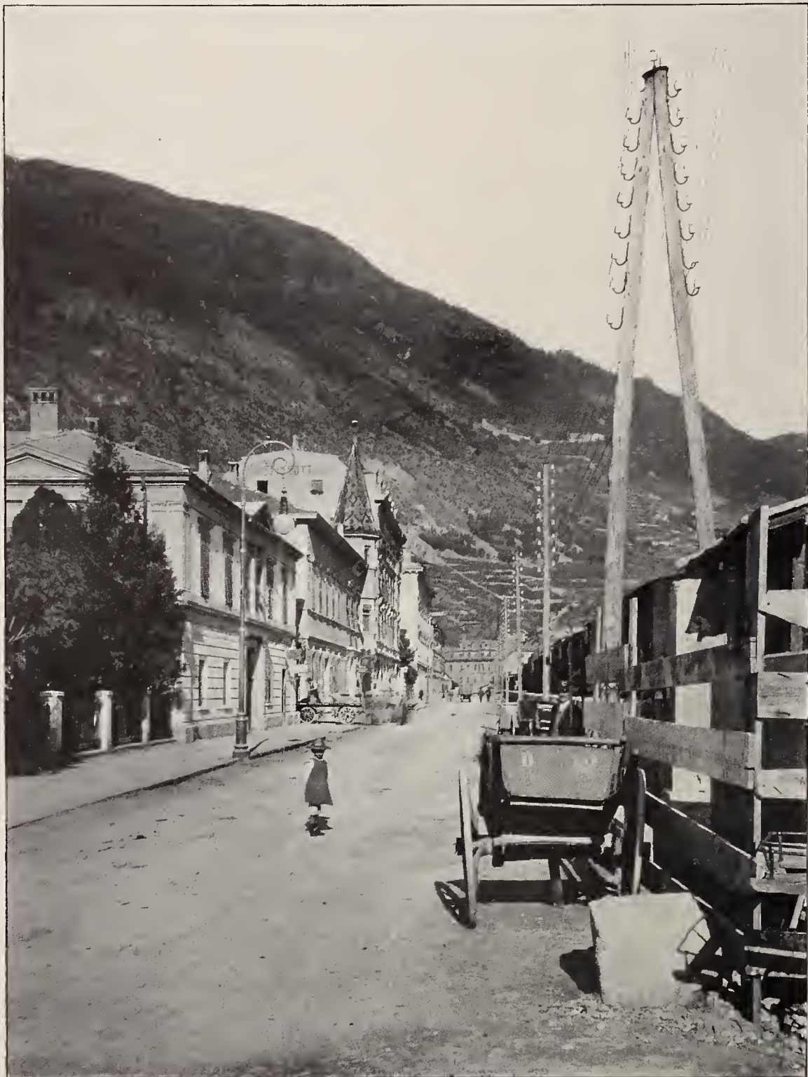
A VIEW OF THE OVERHEAD TRANSMISSION LINES
