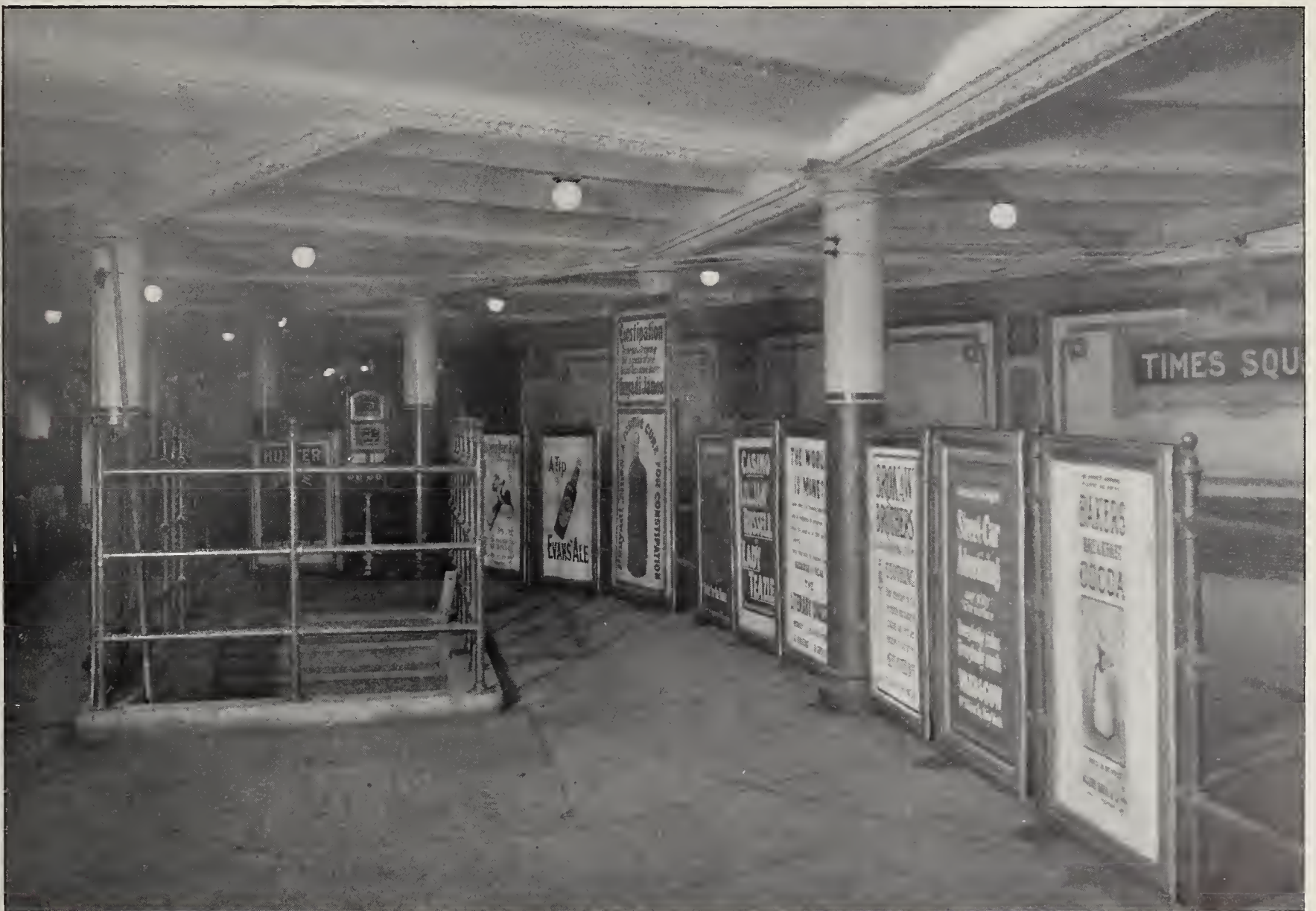
FIG. I.—A SUBWAY STATION SHOWING ARRANGEMENT OF LAMPS ENCLOSED IN FROSTED GLASS BALLS
