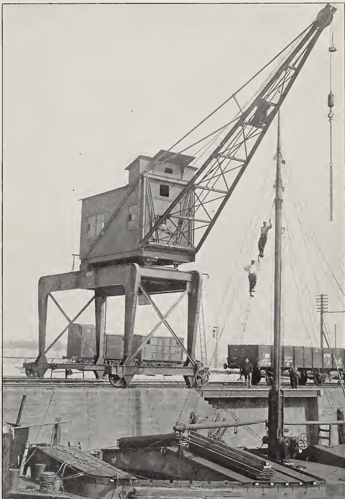
FIG. 1.—A 5-TON GANTRY CRANE AT LUDWIGSHAFEN, GERMANY, EQUIPPED WITH POLYPHASE MOTORS BY MESSRS. BROWN, BOVERI & CO., BADEN, SWITZERLAND
