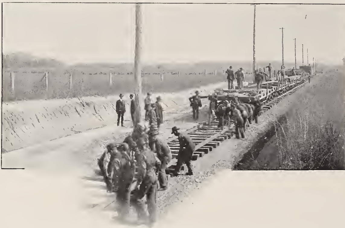
TRACK LAYING ON THE INDIANAPOLIS & CINCINNATI SINGLE-PHASE RAILWAY
