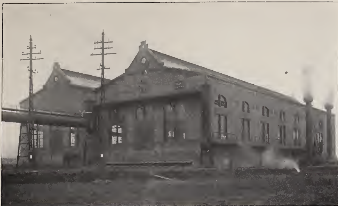
THE GAS FROM THE BLAST FURNACE ARRIVES THROUGH THE LARGE MAINS HERE SHOWN
