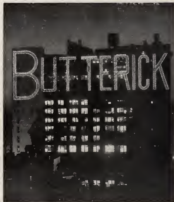
ELECTRIC SIGN CONTAINING 1152 EDISON LAMPS INSTALLED ON THE BUTTERICK BUILDING, NEW YORK CITY
