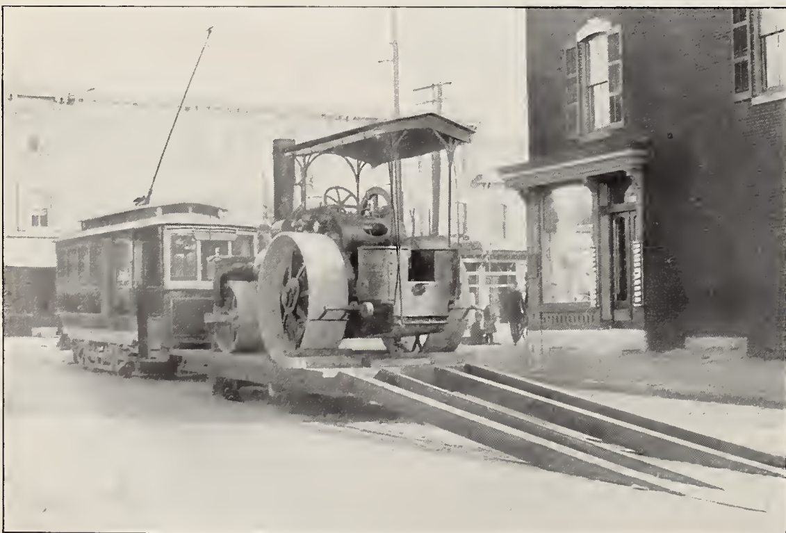
TRANSFERRING THE ROLLER TO THE STREET LEVEL. SEE PAGE 8
