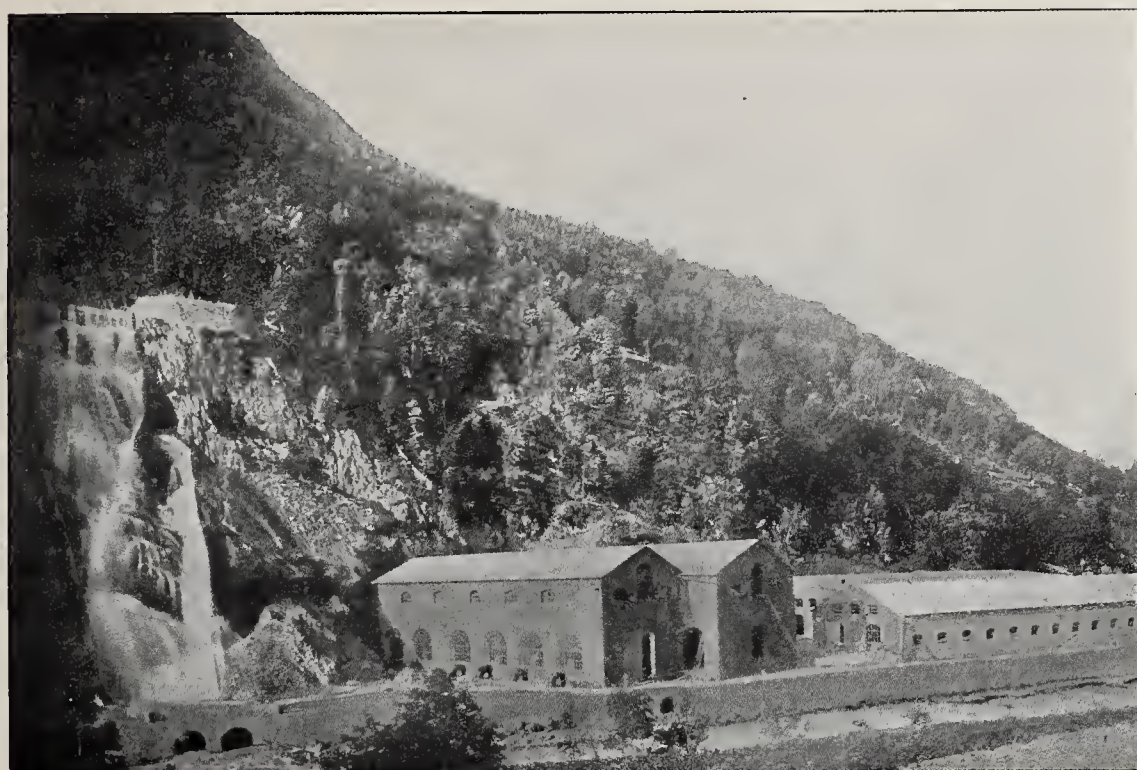
THE STEEL WORKS AT LIVET, FRANCE, OF THE THERMO-ELECTRIC COMPANY, OF PARIS. WATER POWER DEVELOPS THE ELECTRIC CURRENT HERE USED
