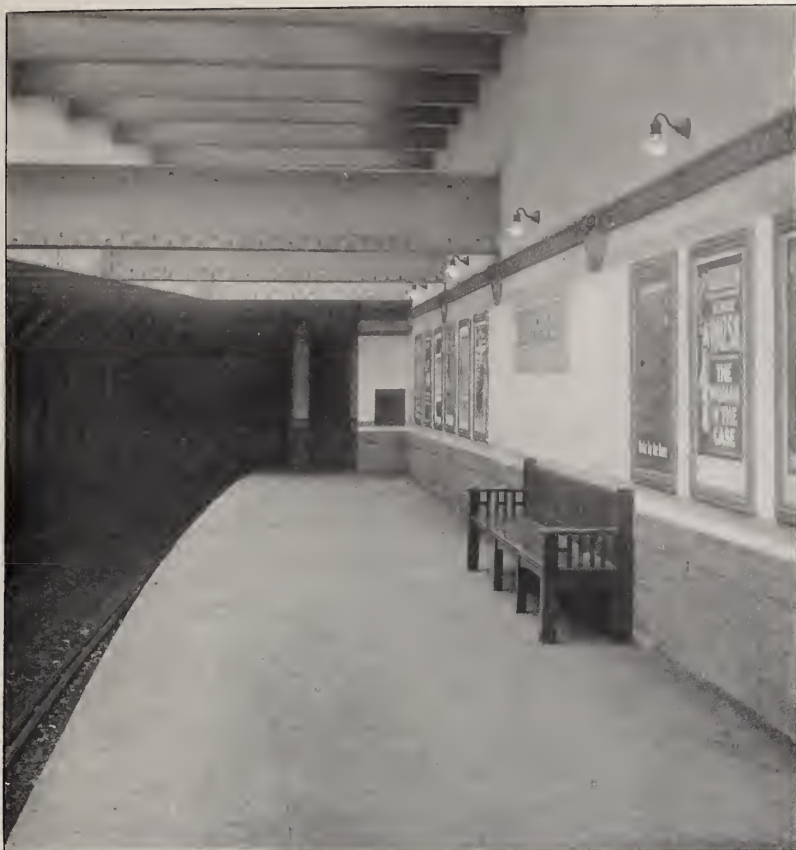
FIG. 7.—A SUBWAY STATION SHOWING A CURVED PLATFORM, BELOW WHICH LAMPS ARE PLACED TO LIGHT UP THE OPENING BETWEEN ITS OUTER EDGE AND THE CAR PLATFORMS
