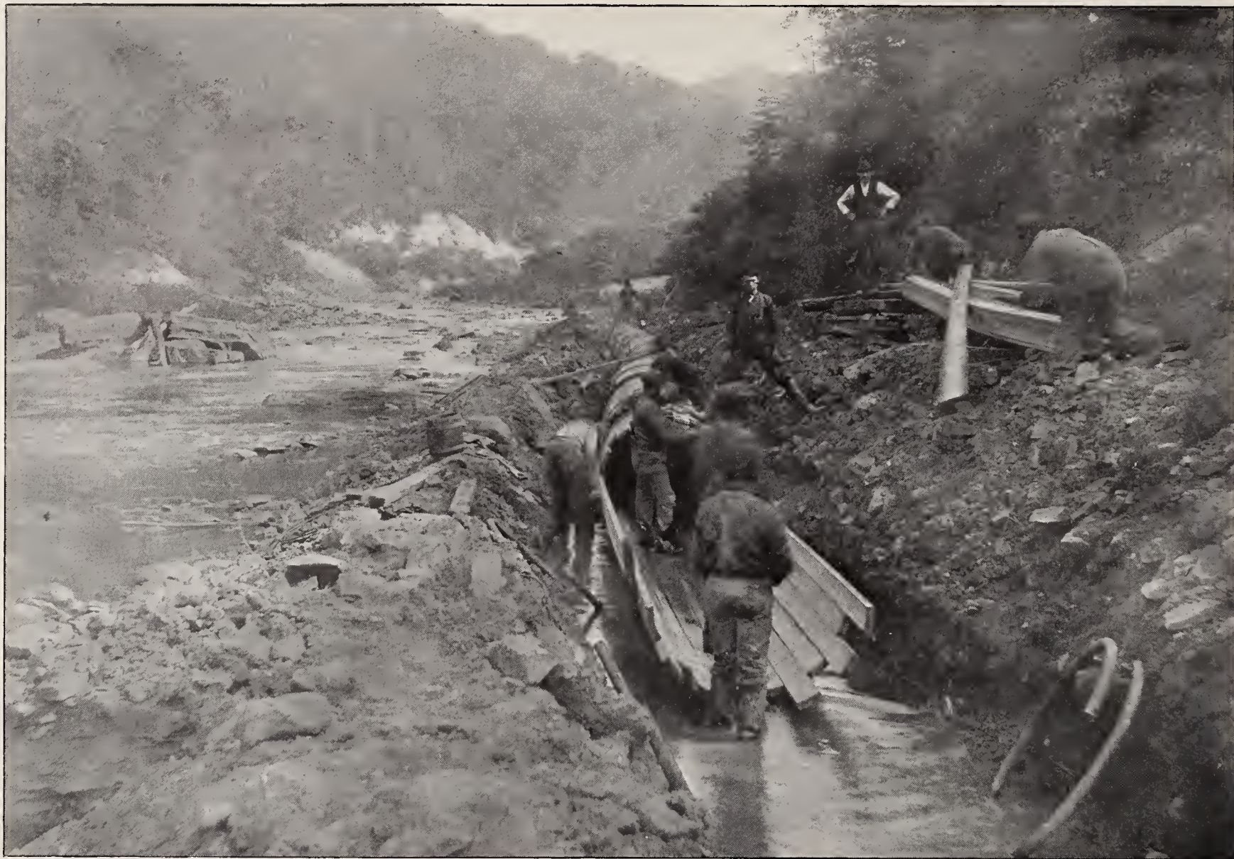
SETTING UP THE JOHNSTOWN PIPE LINE
