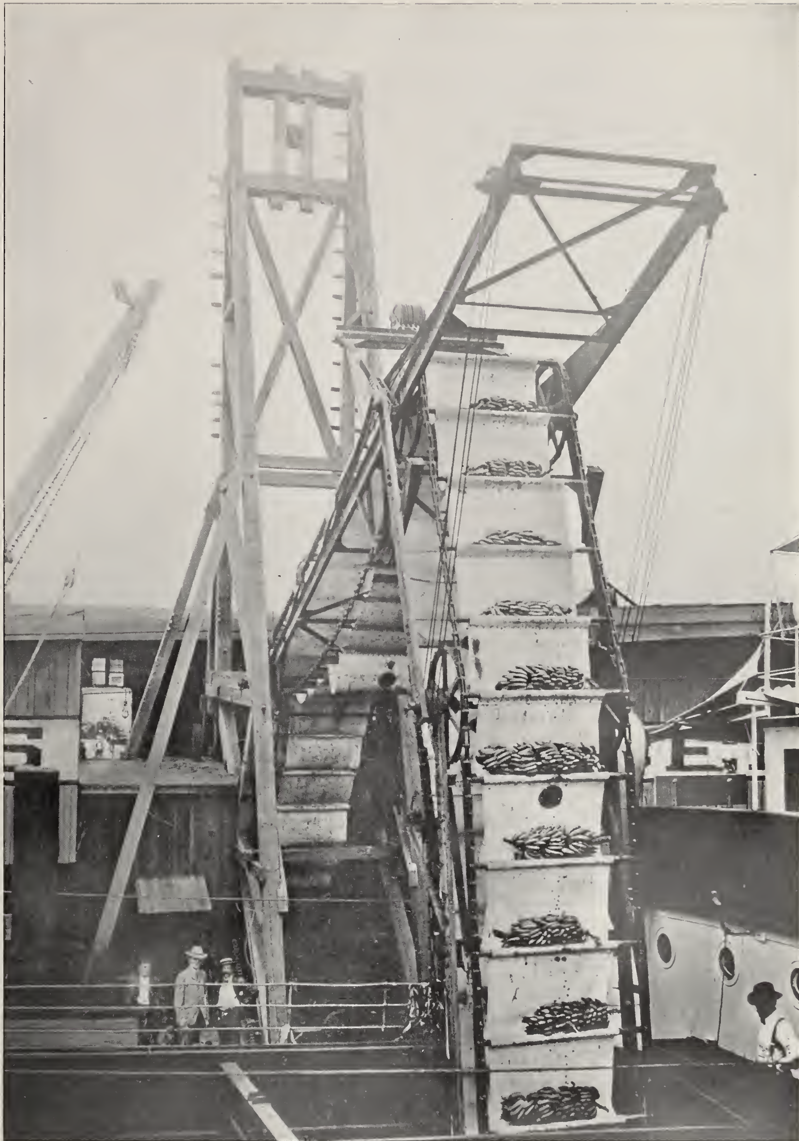
AN ELECTRICALLY DRIVEN BANANA CONVEYOR AT NEW ORLEANS. THE CONVEYOR LEG IS SHOWN EXTENDED FROM THE WHARF INTO THE HOLD OF THE SHIP ALONGSIDE
