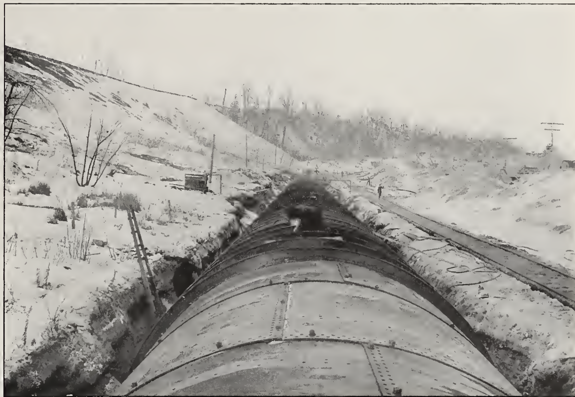
ONE OF THE 18-FOOT CONDUITS OF THE ONTARIO POWER COMPANY, CARRYING WATER FROM THE HEAD WORKS TO THE POWER HOUSE. SEE MAP ON PAGE 401
