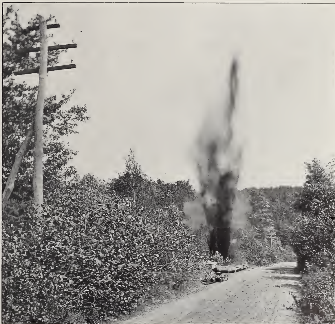
FIG. 1.—BLASTING OUT A POLE HOLE
