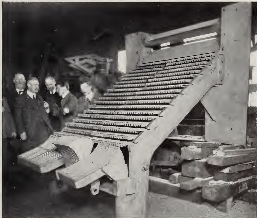
A VIEW OF THE FULTON STEPPED GRATE
