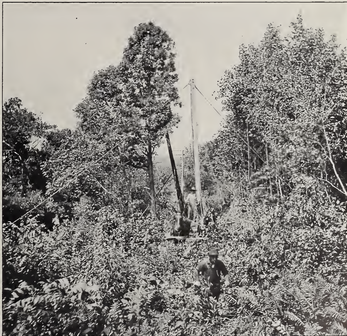
FIG. 6.—THE DERRICK BEING HAULED BETWEEN POLES
