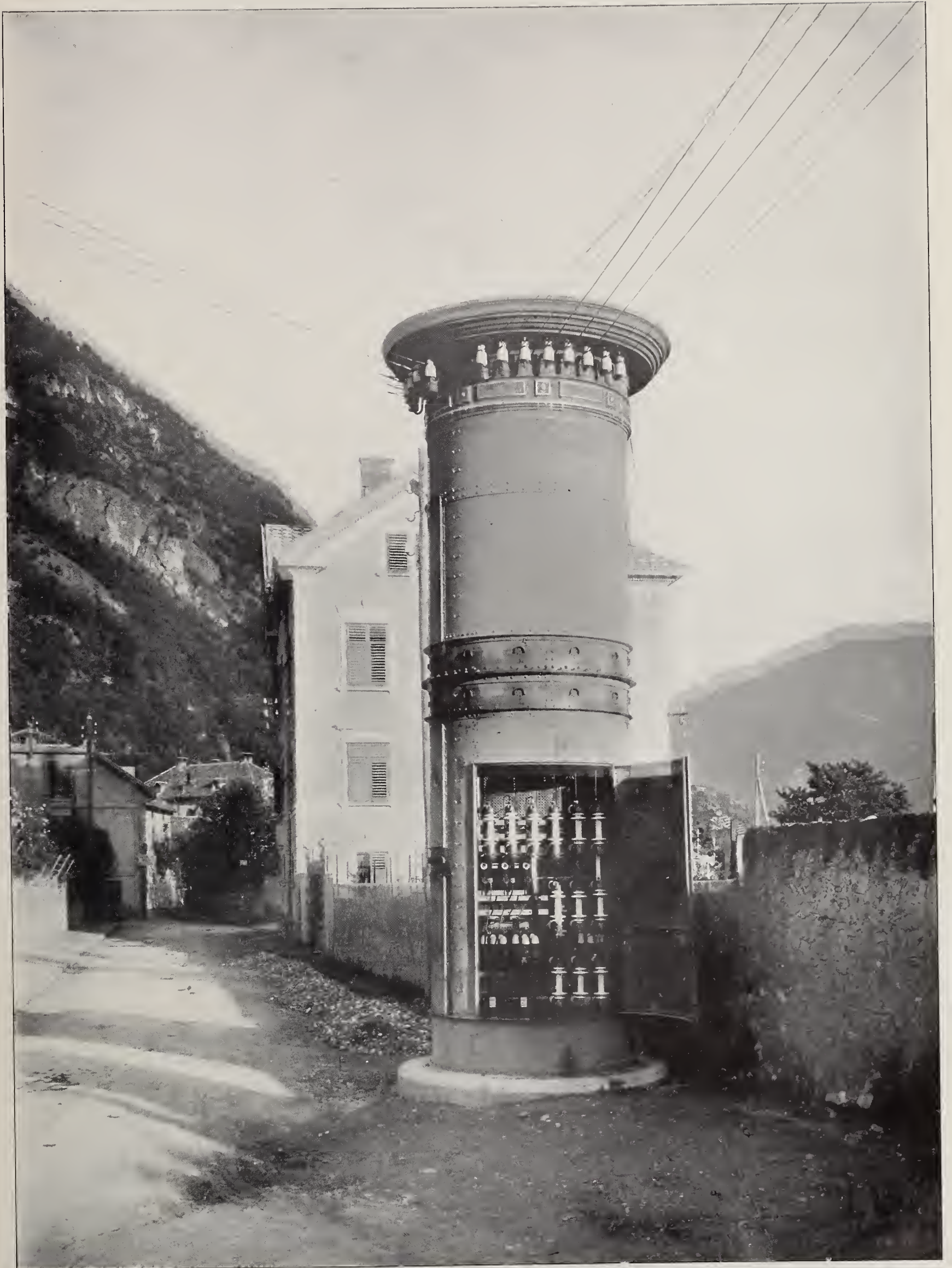
ONE OF THE SHEET-IRON TRANSFORMER TOWERS USED FOR THE OVERHEAD WIRES
