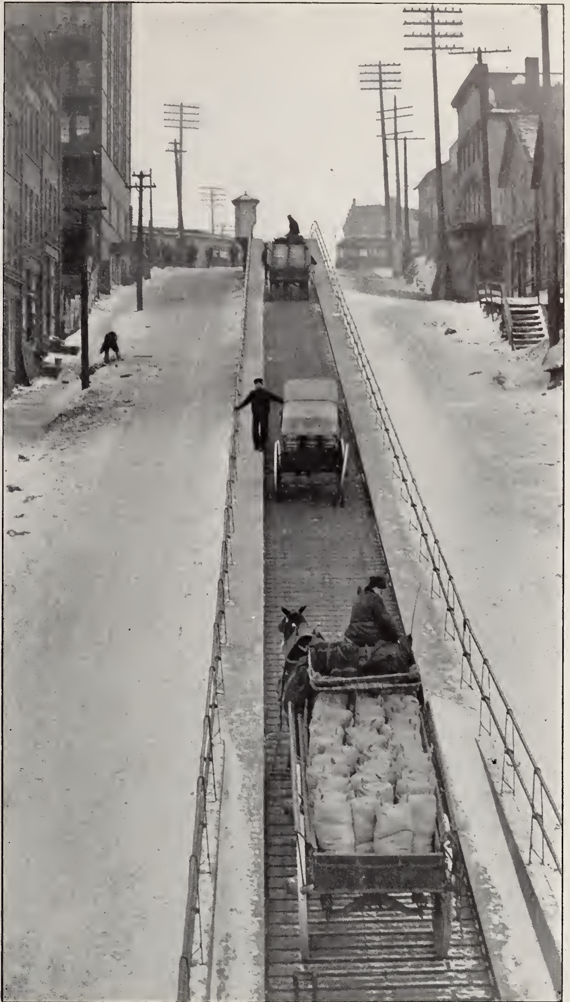
THE "ROLLING ROAD" AVOIDS THE NECESSITY OF A PULL UP A LONG, STEEP HILL. AS MANY AS EIGHT WAGONS MAY BE CARRIED AT ONE TIME
