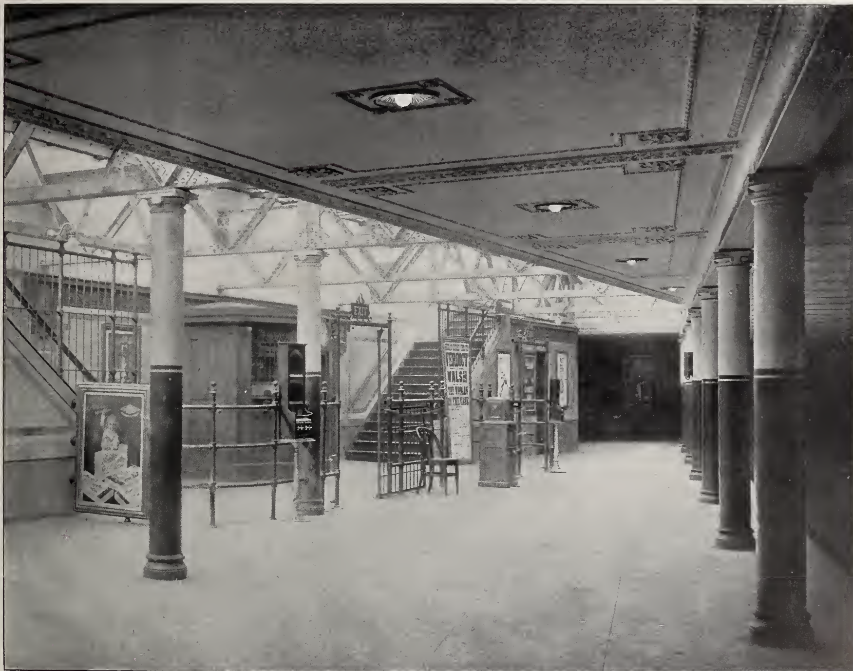
FIG. 3.—A SUBWAY STATION SHOWING ARRANGEMENT OF LAMPS ENCLOSED IN REMOVABLE FROSTED GLASS BALLS, AND PROVIDED WITH FLATTENED PRISMED GLASS REFLECTORS HAVING A WHITE COATING ON THE PRISMED SIDE
