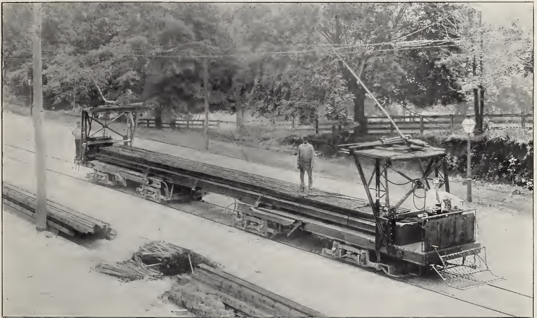
A SPECIAL CAR FOR TRANSPORTING RAILS FOR CONSTRUCTION WORK
