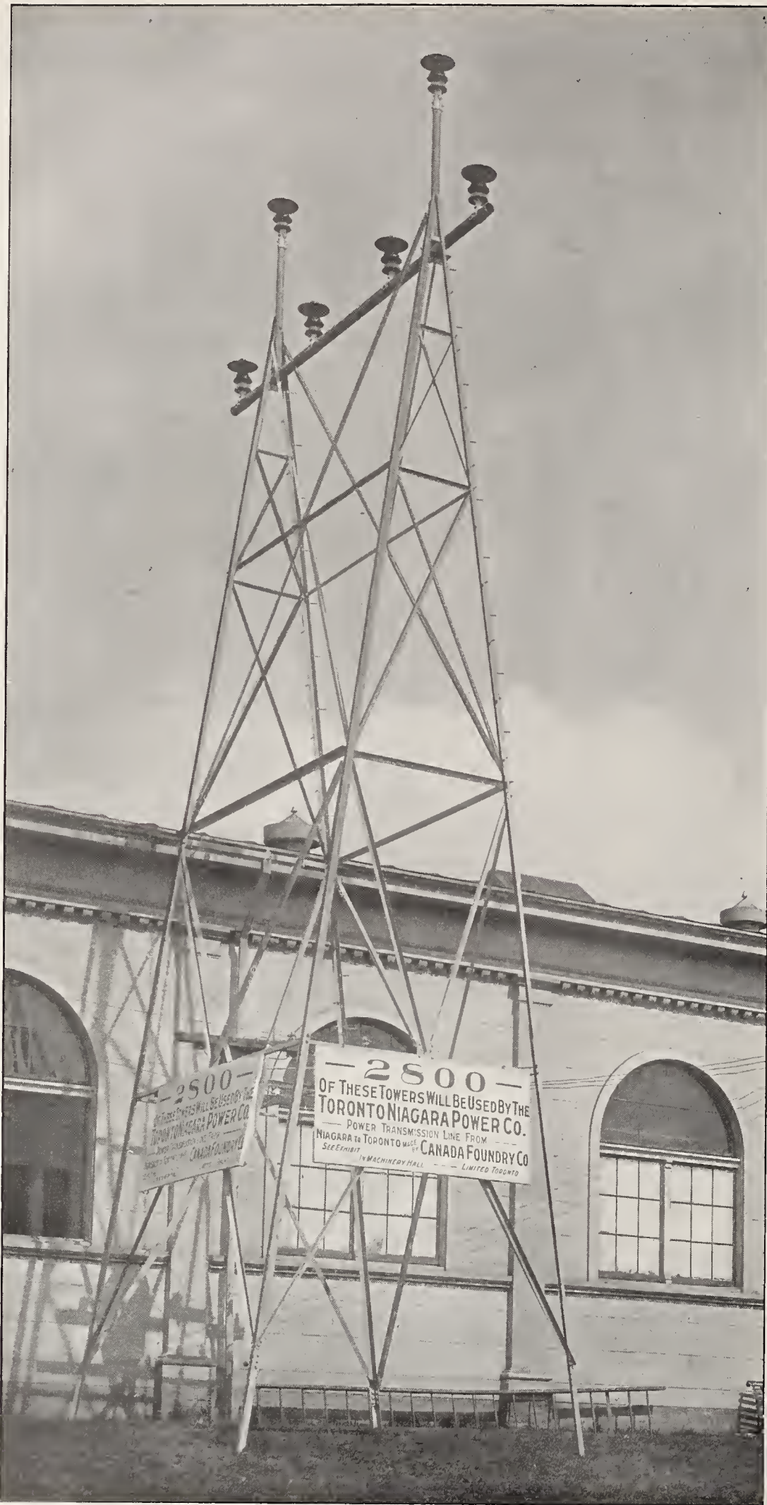
ONE OF THE STEEL TOWERS BUILT FOR THE TORONTO-NIAGARA POWER COMPANY BY THE CANADA FOUNDRY CO., LTD., TORONTO
