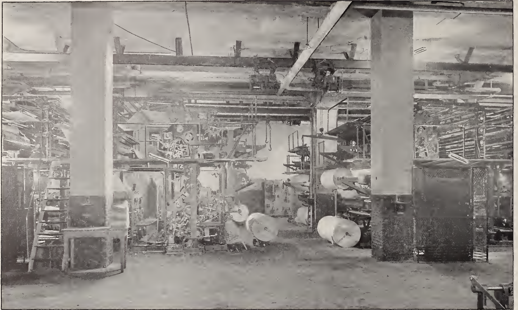
FIG. 21.—A VIEW OF THE NEW PRESS ROOM OF THE NEW YORK "TIMES." IN ADDITION TO THE MOTORS SUPPLIED BY THE MILWAUKEE ELECTRIC COMPANY, OF MILWAUKEE, WIS., DRIVING THE PRESSES, THERE ARE EIGHT SPRAGUE ELECTRIC HOISTS FOR HANDLING THE HEAVY ROLLS OF PAPER. TWO OF THESE HOISTS ARE TO BE SEEN HERE
