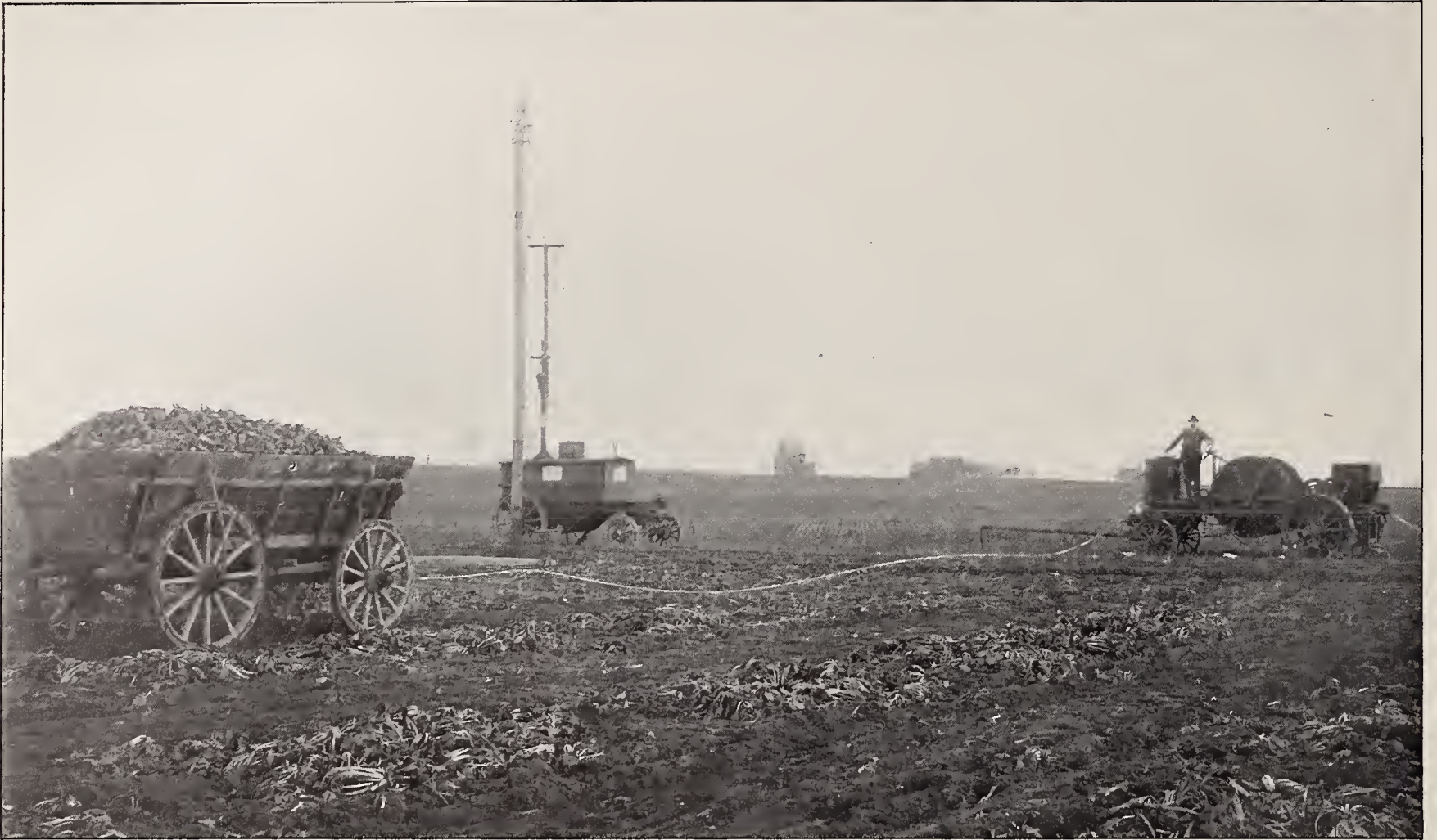
FIG. 3.—THE TRANSFORMER WAGON IS HERE SHOWN IN ITS OPERATING POSITION, NEAR THE POLE CARRYING THE ELECTRIC TRANSMISSION LINE AND CONNECTED, FROM ITS OWN MAST, WITH THAT LINE
