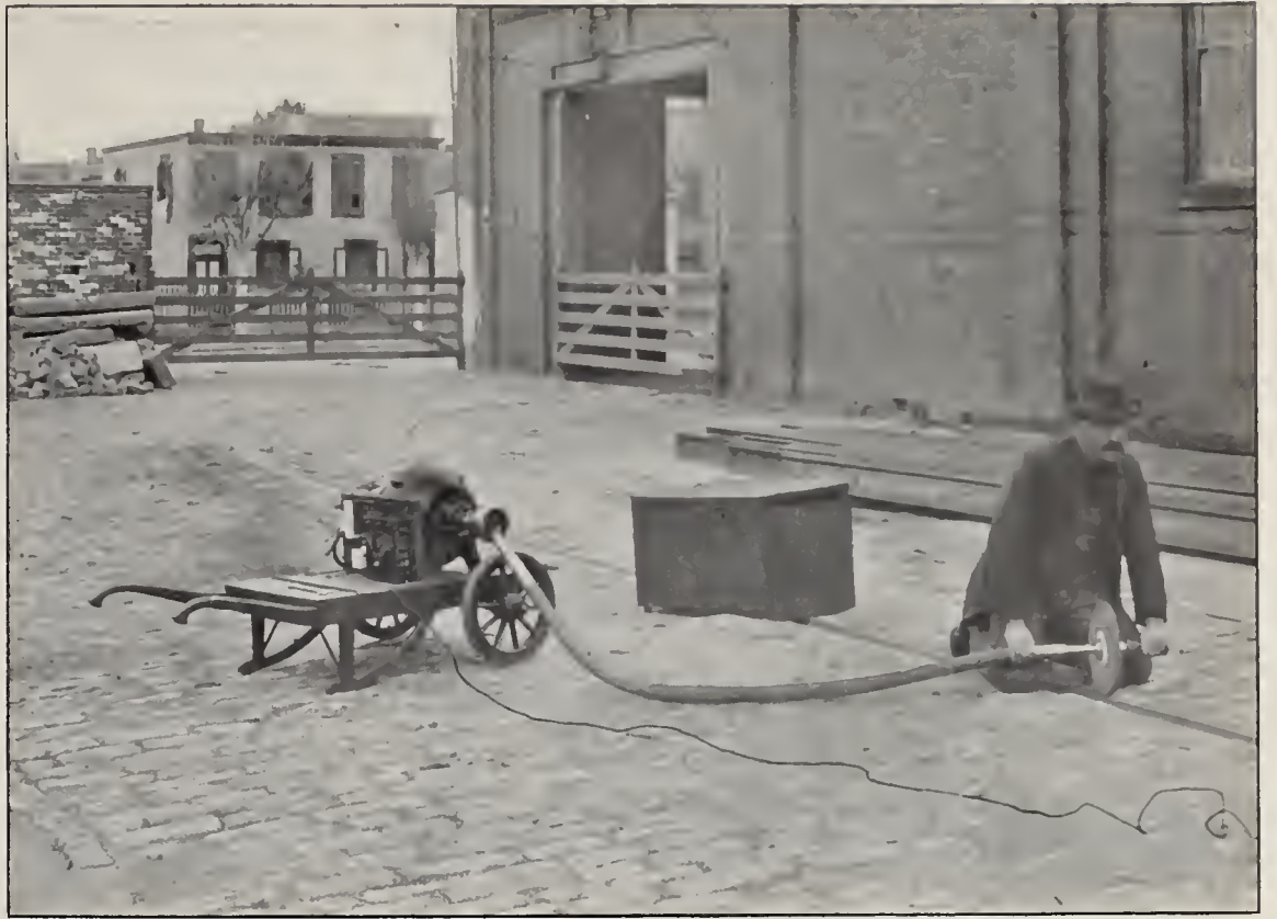
GRINDING WELDED RAIL JOINTS WITH A PORTABLE MOTOR OUTFIT
