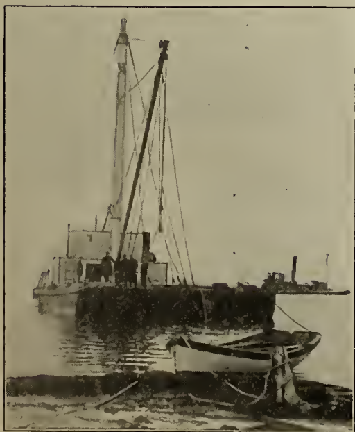
Landing the Shore End of the Cable at Fire Island.
