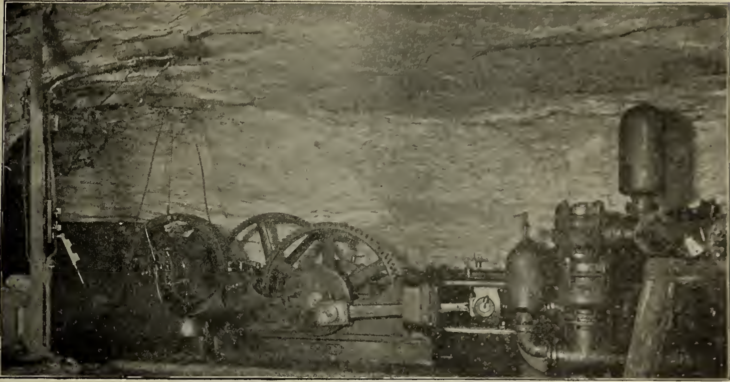
10-in. x 18-in. Pump and 85 H.-P. Motor.
