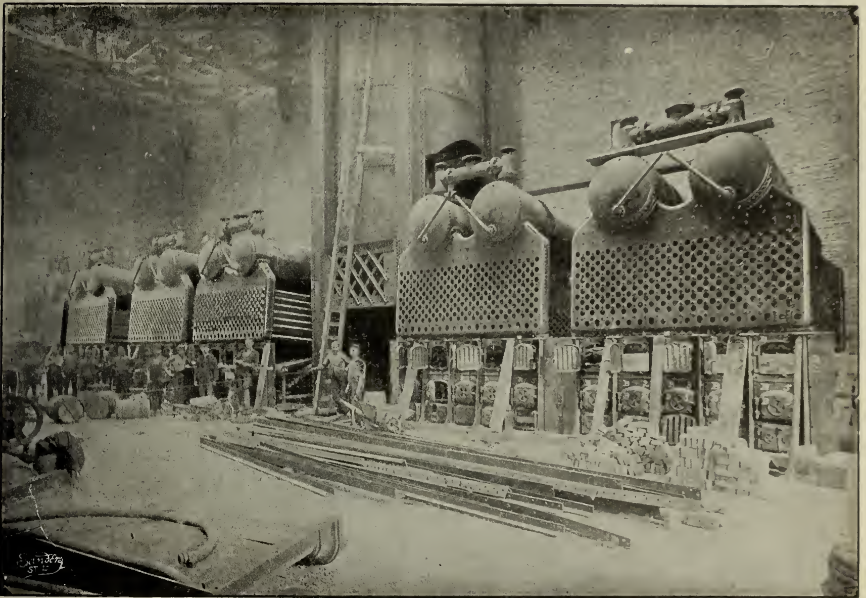
The Edison Company's Electric Light Plant. Installing the Down-Draft Furnace.
