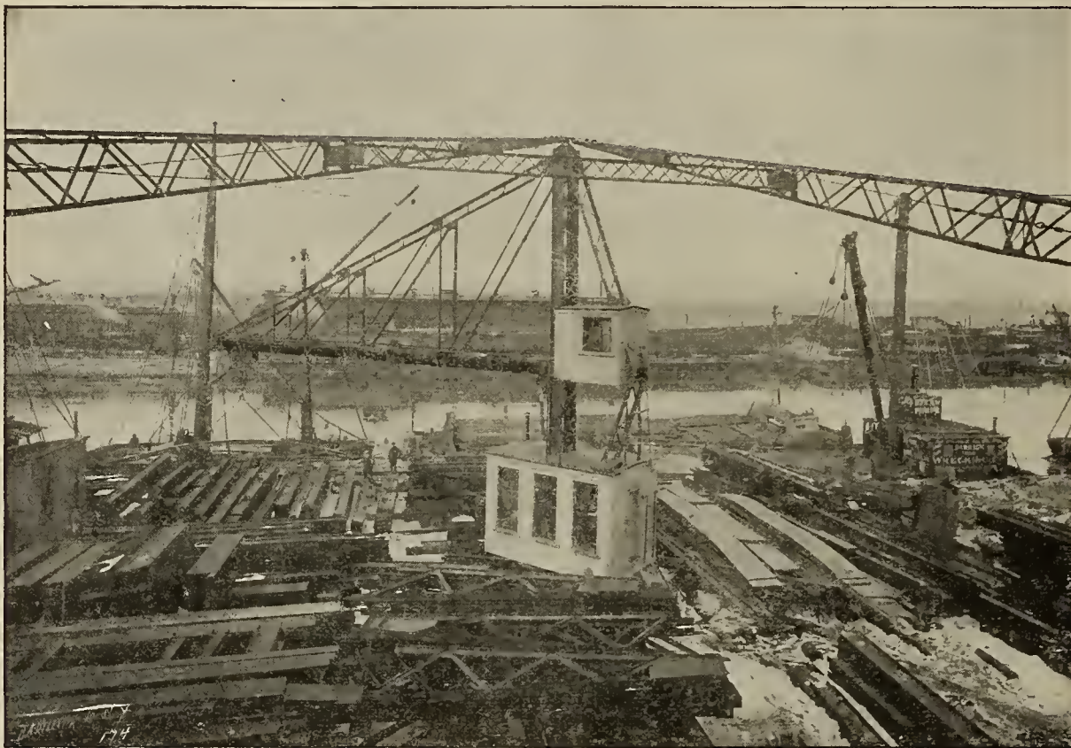
10-Ton Derrick Crane at Iron Works of Messrs. Post & McCord, Brooklyn, N. Y. One size 10 C.-W. Single-Reduction Motor on Hoist and one size 3 C.-W. Motor on Trolley Travel.
