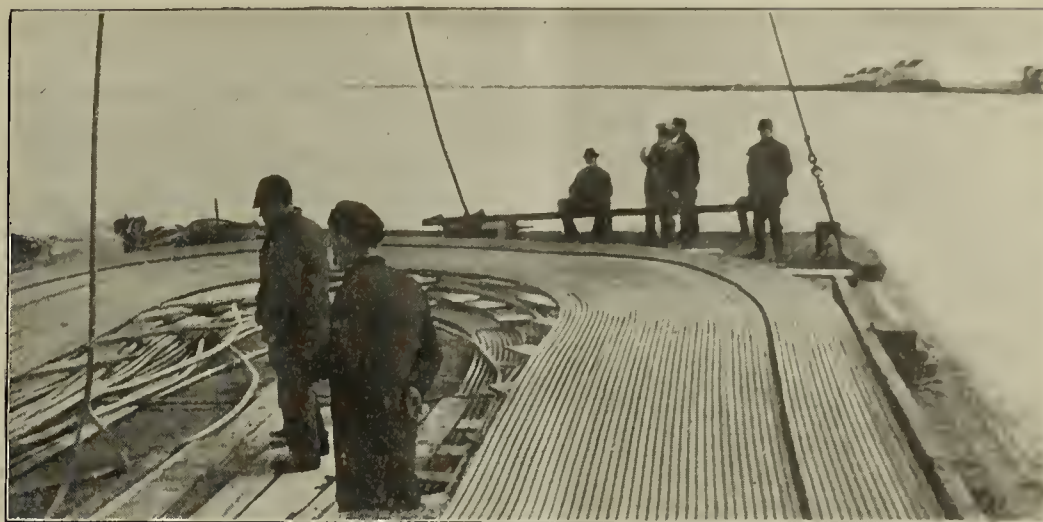
Paying Out the Cable Across Great South Bay.
